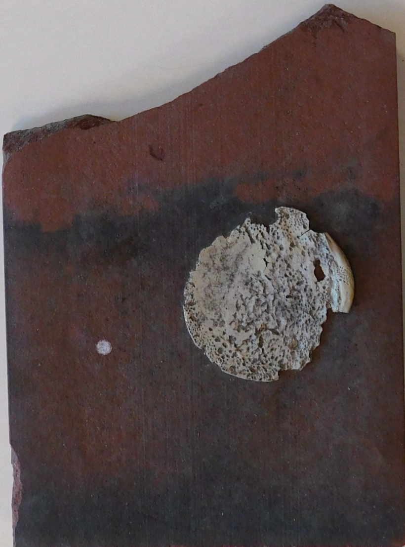
EXISTING ROOF TILE
