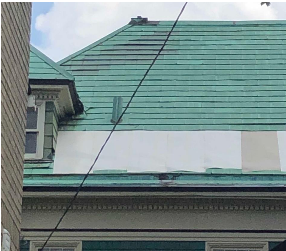
Rear elevation of house, with standard dormer. Largest area of missing roofing.
