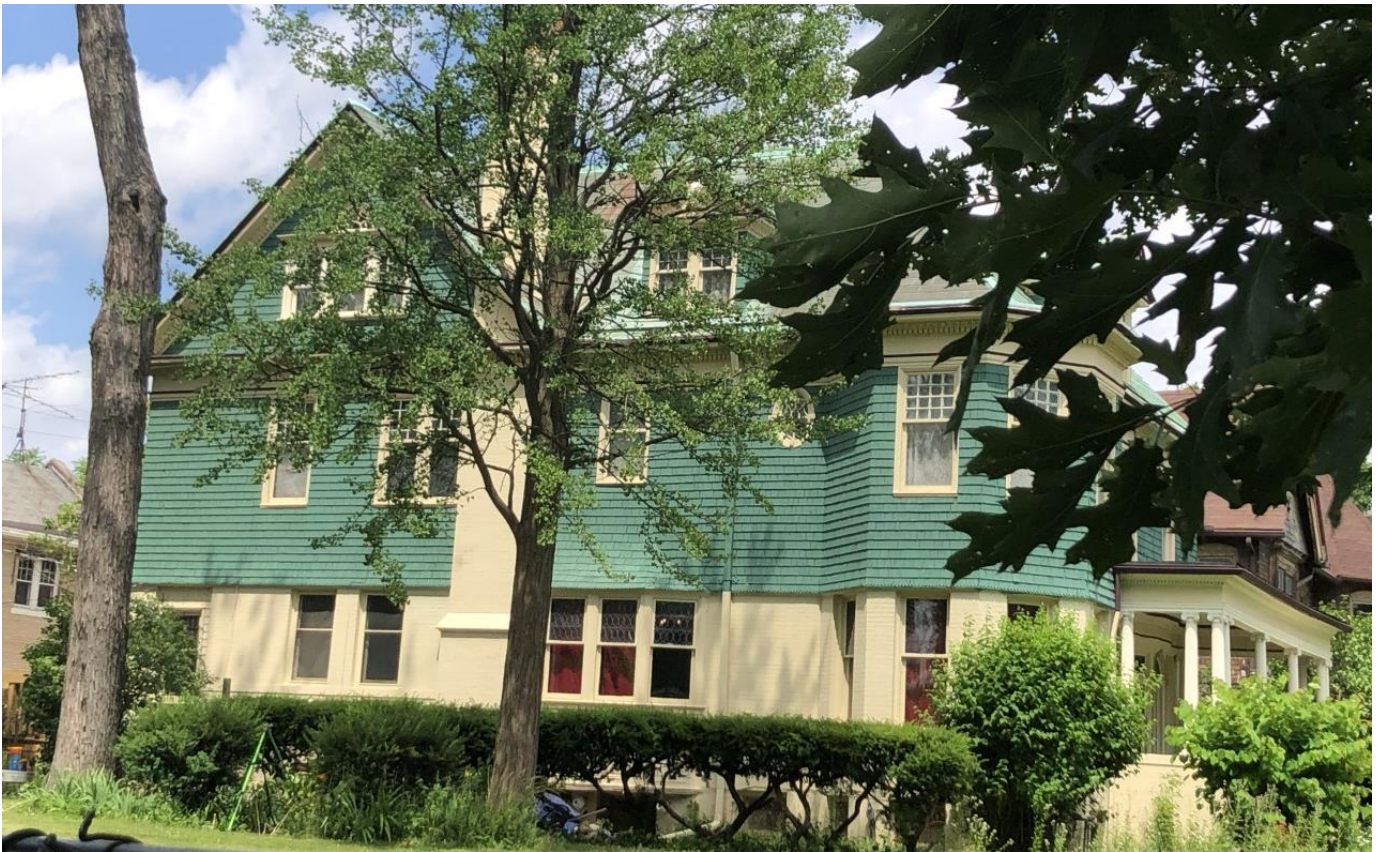
West elevation facing John R
