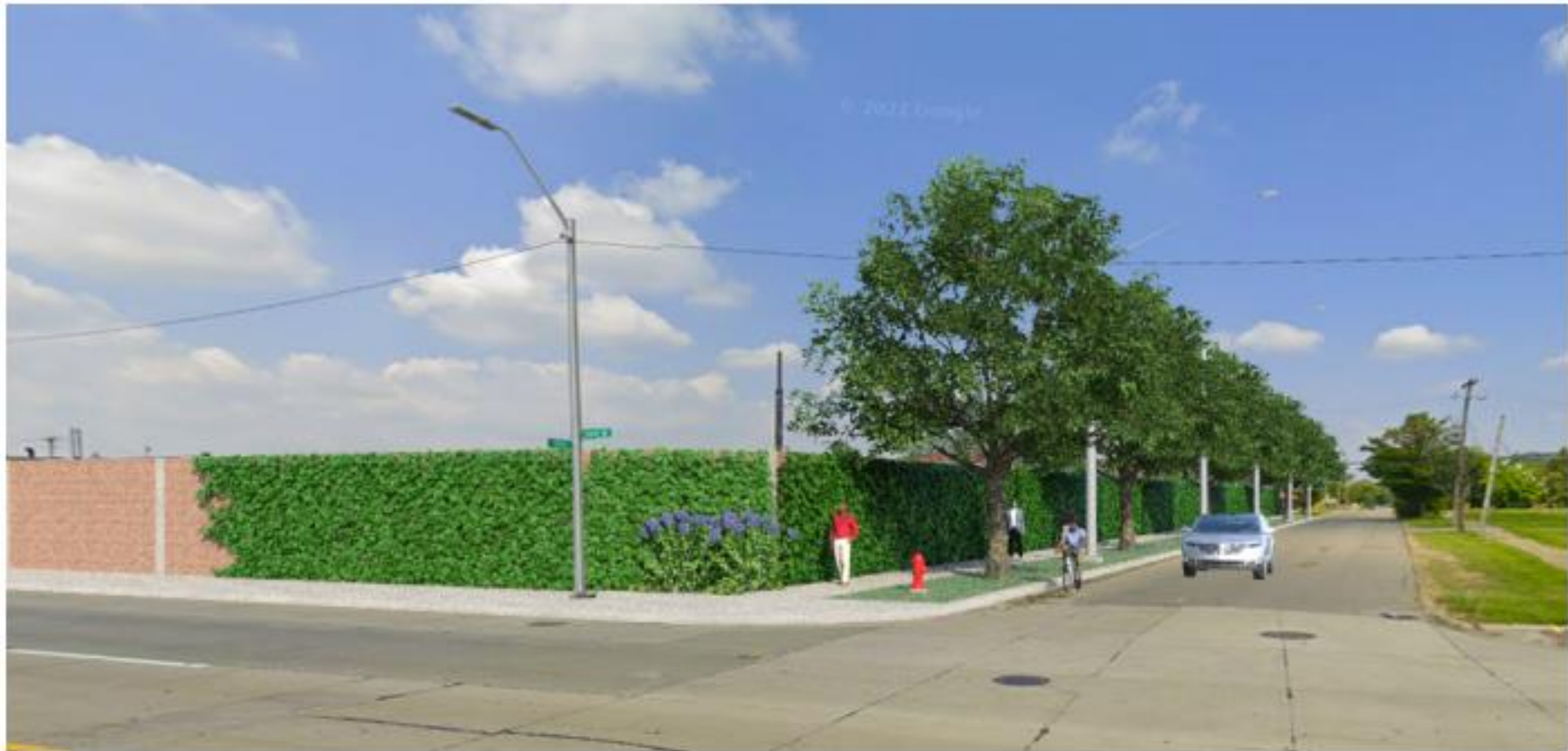
VIEW LOOKING NORTH AT THE CORNER OF 18TH STREET AND FORT STREET
