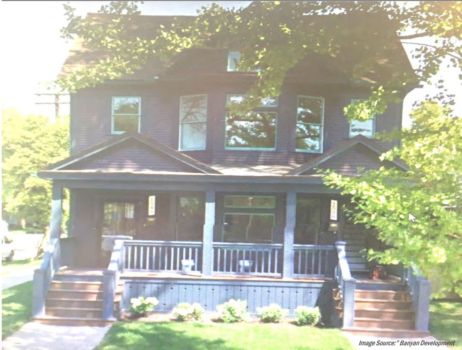
Van Dyke Rehab AFTER
