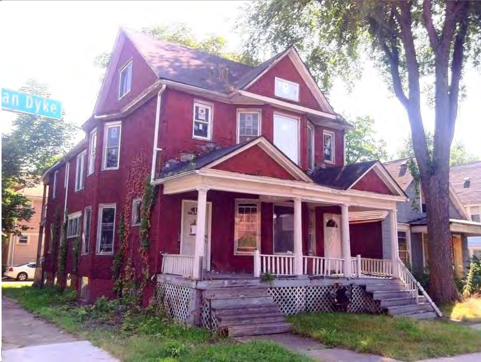
Van Dyke Rehab BEFORE
