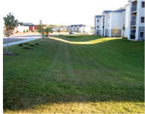
Traditional Dry Detention Basin
