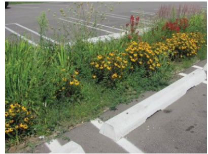
Bioretention between Parking Lot Aisles
