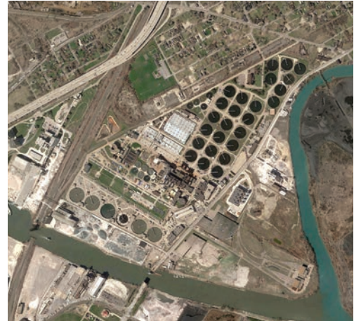
Detroit's Wastewater Treatment Plant
