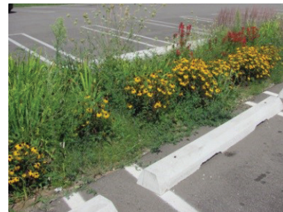
Bioretention between Parking Lot Aisles
