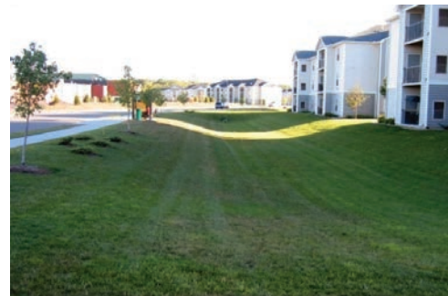
Dry Detention Basin
