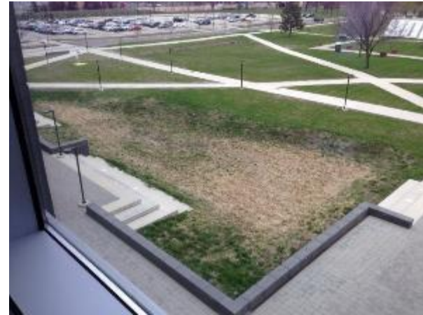
WCCC dry detention pond
