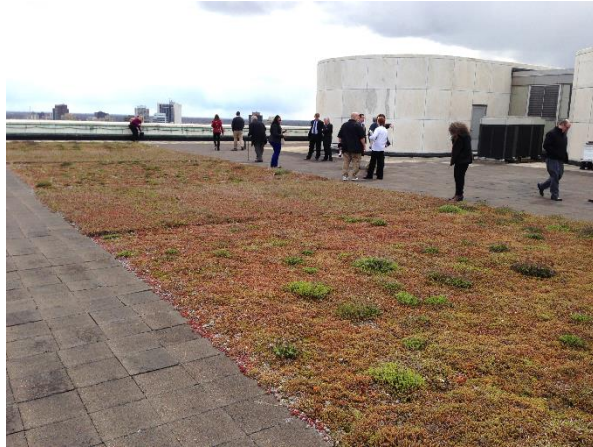
CAYMC Green Roof
