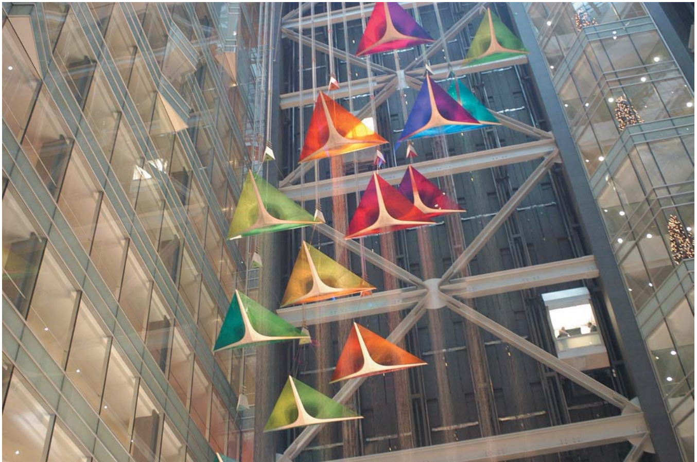
The view inside the Compuware World Headquarters atrium lobby is striking.
