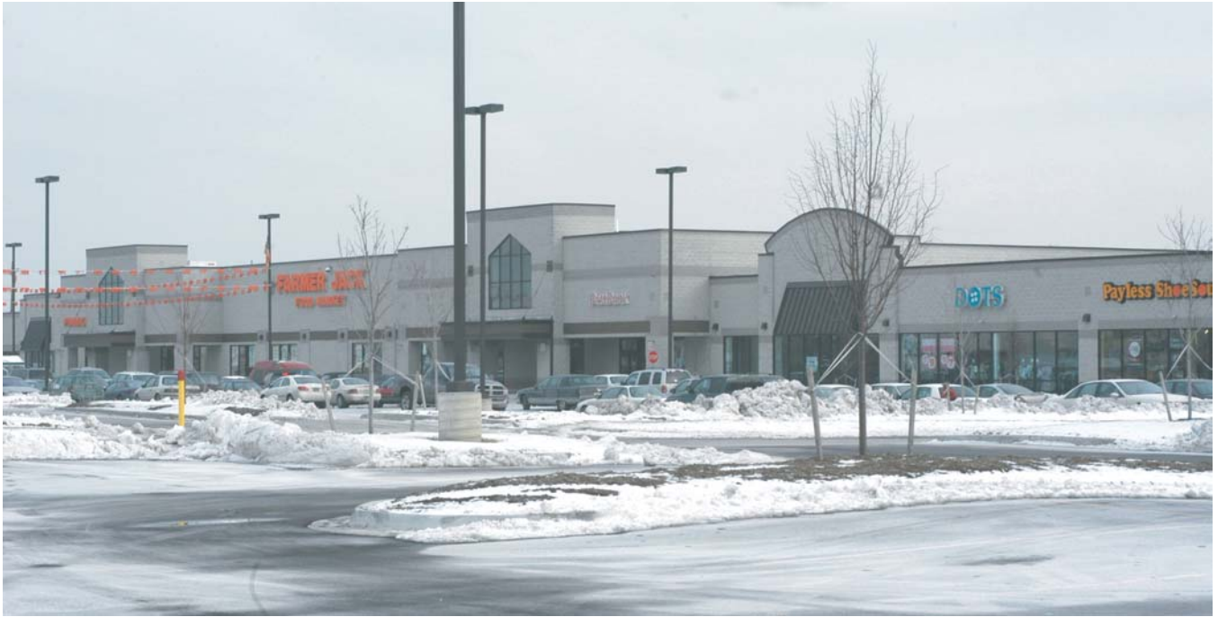
The largest Farmer Jack store in Michigan - at 64,000 square feet - is in Detroit on East Jefferson. The full-service supermarket, which opened in 2003, is an asset for appreciative east side residents.
