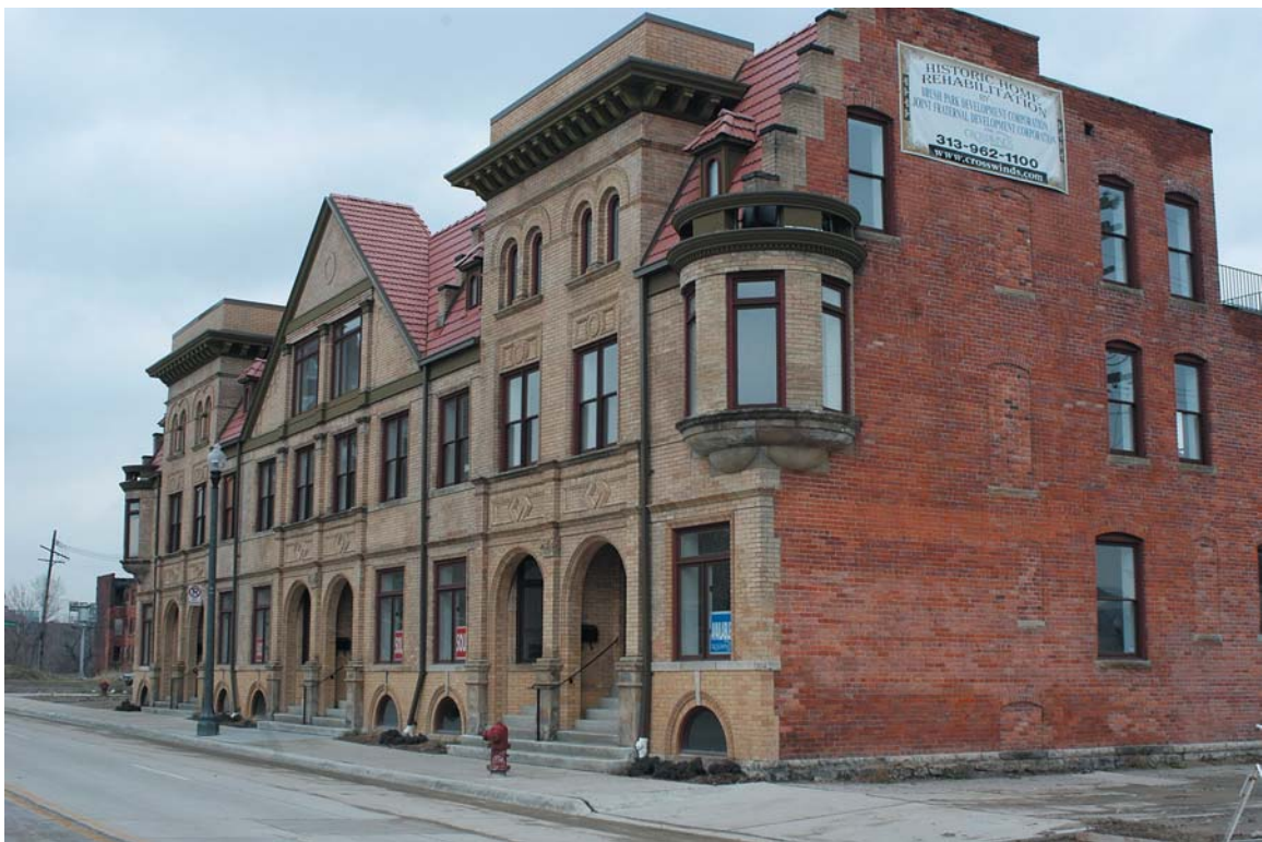
The Brownstones on John R are part of Crosswinds Communities' Woodward Place project in Brush Park, just north of downtown. Six renovated luxury townhouse units, beginning in the $400,000s, offer modern urban living in a historic 1890s rowhouse building.
