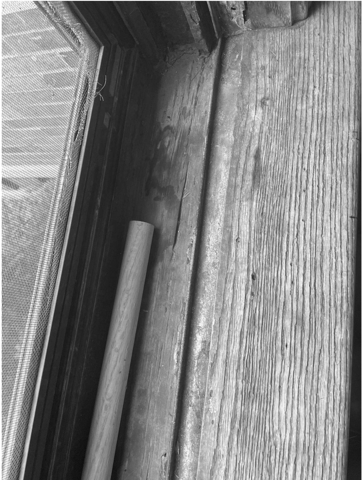
Window #1 - Waterdamage
