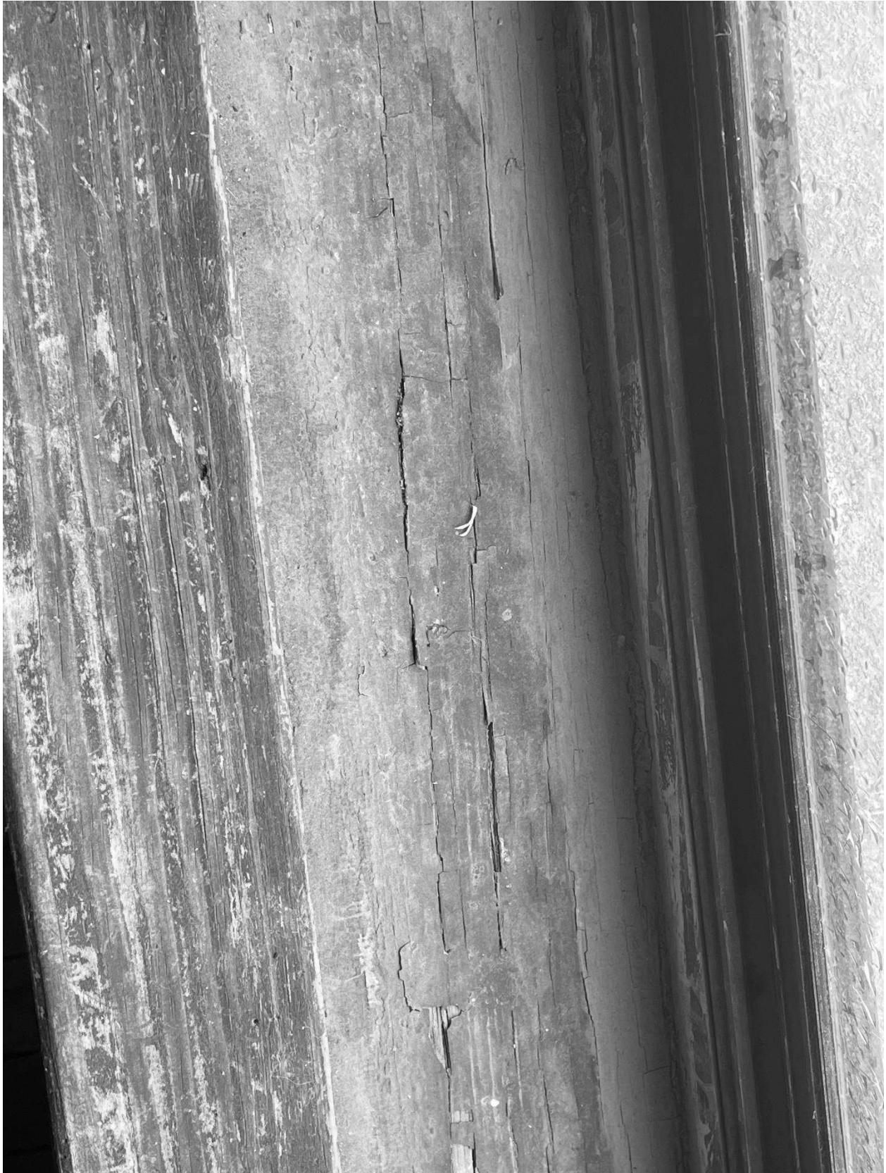
Window #11 – Water Damage
