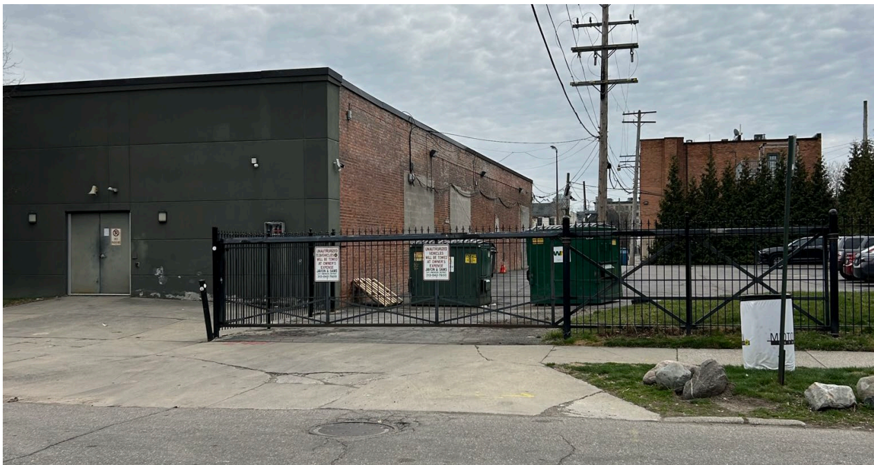
Looking south to adjacent commercial building, sliding gate and trash dumpsters
