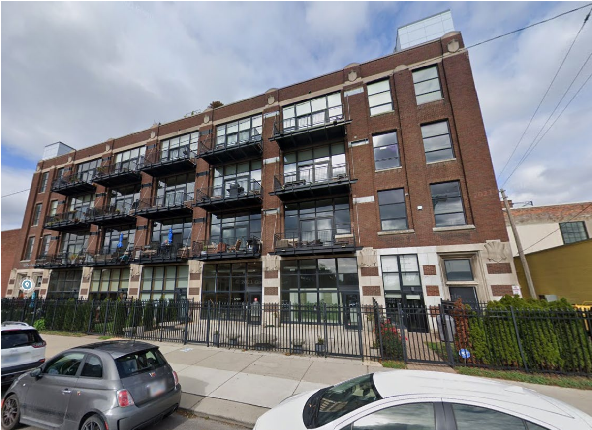
Looking north at the Willys-Overland Residential Lofts
