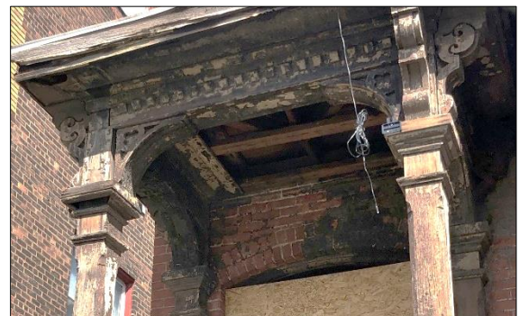
Intact 19 th century porch at 3644 Lincoln. Nearby property referenced by applicant. Staff photo.
