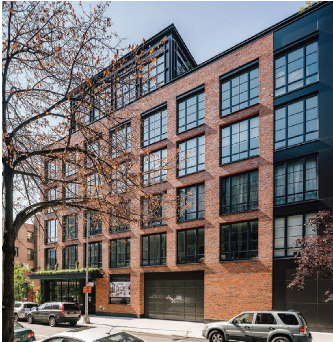
RED BRICK & CORNICE
