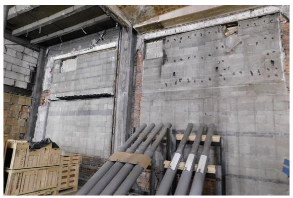
Figure 57: Interior, Looking West, CMU Infill Where Alley Storefronts used to be located. 2/27/20
