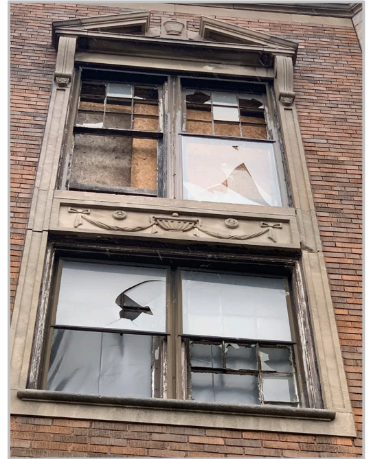
Photo 2: Mulled Double-Hung Windows on the Front Facade
