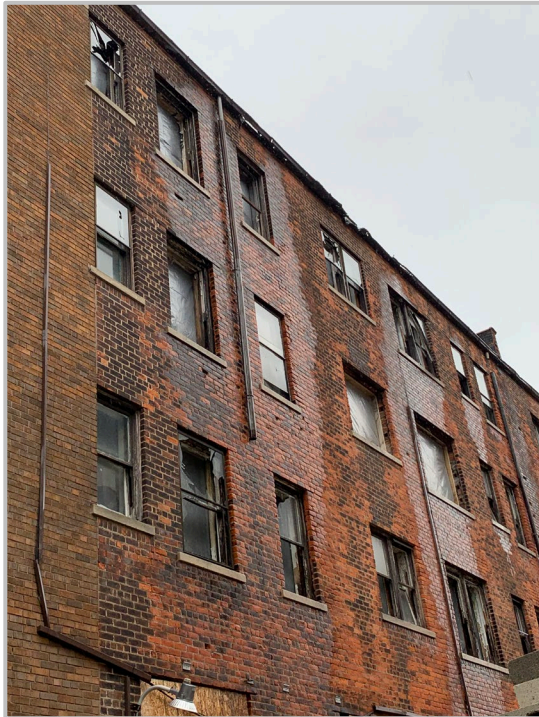
Photo 1: View of Windows on the West Elevation
