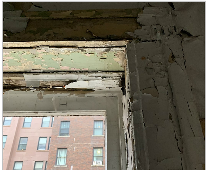
Photo 4: Interior view of the Top Rail, Side Rail and Interior Casing
