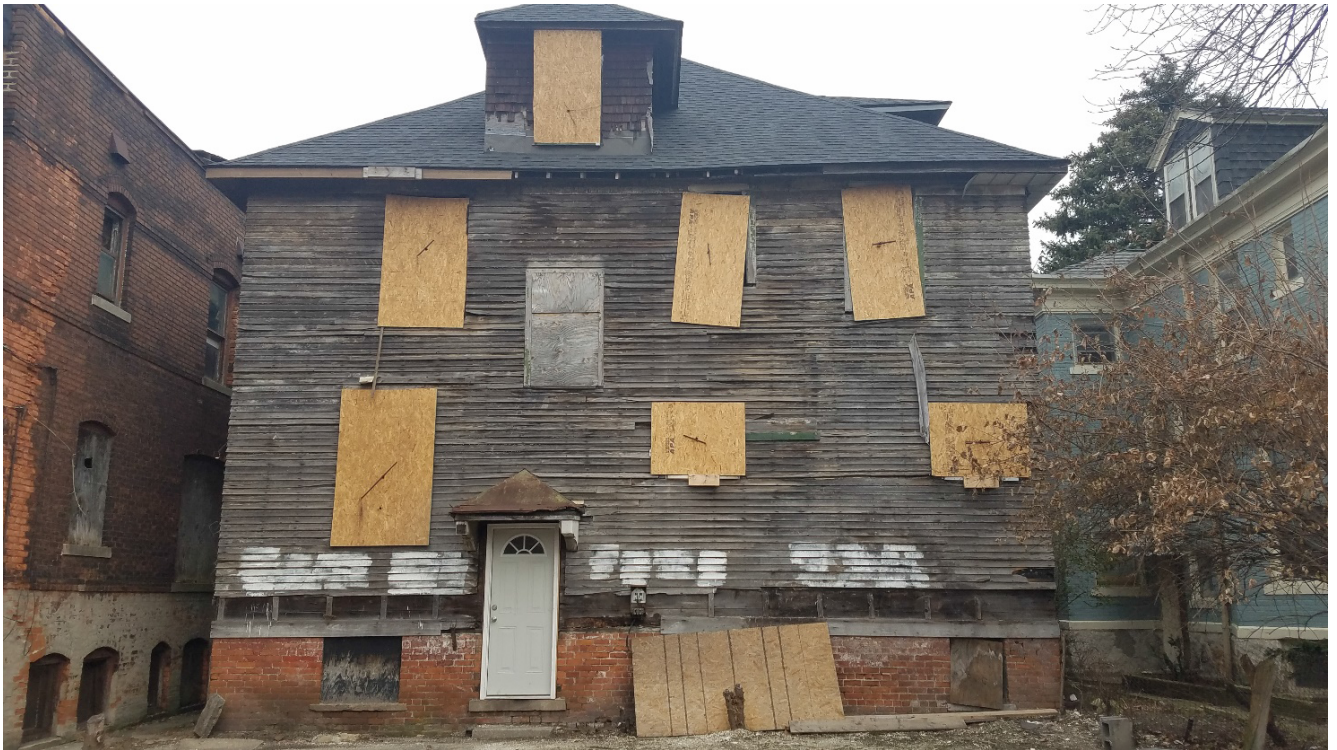
Rear façade, Applicant Photo
