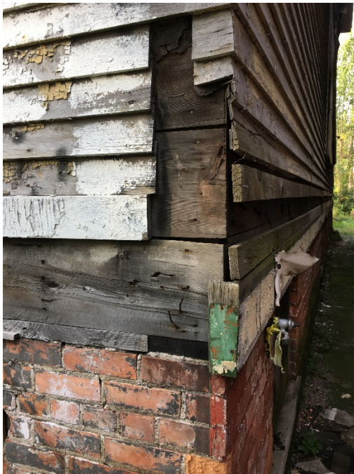
Typical Wood Siding and Sheathing Condition
