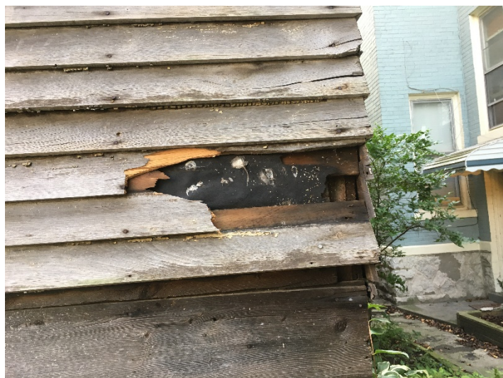
Typical Wood Siding and Sheathing Condition
