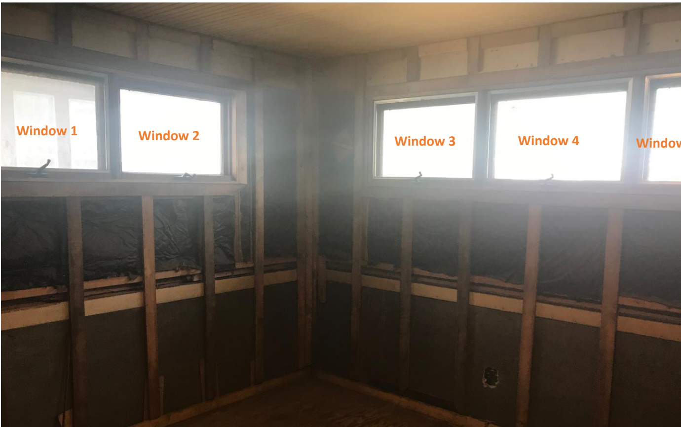
Interior West and North Walls
