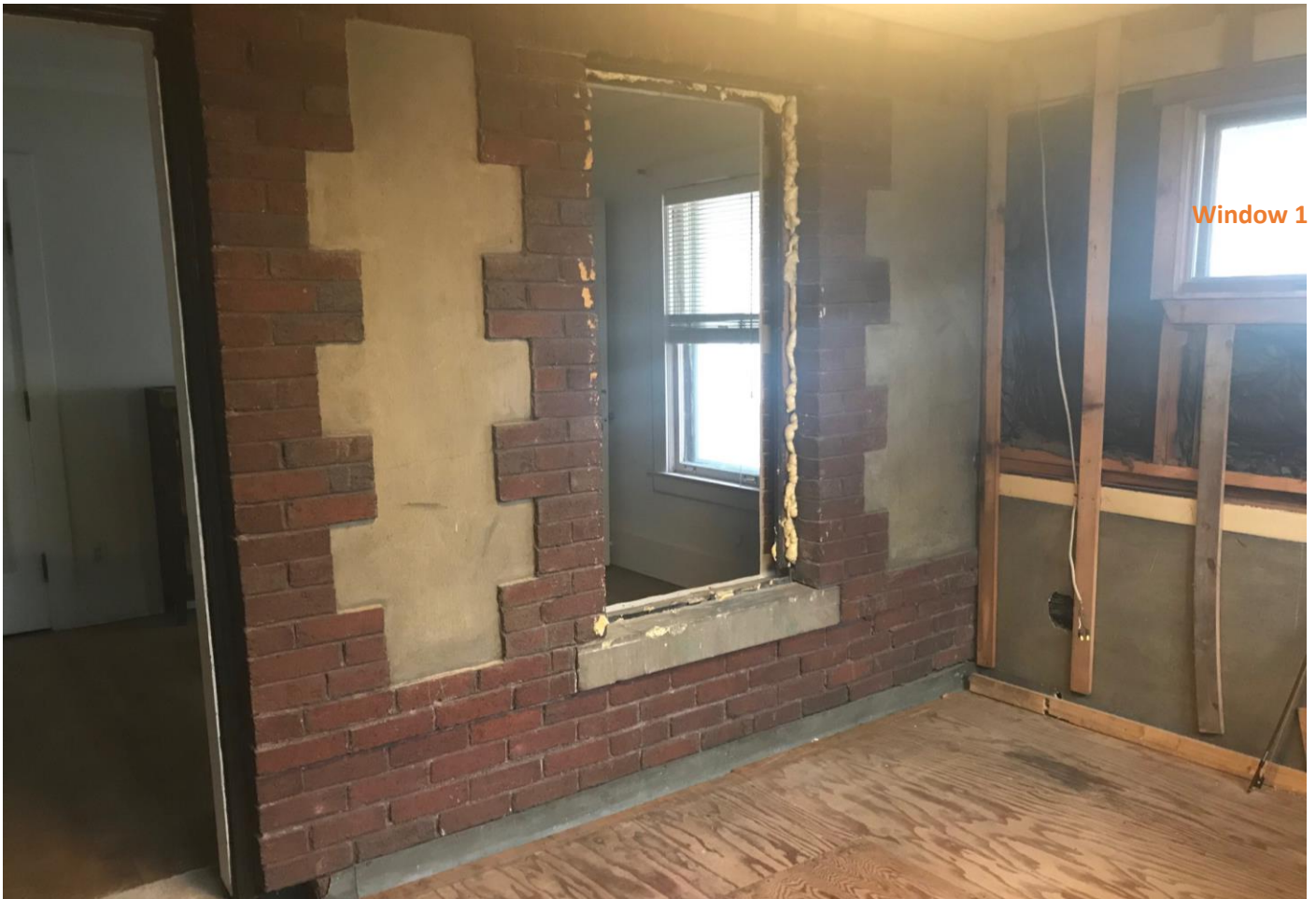
Original Rear Exterior Window Opening - South Wall Interior
