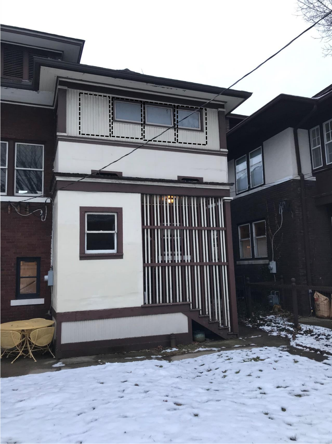
Photo 2. North face of exterior (photo taken facing south)
