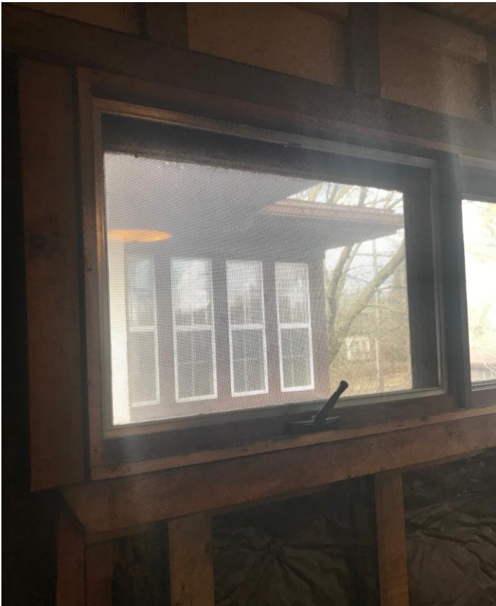
Window 1 – West Wall Interior
