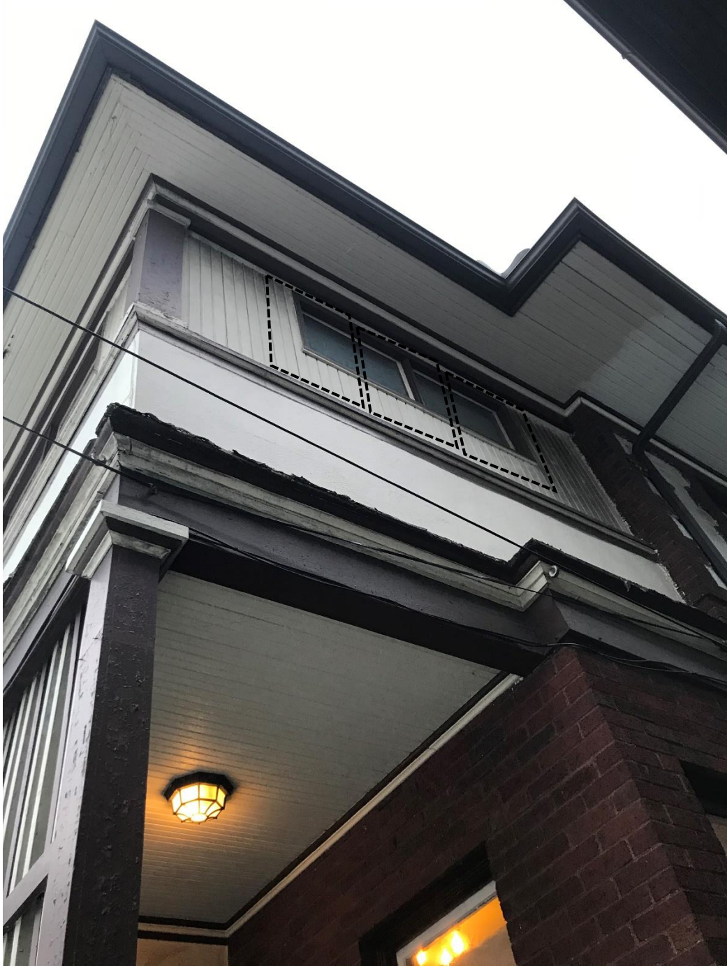
Photo 3. West face of the exterior (photo taken facing east)
