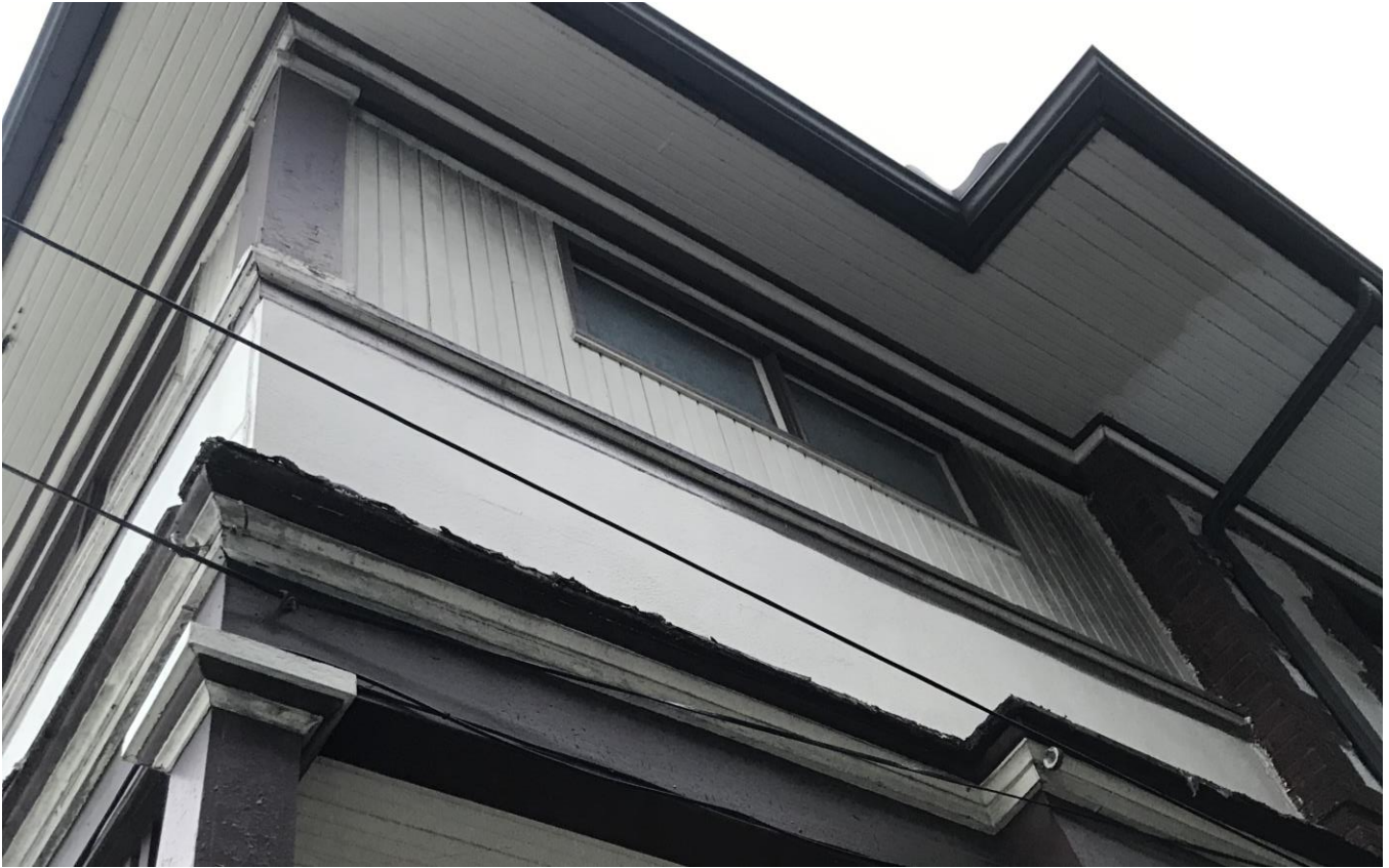
Exterior View of Windows 1 & 2 - West Wall Exterior (photo facing east-southeast)
