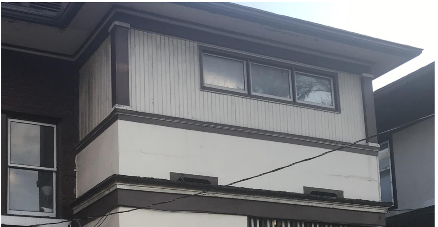
Exterior View of Windows 3, 4, & 5 - North Wall Exterior (photo facing south-southwest)
