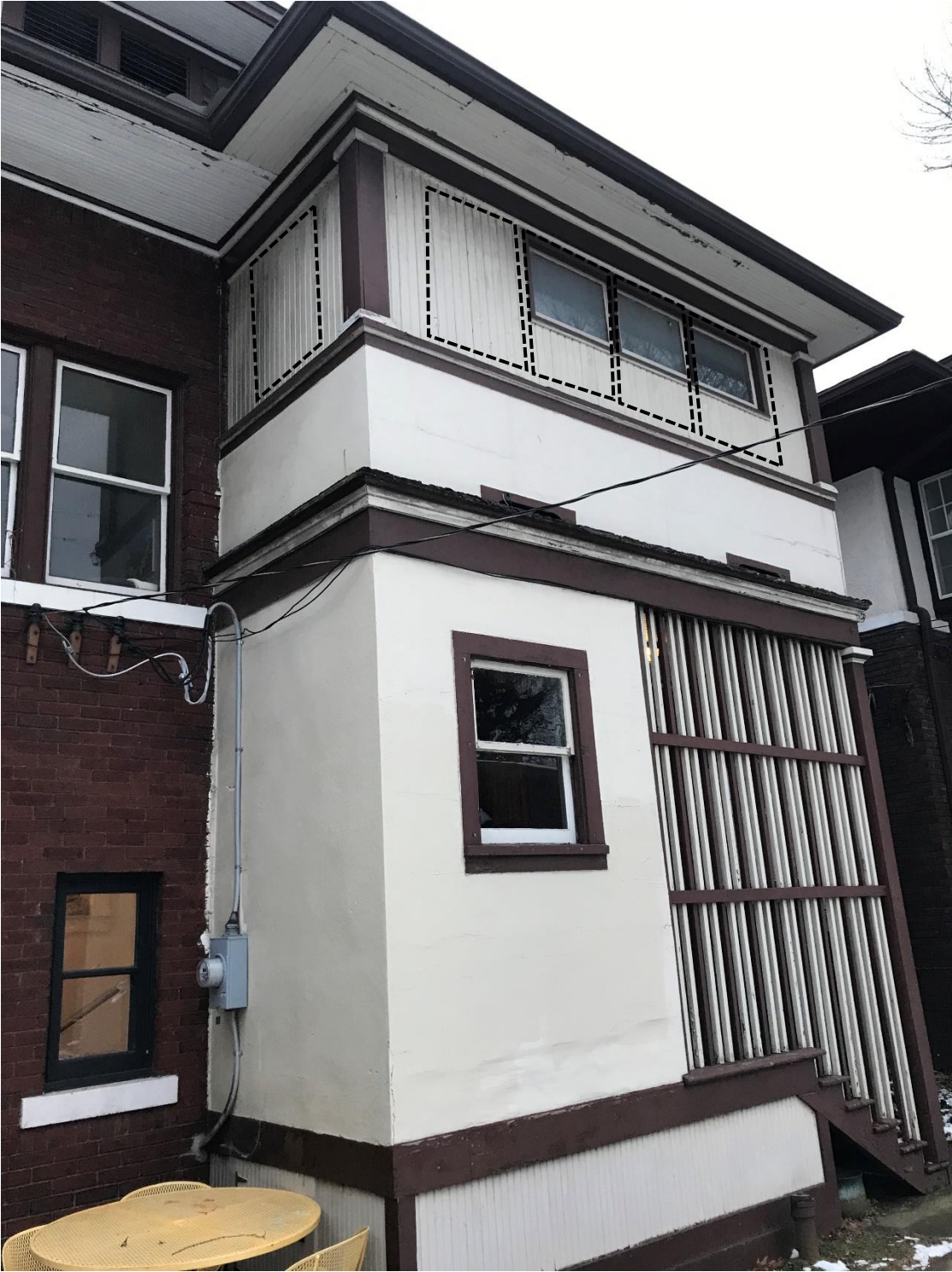
Photo 1. East and North faces of the exterior (photo taken facing southwest)
