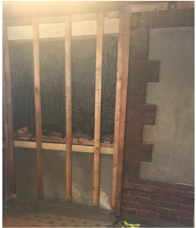
No Existing Window - East Wall Interior
