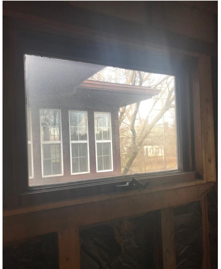
Window 2 – West Wall Interior
