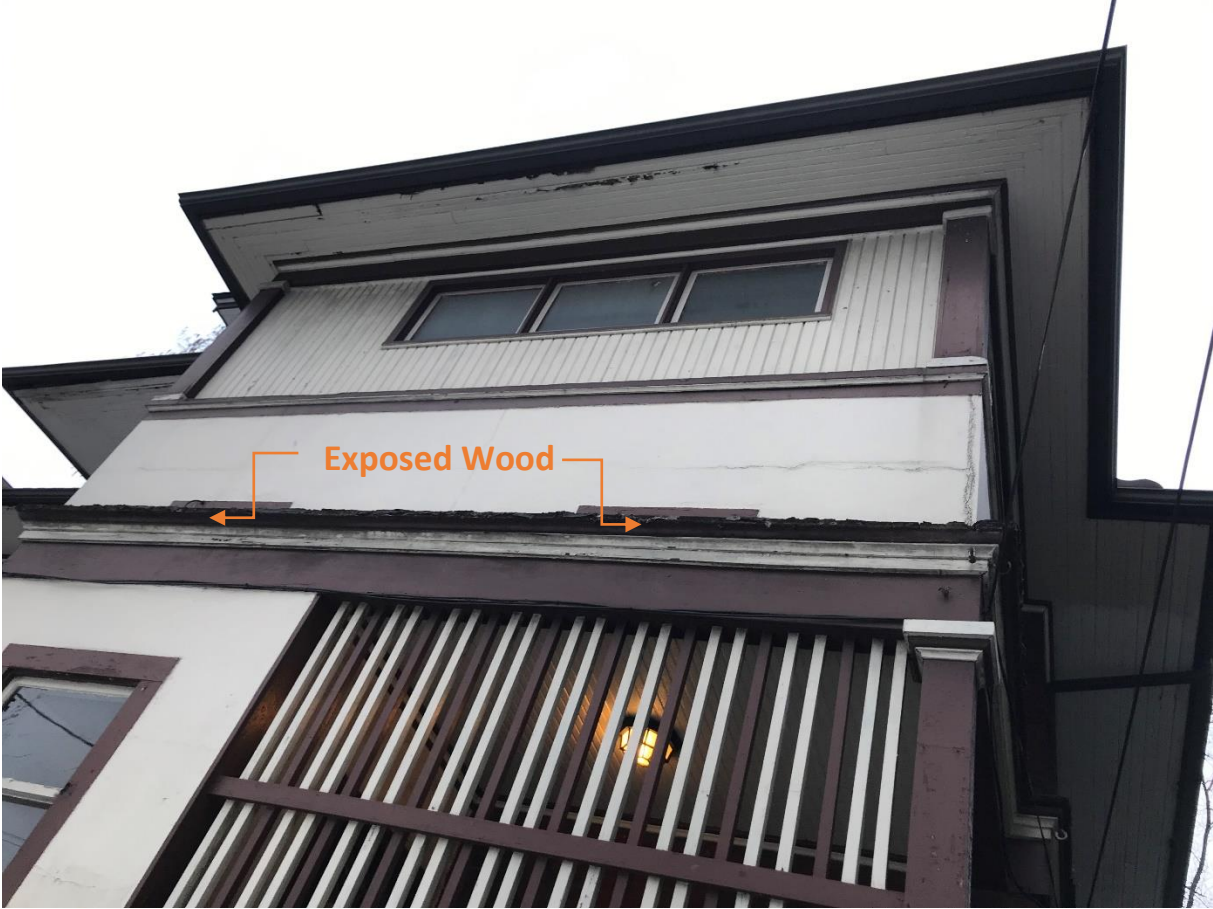
Photo 4. North face of the exterior highlighting exposed wood edge (photo taken facing south)
