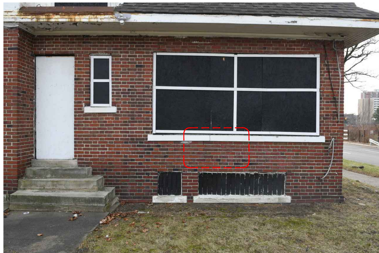
04 NORTH FACADE - BELOW WINDOW 106
