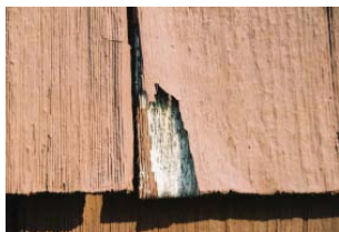
Not back primed. Primed over weathered wood .
