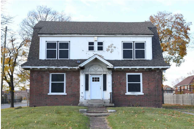
Front of home, Applicant Photo (South Elevation)
