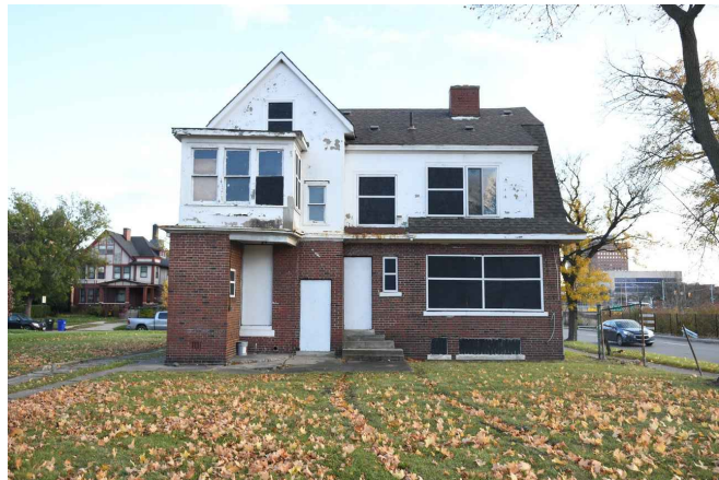
Rear of home, Applicant Photo (North Elevation)
