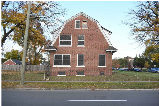
Side of home, Lodge Service Dr., Applicant Photo (West Elevation)
