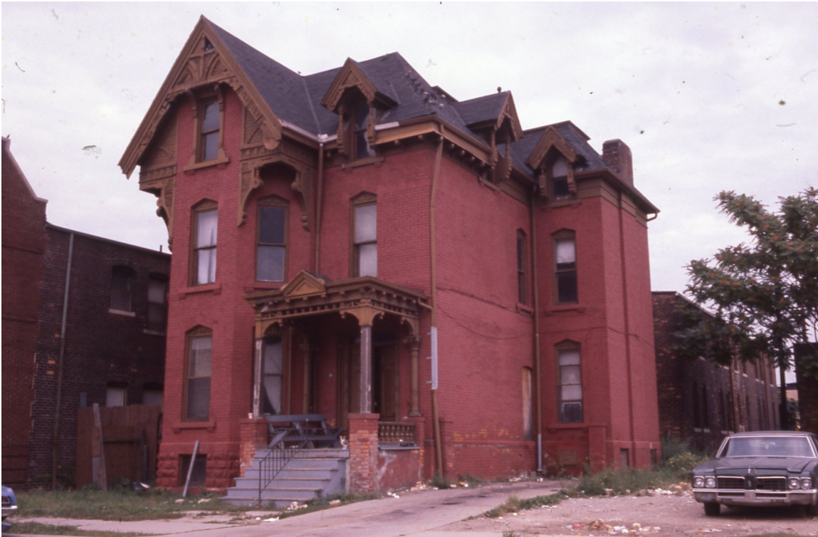
HDAB Designation Photo of 291 Winder, 1980. The original nineteenth century three-story mansion featured red brick and a spectacularly intricate and ornamented roof line and porch. Note the early twentieth century apartment block addition extending to the rear, a typical addition in Brush Park to accommodate more residents in the twentieth century.
