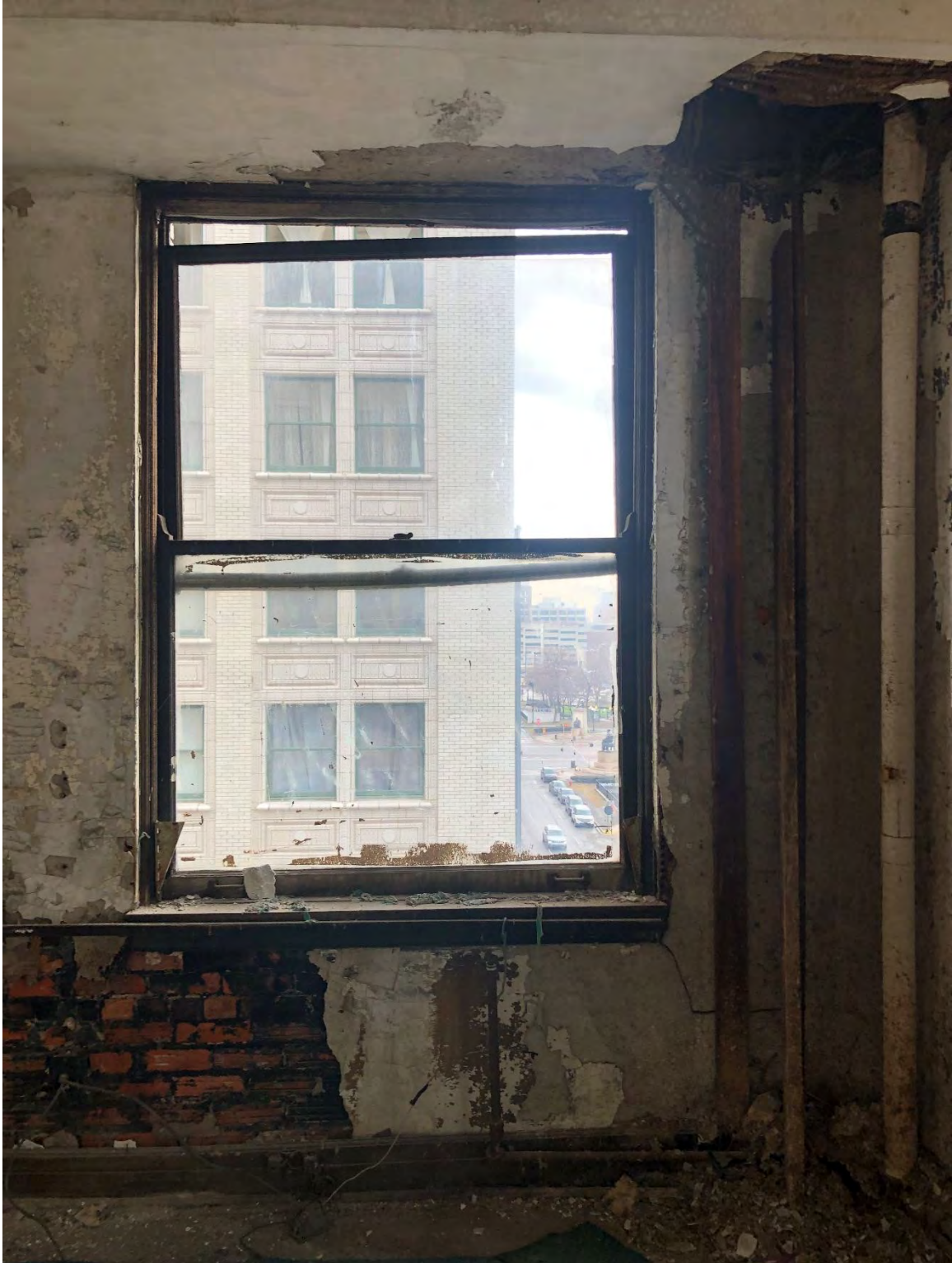
Figure #38: Interior, 6 th floor, Window, Looking East. 2/4/19
