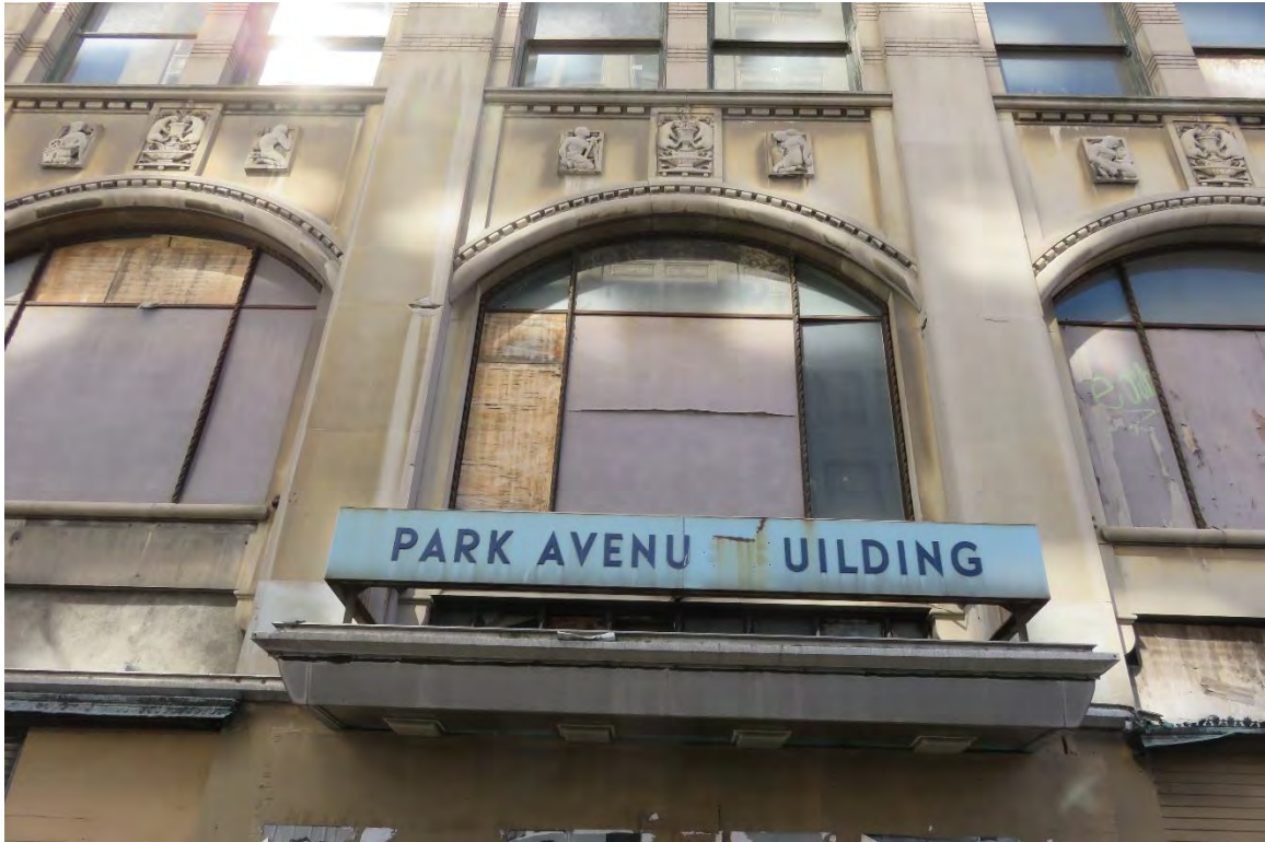
Figure #15: Exterior, window detail, looking west. 9/11/2018
