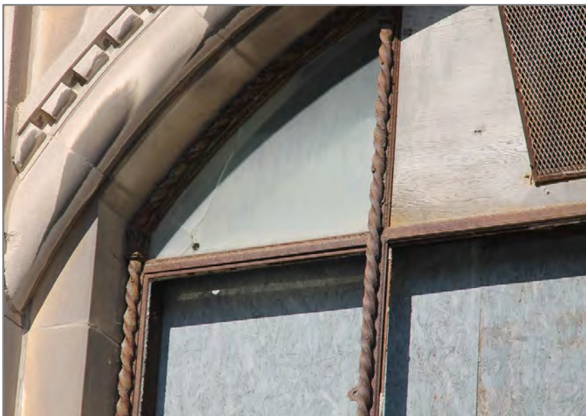
Exterior View of Large Radius Window with Decorative Rope Detail
