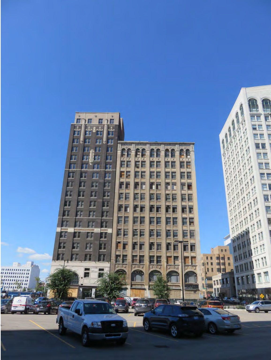
Figure #1: Exterior, South Façade, Looking north. 9/11/2018
