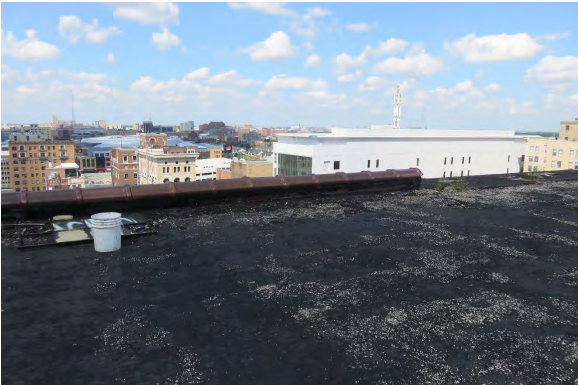
Figure #49: Exterior, roof, looking north. 9/5/2018
