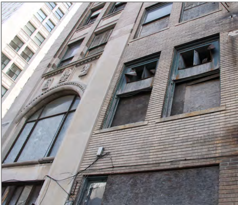
Exterior View of Wood Double-Hung Windows
