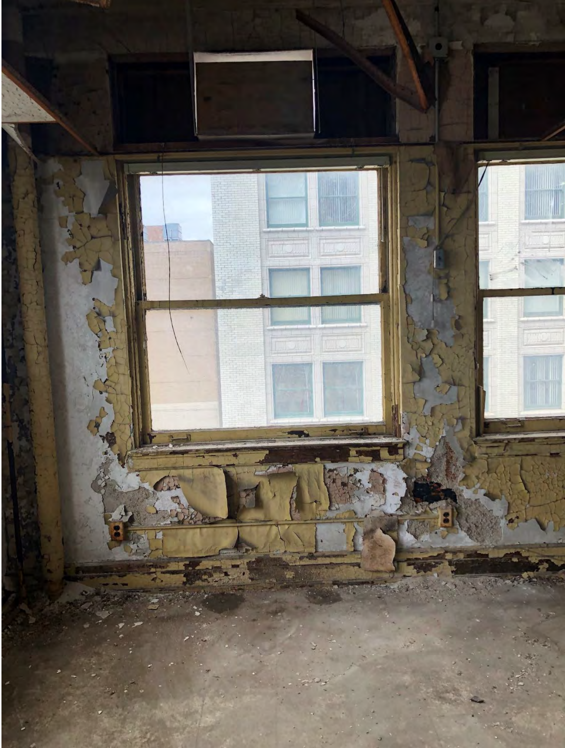
Figure #36: Interior, 8 th Floor, Window Detail. 2/4/2019
