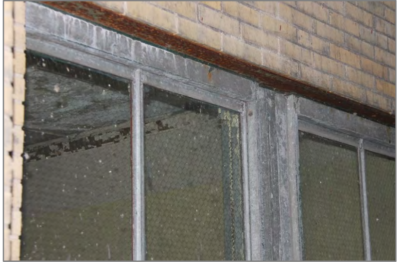
Interior View Steel Double-Hung: Head and Mullion
