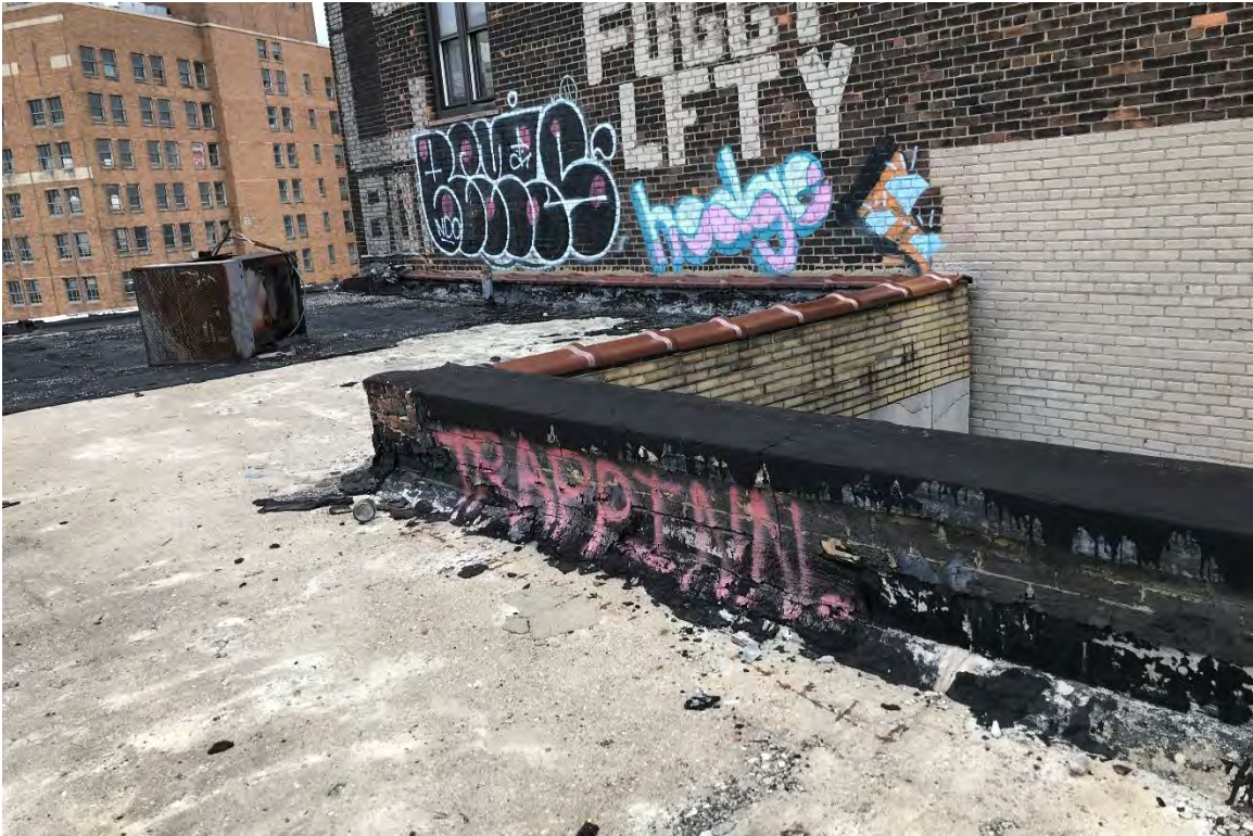
Figure #45: Exterior, parapet next to lightwell, looking southwest. 9/5/2018
