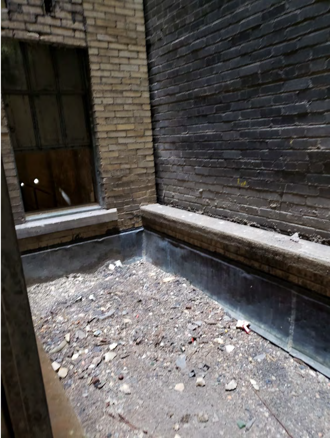
Figure #27: Exterior, Bottom of Lightwell, Looking Southwest. 7/15/19
