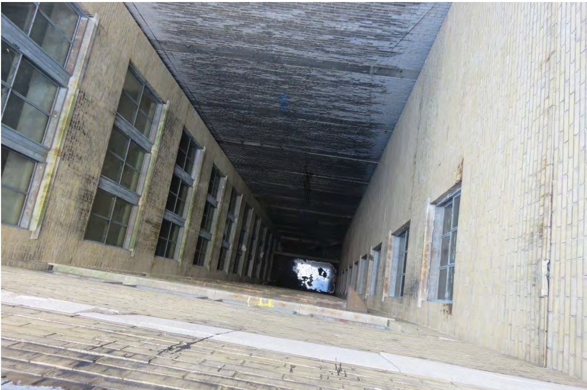
Figure #46: Exterior, lightwell, looking down. 9/5/2018
