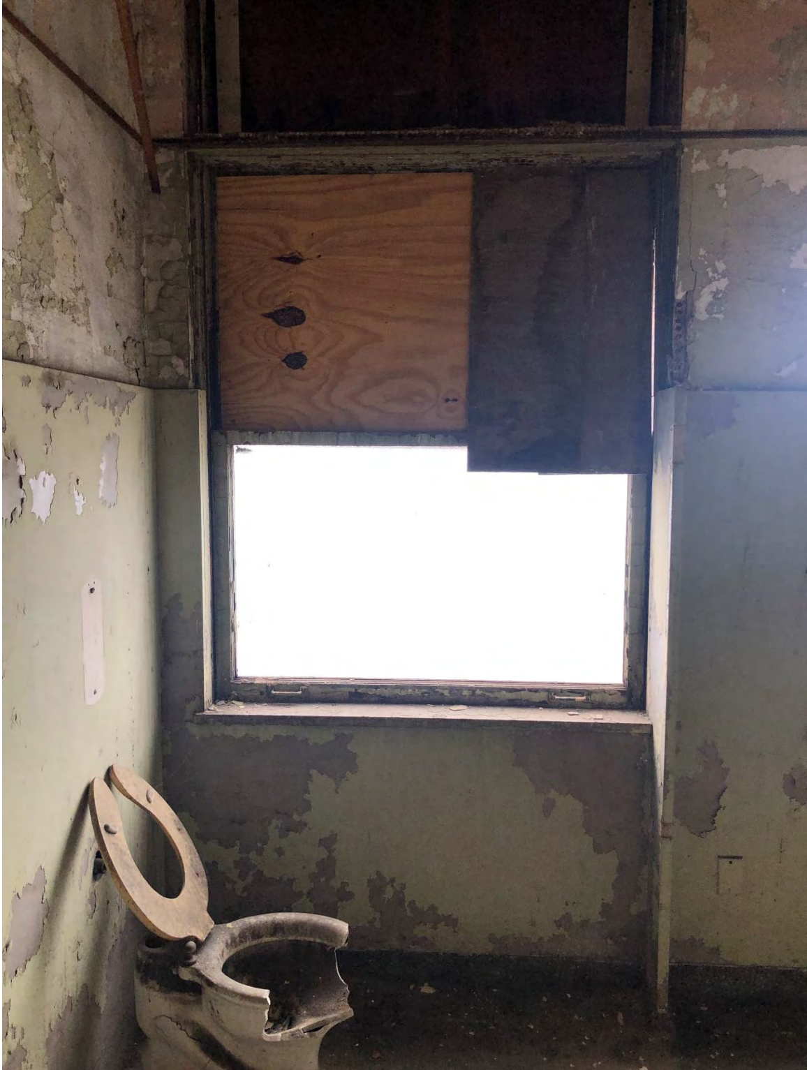
Figure #37: Interior, 8 th Floor, Window, Looking North. 2/4/19
