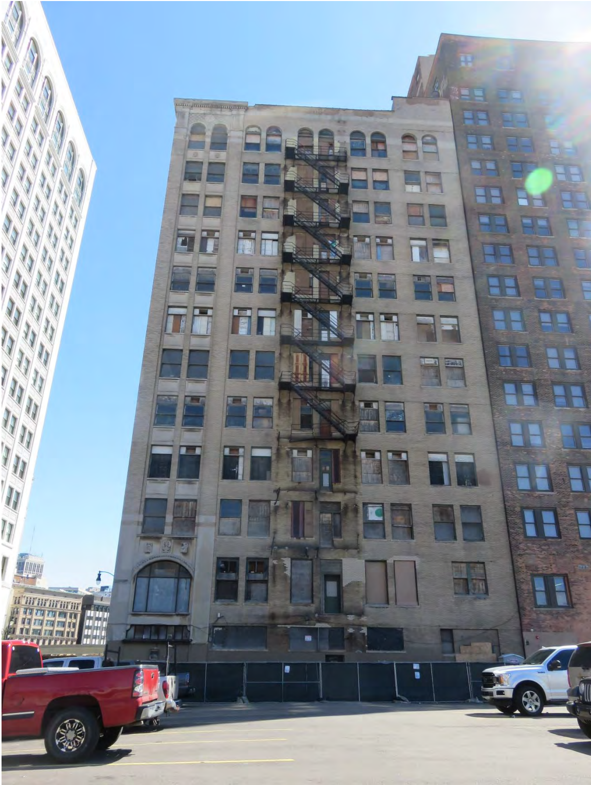
Figure #3: Exterior, North Façade, Looking south. 9/11/2018
