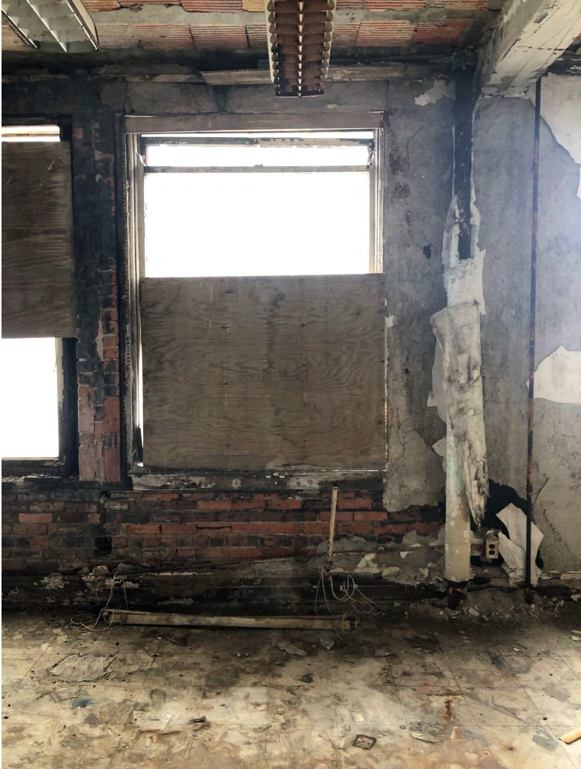
Figure #40: Interior, 11 th floor, Window Detail. 2/4/2019
