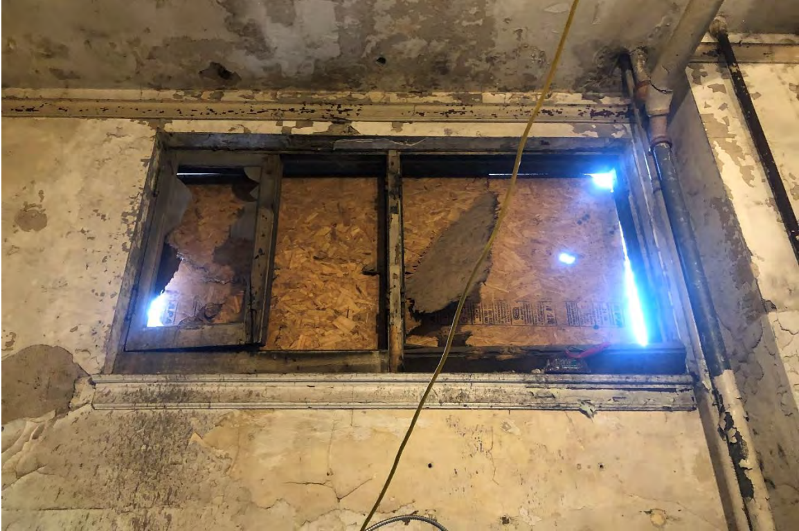
Figure #28: Interior, Window Detail. 2/4/19
