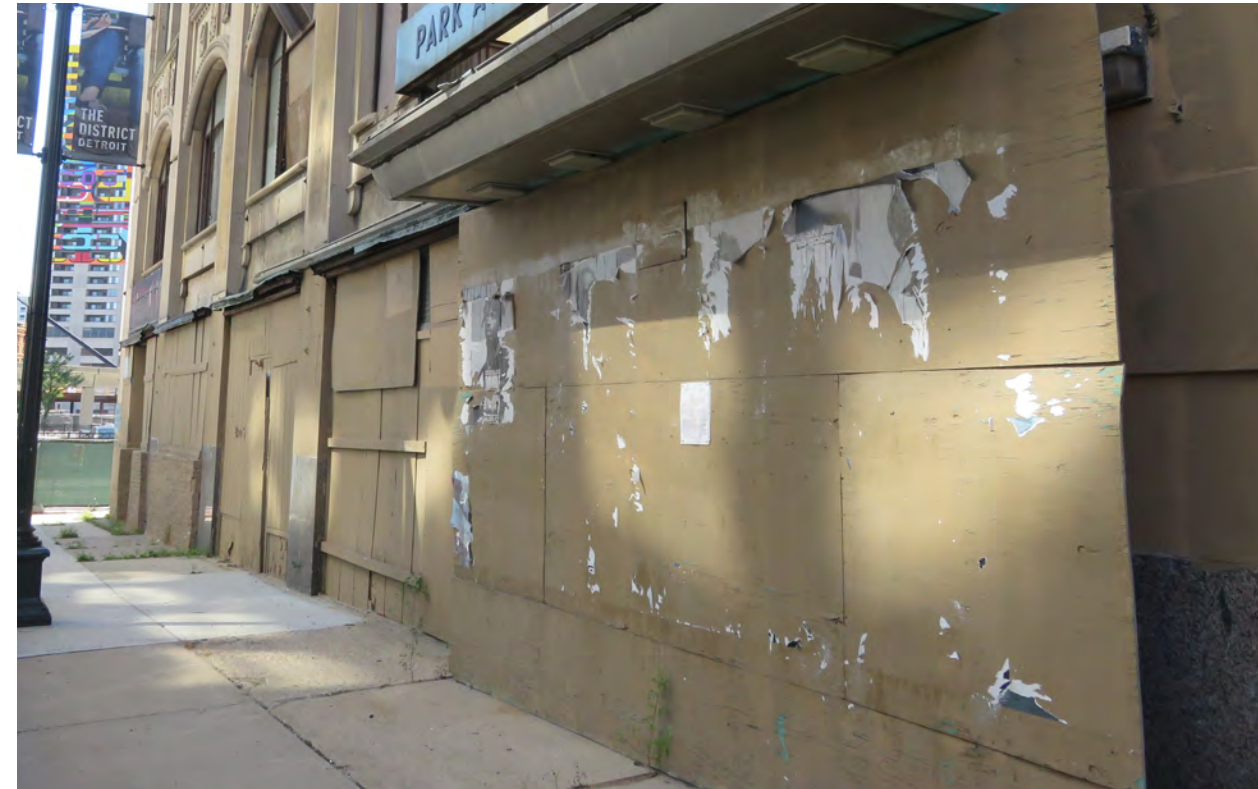
EXISTING CONDITION OF GRANITE AT EAST FACADE
