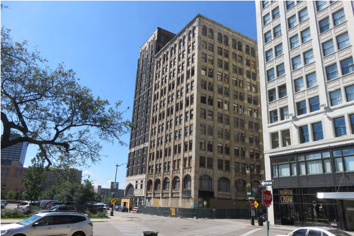
Figure #4: Exterior, East and South Facades, Looking northwest. 9/11/2018
