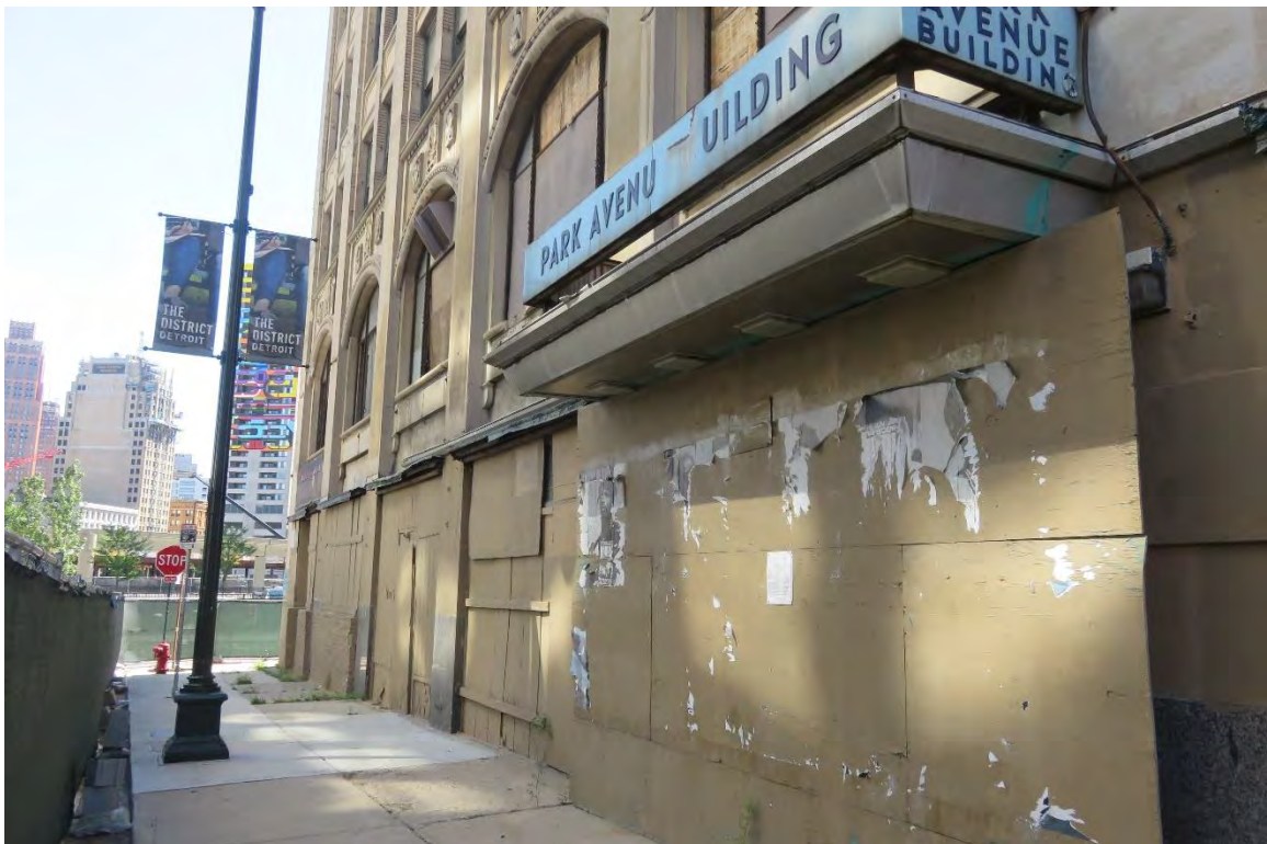
Figure #16: Exterior, canopy detail, looking southwest. 9/11/2018
