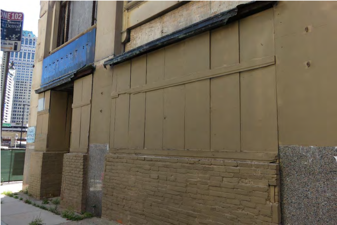
Figure #8: Exterior, looking southwest. 9/11/2018
