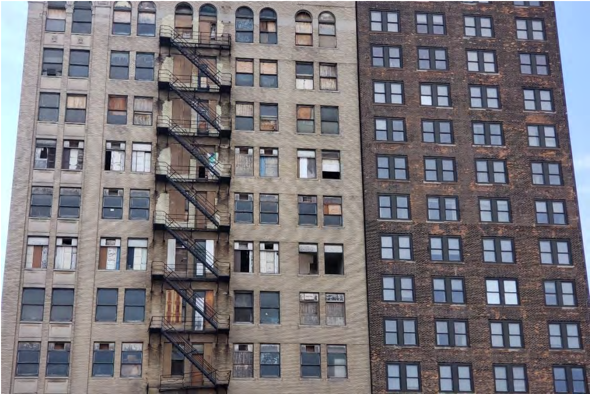
Figure #25: Exterior, Fire Escape, Looking South. 6/27/19
