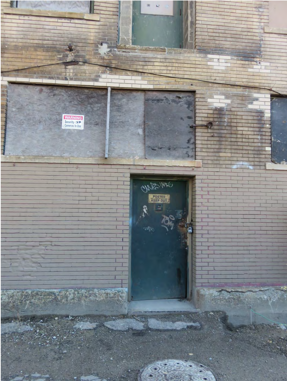
Figure #24: Exterior, North façade, Service Door. 9/11/18
