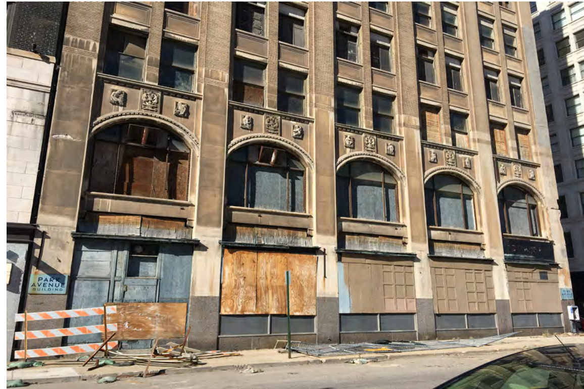
EXISTING CONDITION OF GRANITE AT SOUTH FACADE
