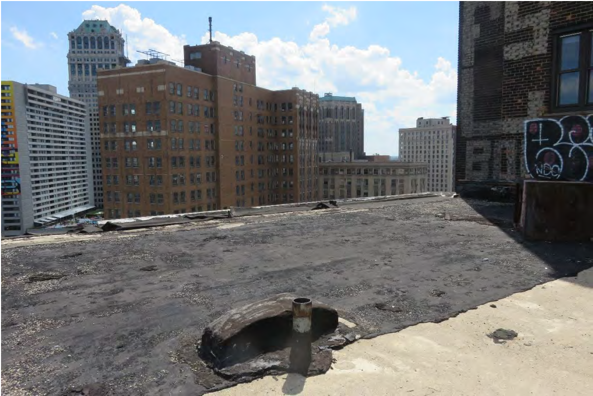
Figure #43: Exterior, roof, looking south. 9/5/2018
