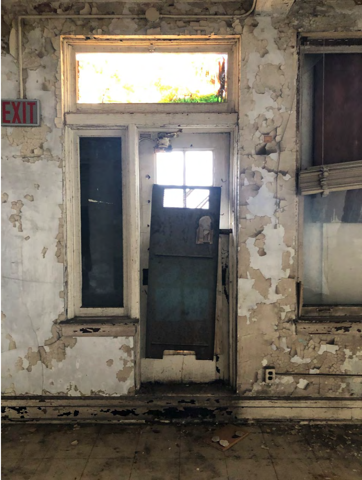
Figure #39: Interior, 11 th floor, Fire Escape Door, Looking North. 2/4/19
