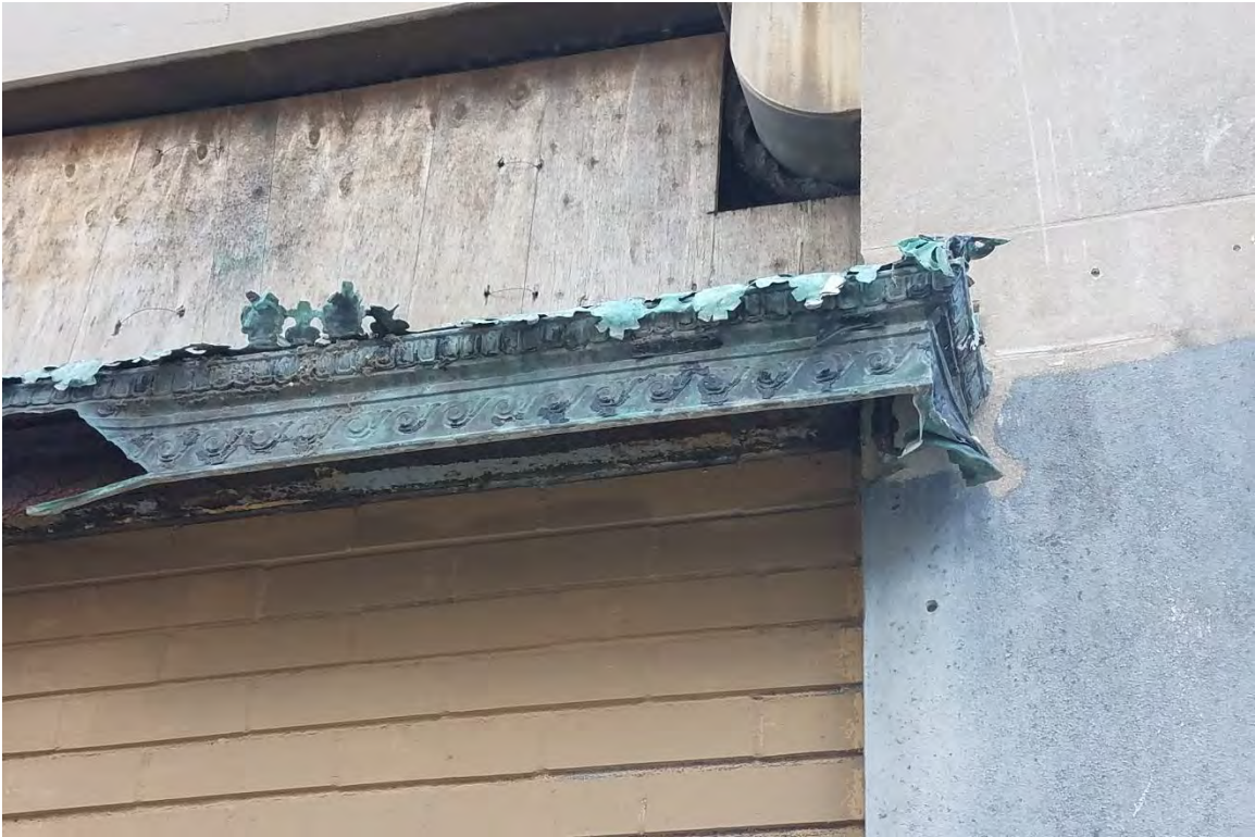
Figure #17: Exterior, metal awning enclosure detail. 9/26/2018
