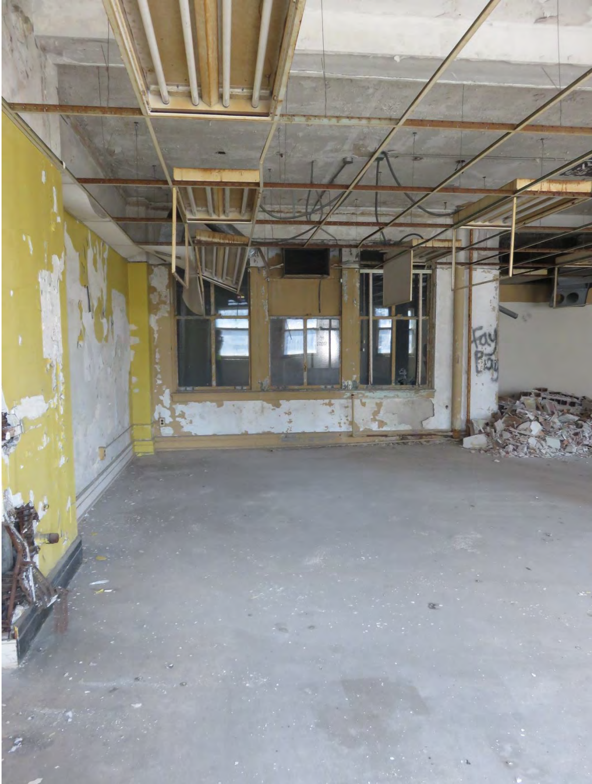
Figure #33: Interior, 5 th Floor, South lightwell window, looking north. 9/5/18
