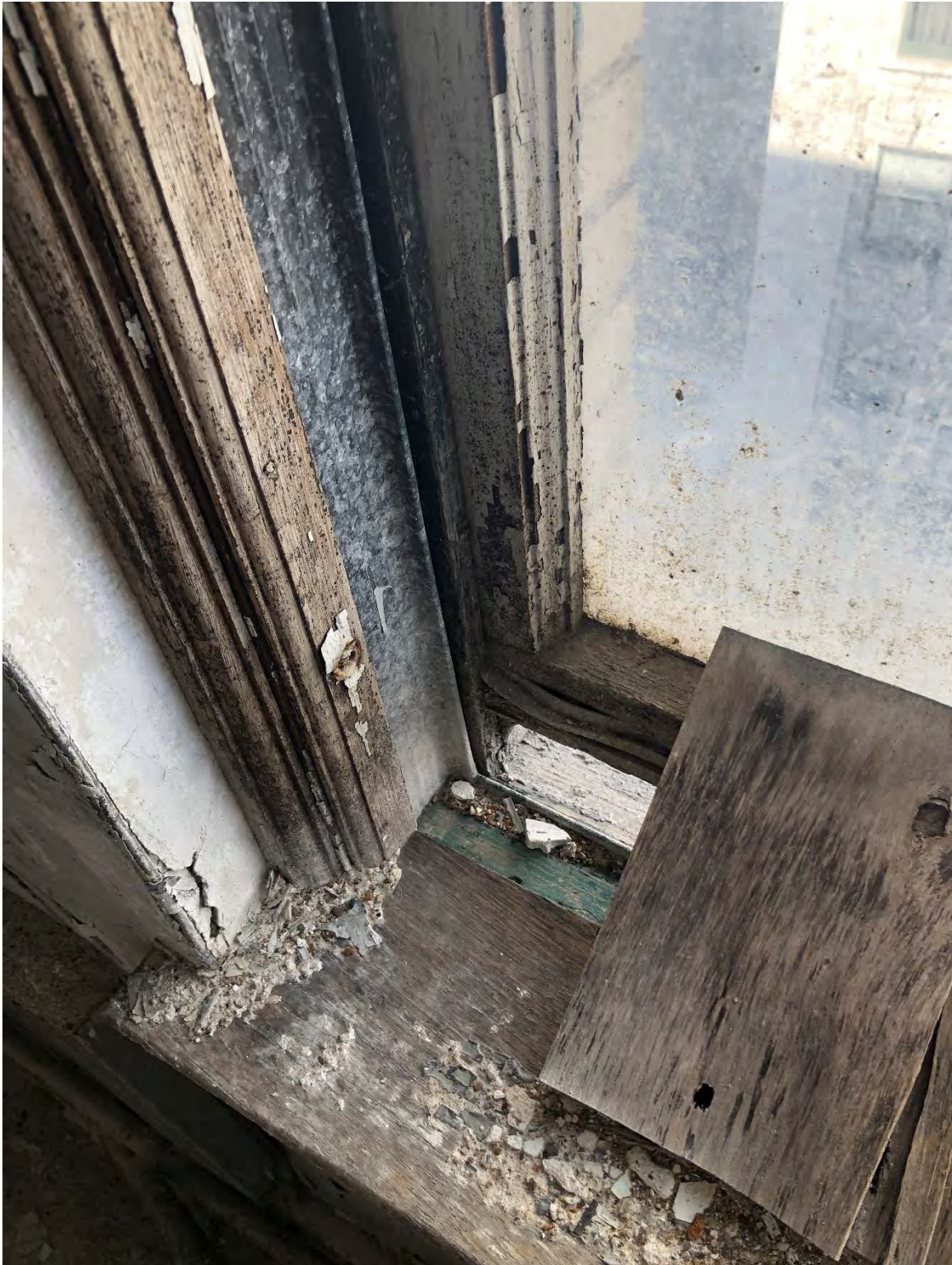
Figure #42: Interior, 12 th Floor, Window Detail. 2/25/19
