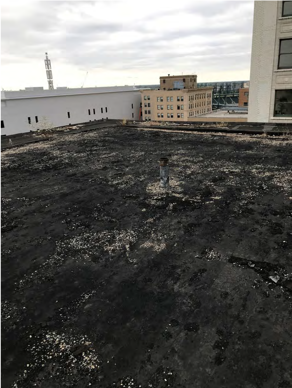
Figure #47: Exterior, roof, looking northeast. 9/5/2018
