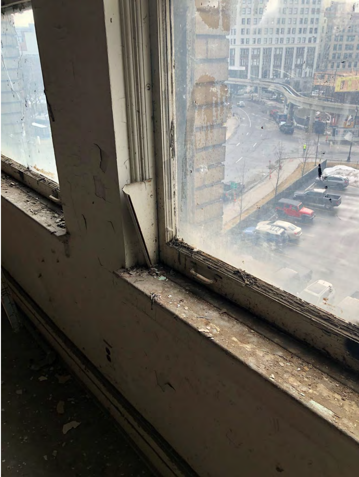
Figure #34: Interior, 5 th Floor, Window Detail. 2/4/19
