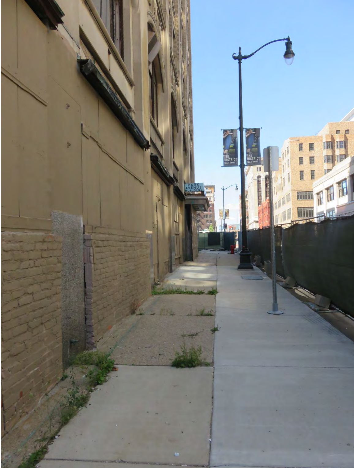
Figure #10: Exterior, looking north. 9/11/2018
