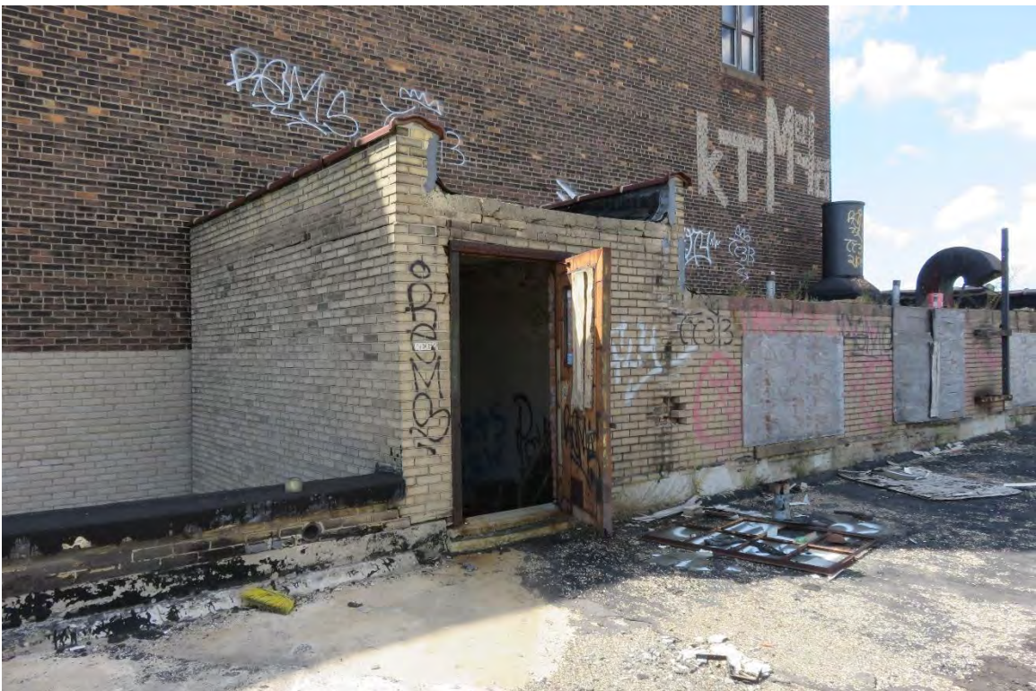
Figure #44: Exterior, roof, looking west. 9/5/2018
