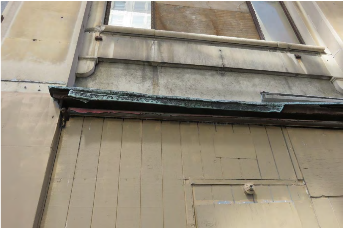
Figure #9: Exterior, looking west. 9/11/2018
