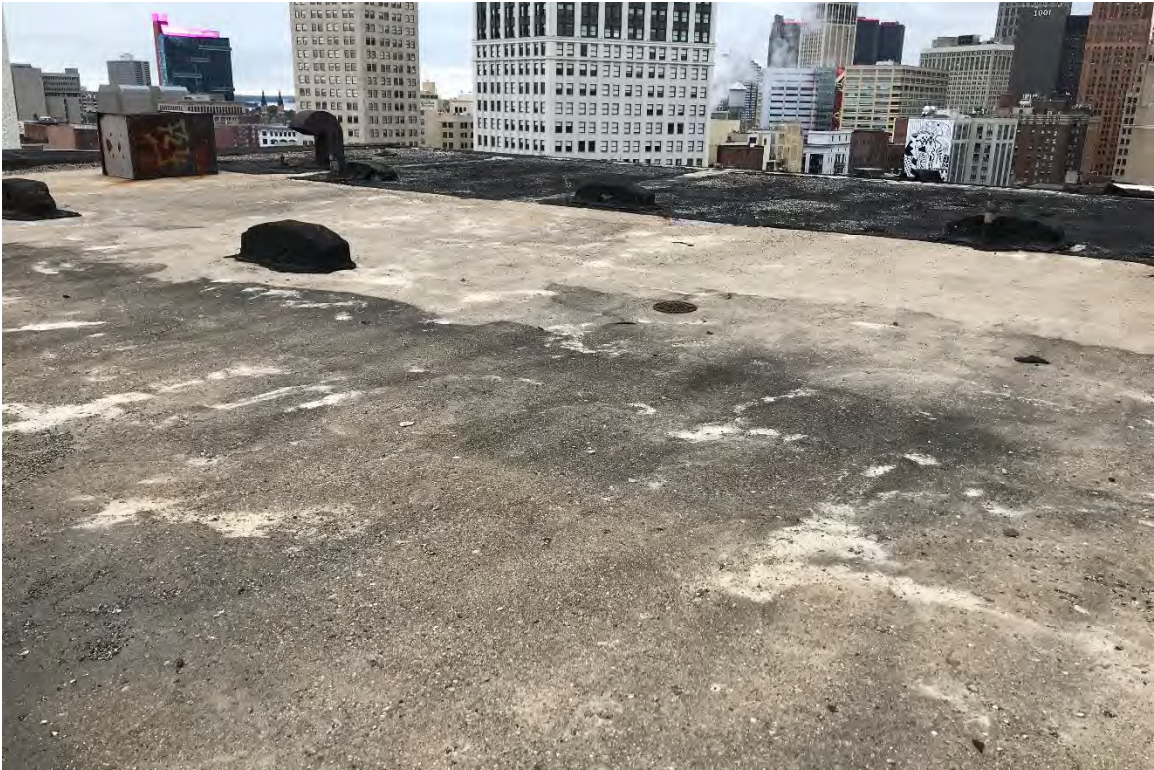
Figure #48: Exterior, roof, looking southeast. 9/5/2018
