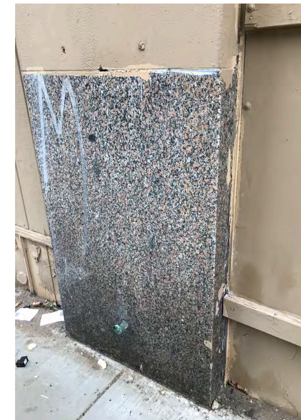
EXISTING CONDITION OF GRANITE, TYPICAL CONDITION WITH GRAFFITI
