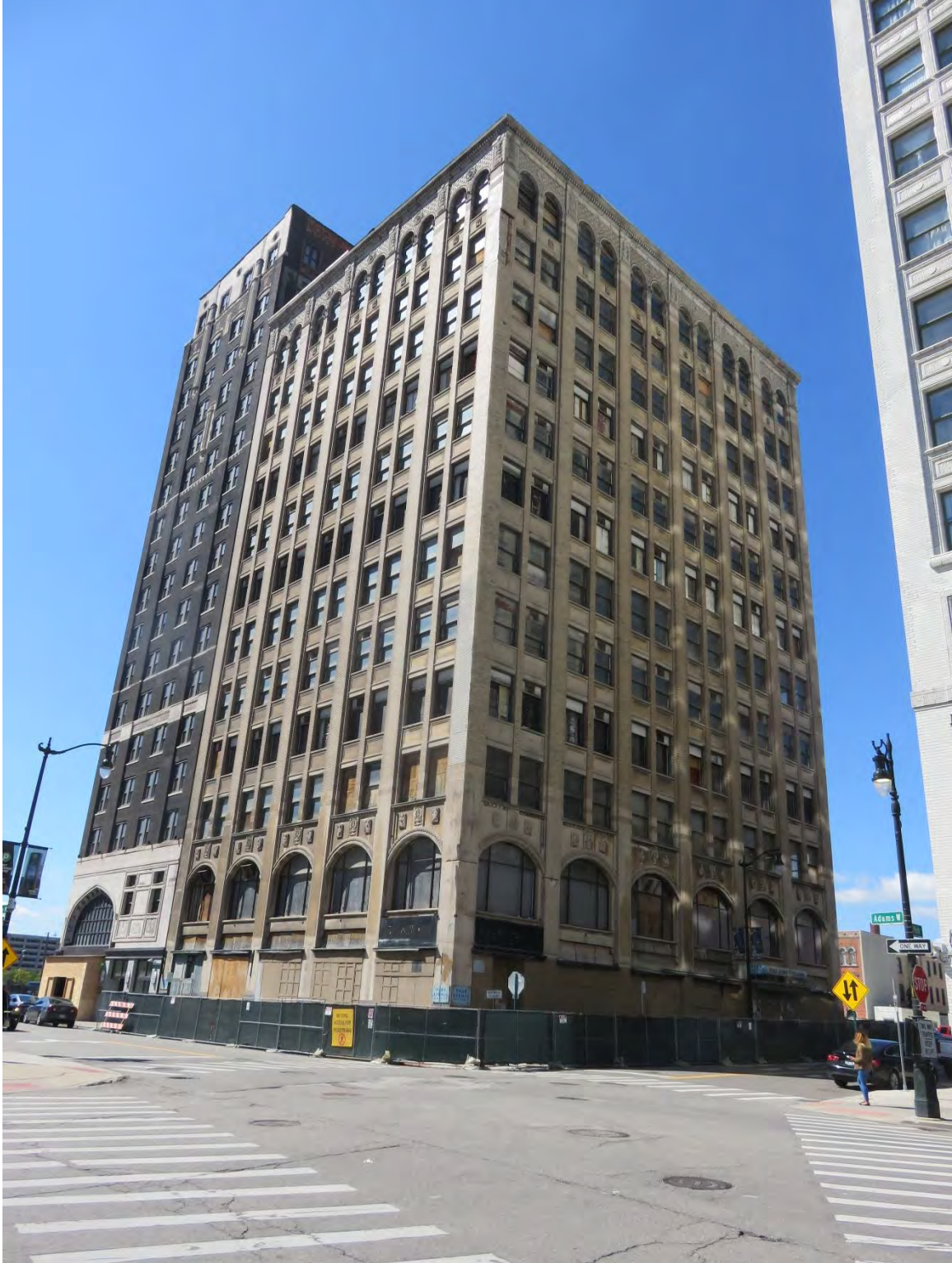
Figure #2: Exterior, East and South Facades, Looking Northwest. 9/11/18
