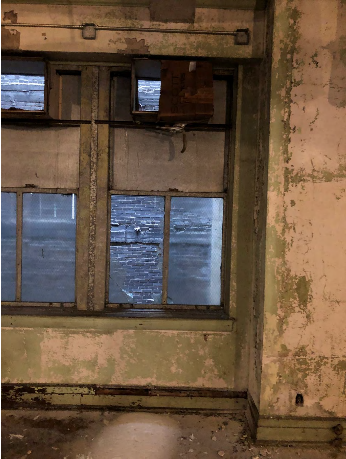
Figure #35: Interior, 7 th Floor Lightwell Window, Looking West. 2/4/19
