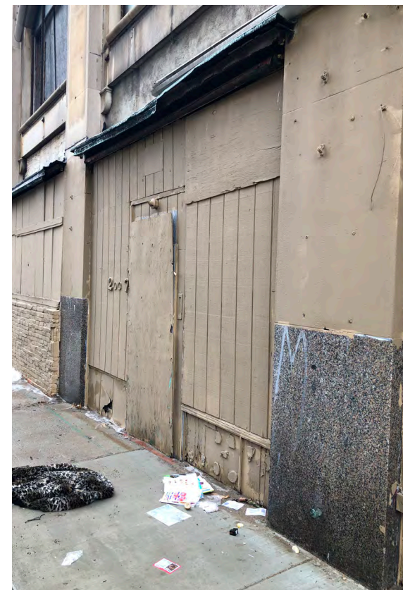
EXISTING CONDITION OF GRANITE, TYPICAL CONDITION WITH GRAFFITI
