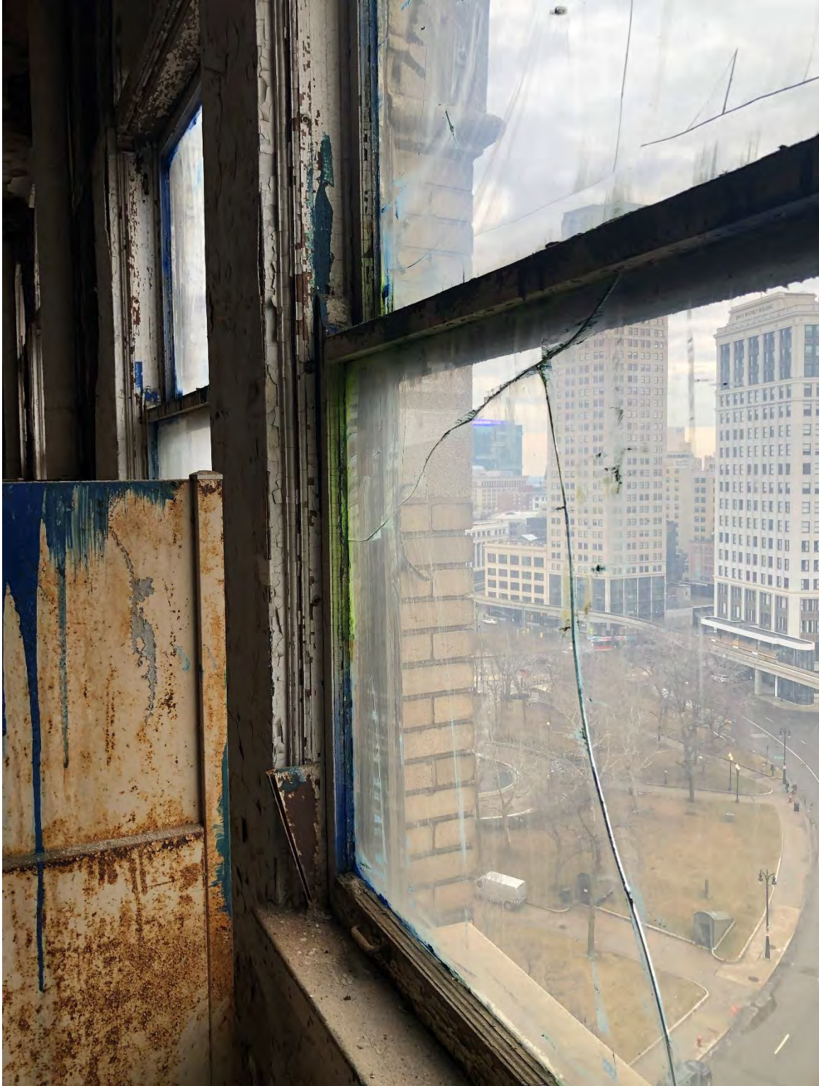
Figure #41: Interior, 12 th Floor, Window Detail, Looking Southeast. 2/4/19
