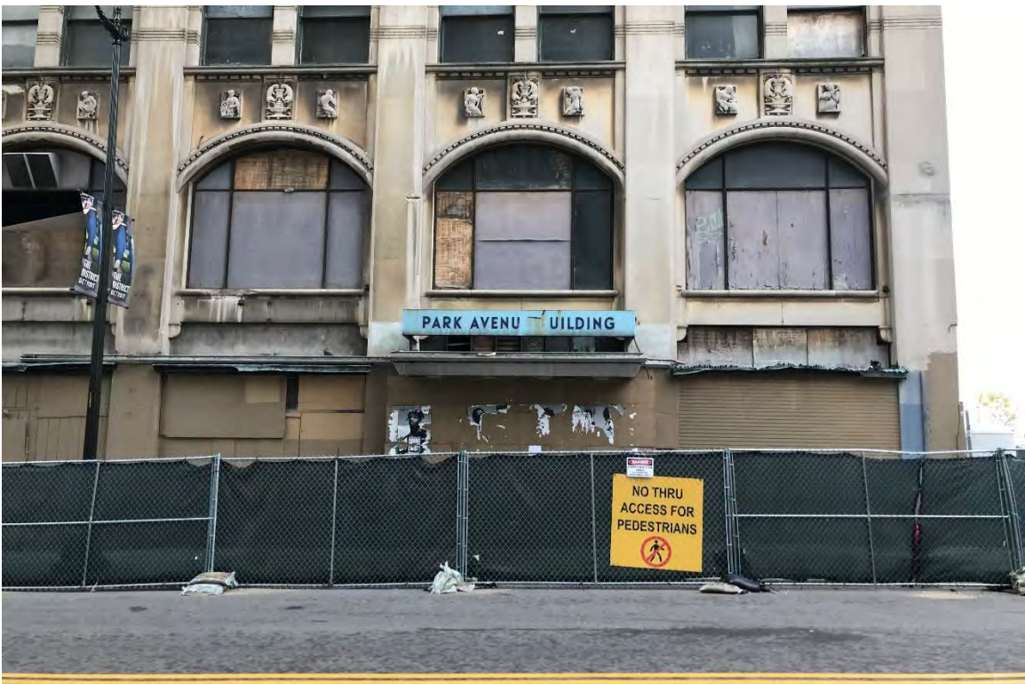
Figure #5: Exterior, looking west. 10/5/2018
