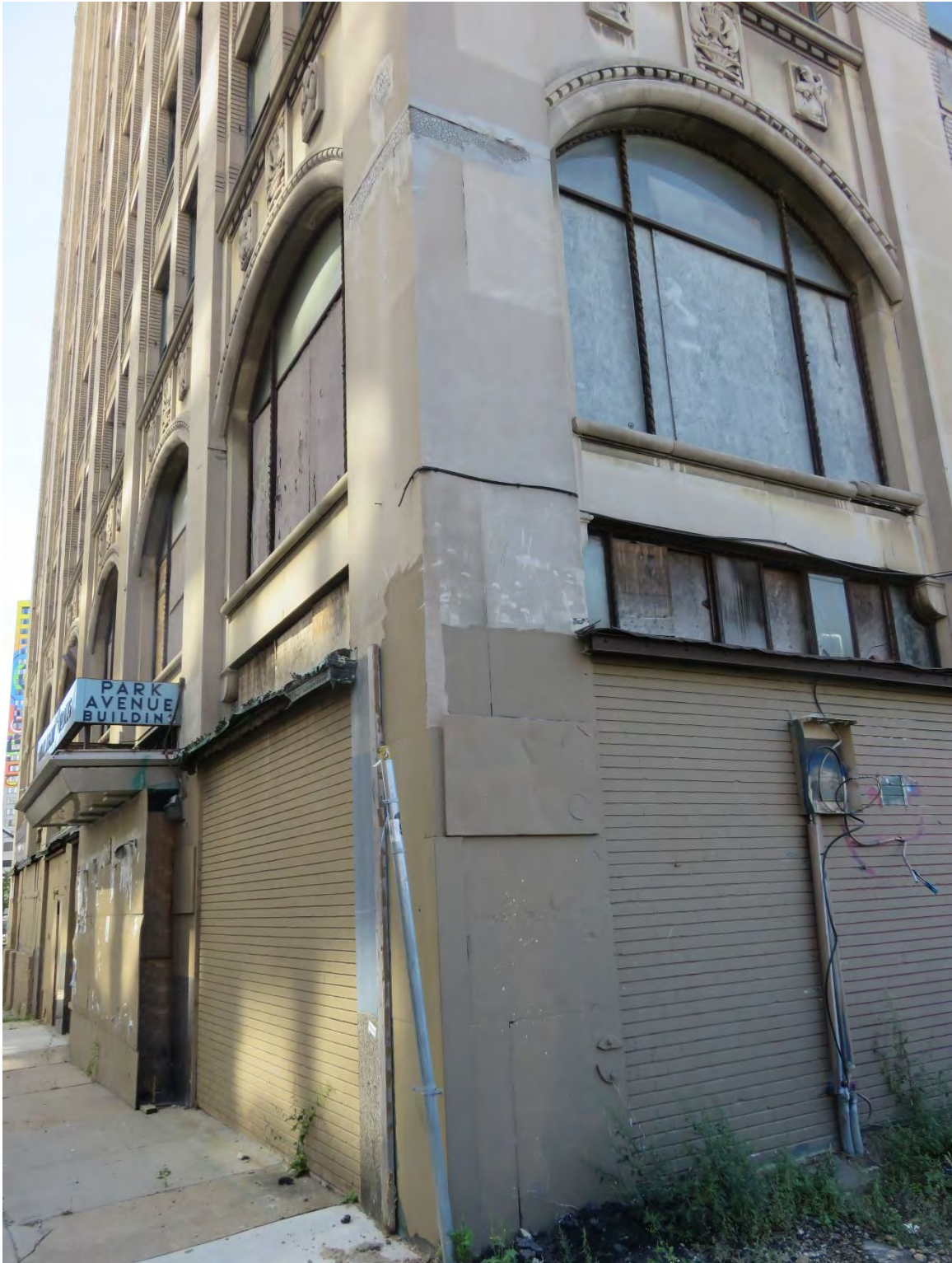
Figure #19: Exterior, window detail, looking southwest. 9/11/2018
