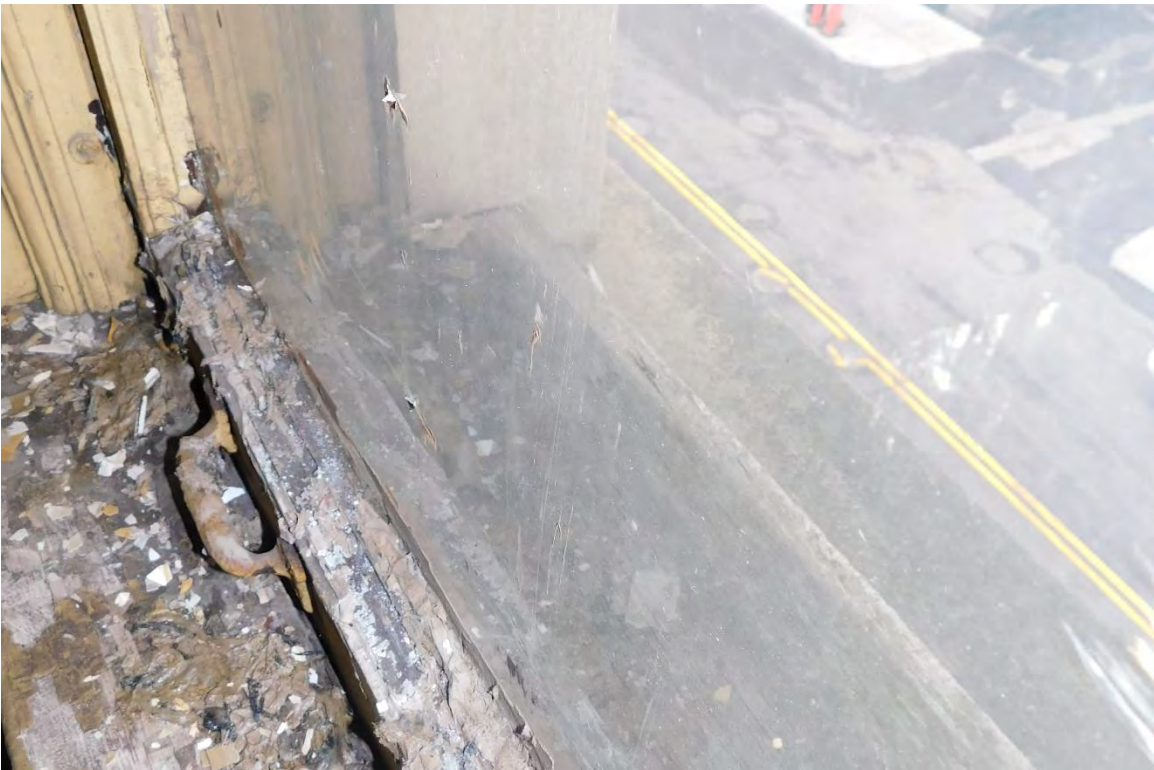
Figure #32: Interior, 3 rd Floor, Window Detail. 2/5/19
