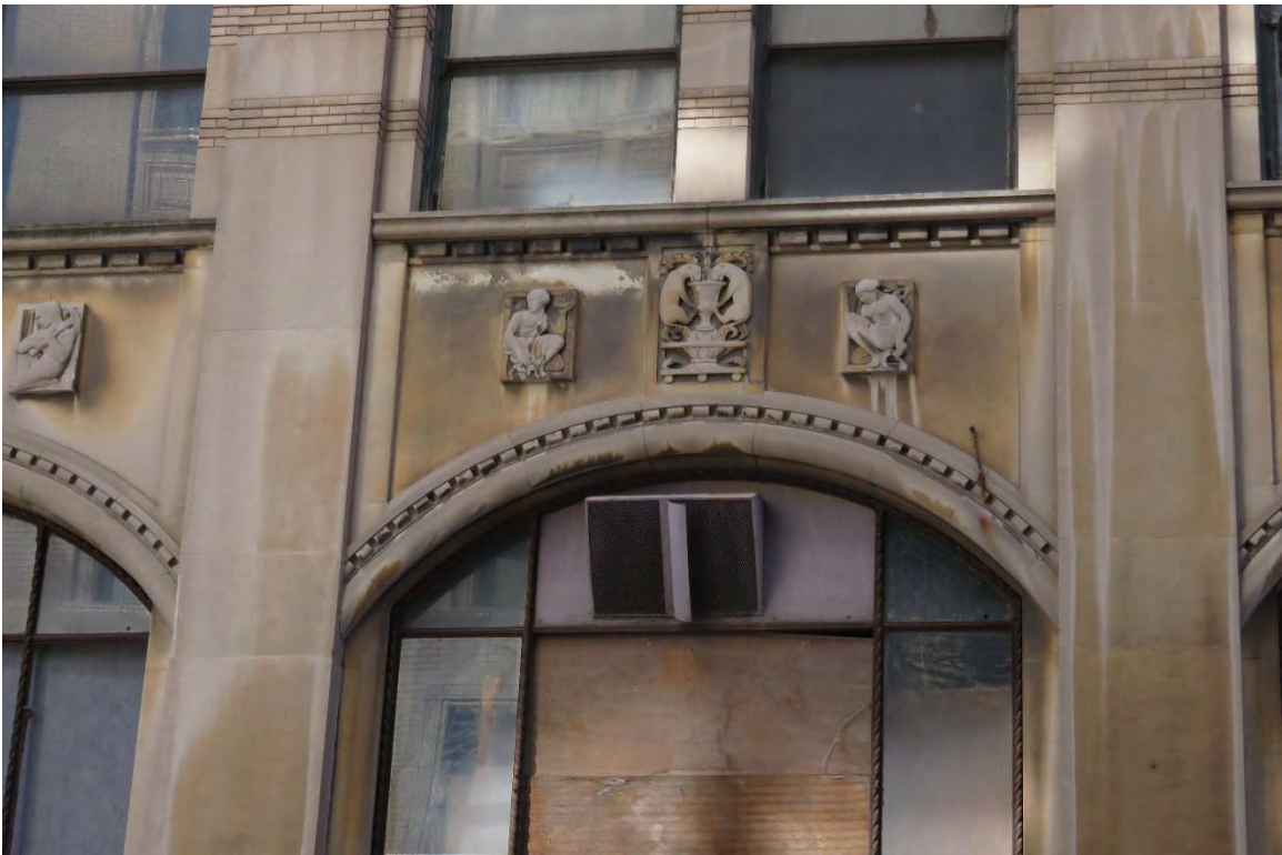
Figure #22: Exterior, window and carving detail, looking west. 9/11/2018
