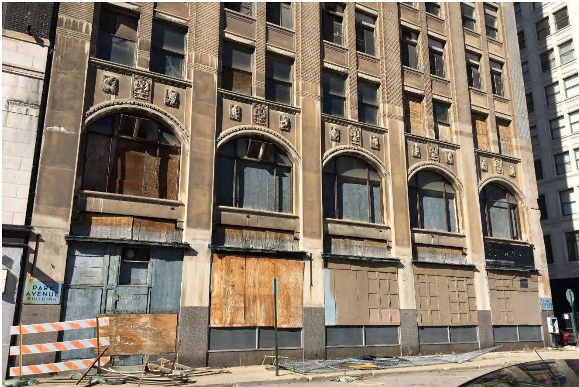
Figure #13: Exterior, South Façade, Looking Northeast. 2/25/19
