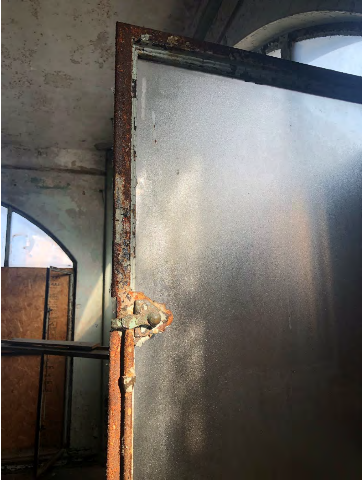
Figure #30: Interior, 2 nd Floor Window Detail. 2/4/19
