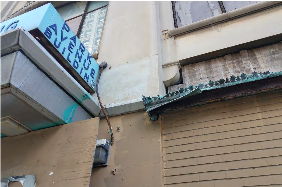
Figure #18: Exterior, canopy and awning enclosure detail. 9/26/18
