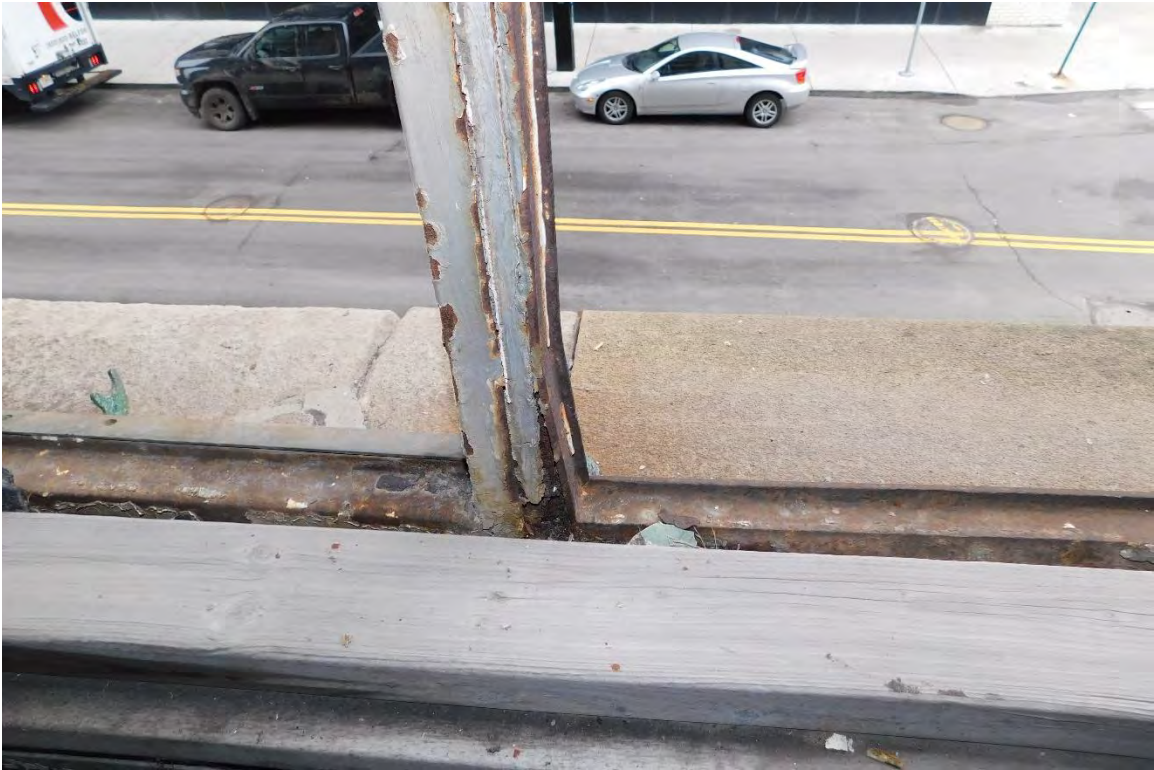
Figure #31: Interior, 2 nd Floor, Window Detail. 2/5/19
