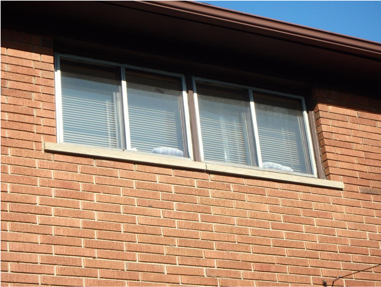
Unit 202 Replacing two gliding windows with one large 3 panel (1:2:1) gliding window
