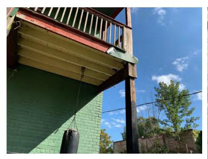
Above: (D4) RH side of deck Structural detail. Note slight bow in upper 4"x4", condition of joist over the beam, and extra blocking around the floor to floor connection.
