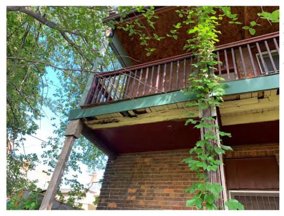
Left: (D3) Further existing decking details. Also note the O.S.B. Sheathing on the underside of the roof deck. Original has deteriorated to the point of need cover.
