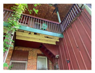
Above: (D1) Existing Decking condition, as well as stair detail shot. Note deterioration in the existing decking, as well as the condition of the existing board and batten (B&B) siding.
