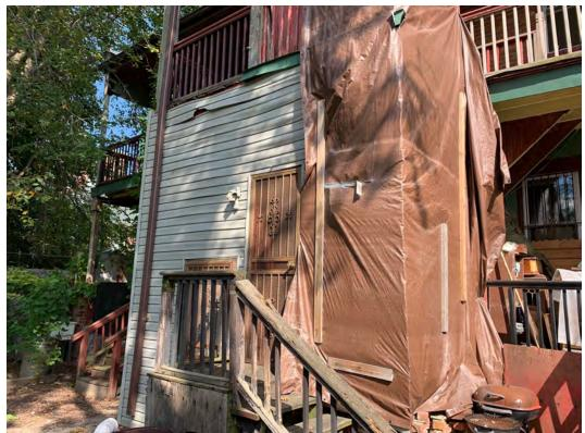
Left: (D7) Center Stair Column Detail. Area Covered by Tarp had a Tree Strike. Fair Amount of damage, Interior has been braced by homeowner temporarily.
