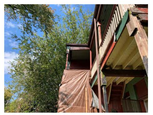
Left: (D9) Profile of center stair column. Notice the bow on the outer-most post on the stair column. The middle column floor to floor connection also shows serious water damage.
