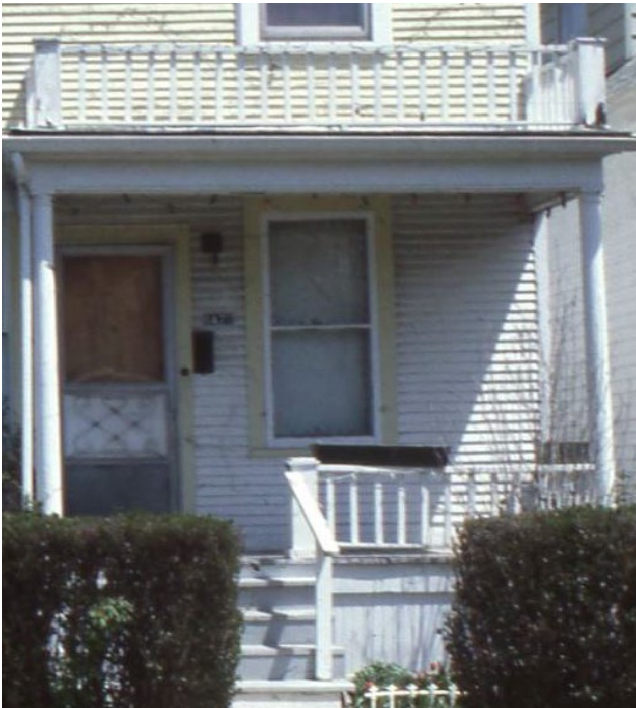
DESIGNATION SLIDE – MAY 1983. Note round wood columns & balustrade at roof and deck
