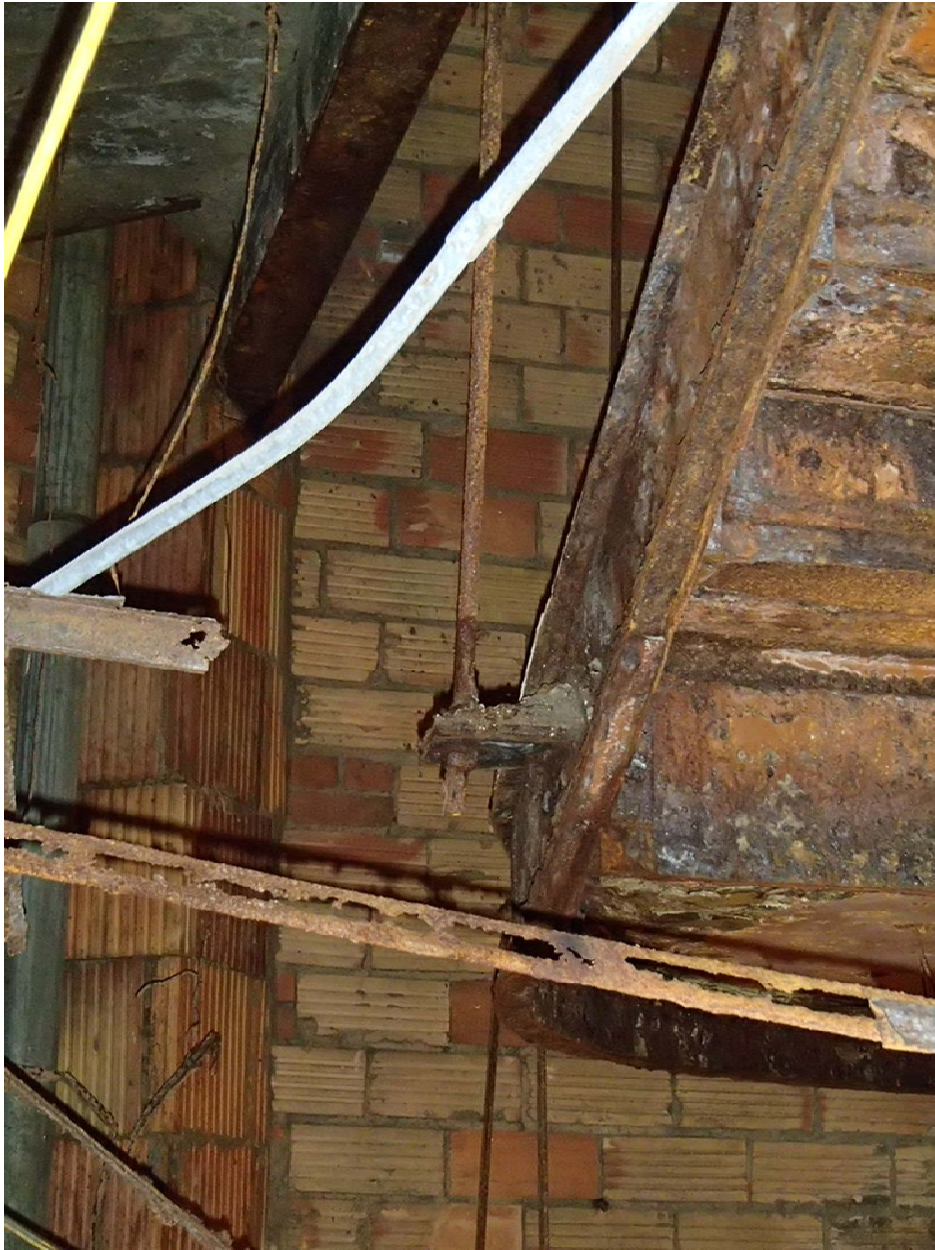
Image #10 – Interior stair stringer is supported by a hanger rod.
