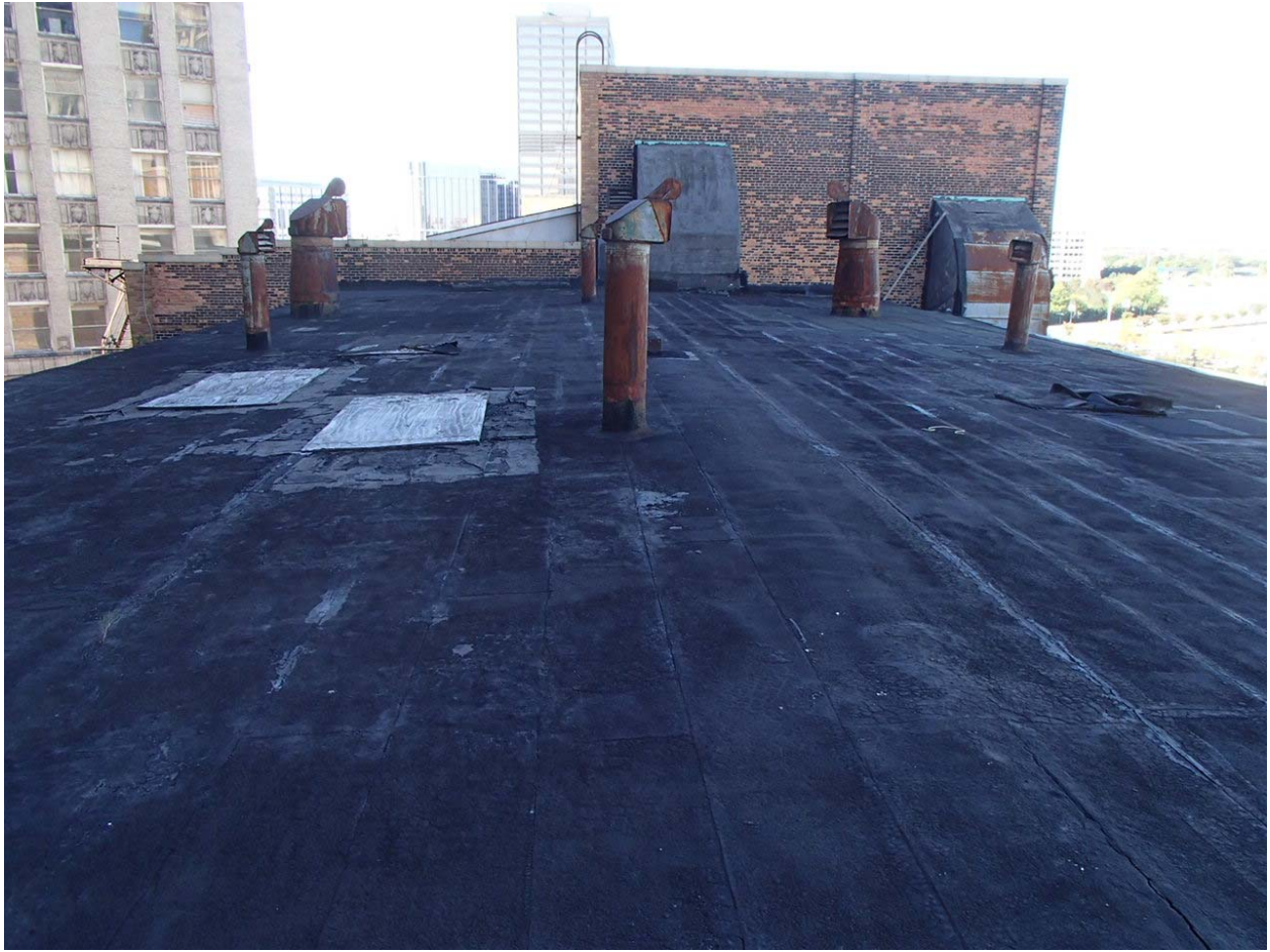
Image #12 – Main roof above theater seating area.
