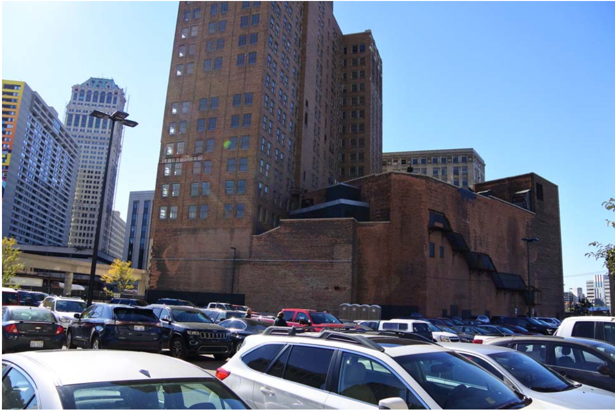
Image #26 – Exterior view from West Adams Street across parking lot. The brickwork facing the parking lot has areas of deterioration.
