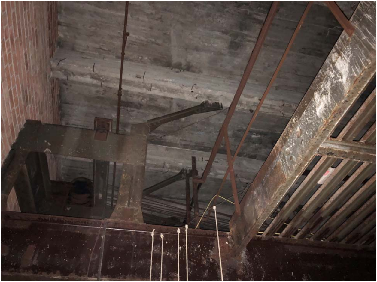
Image #31 – Concrete roof structure above fly loft.
