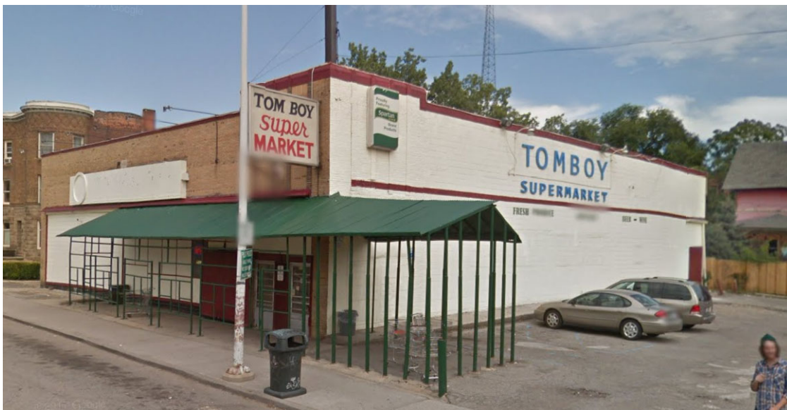
Google Earth Image dating from 2011, appearance prior to 2015 rehab
