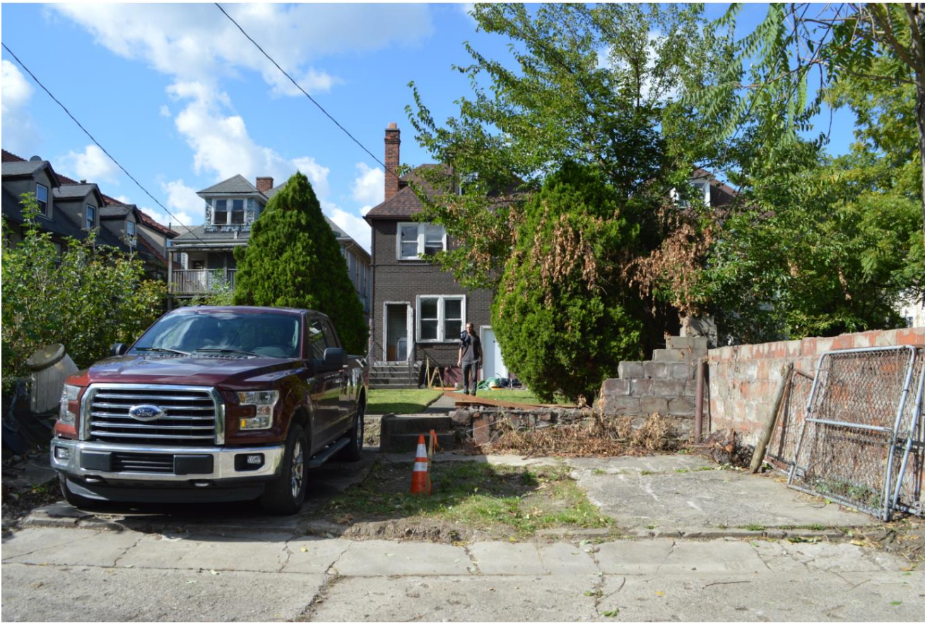
Looking west in rear yard, he is standing at approximate location of new wall at edge of lot, wall on right to remain
