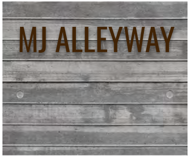
C.I.P. CONCRETE PLANTER WITH STEEL LETTERING
