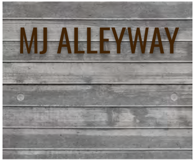
C.I.P. CONCRETE PLANTER WITH STEEL LETTERING
