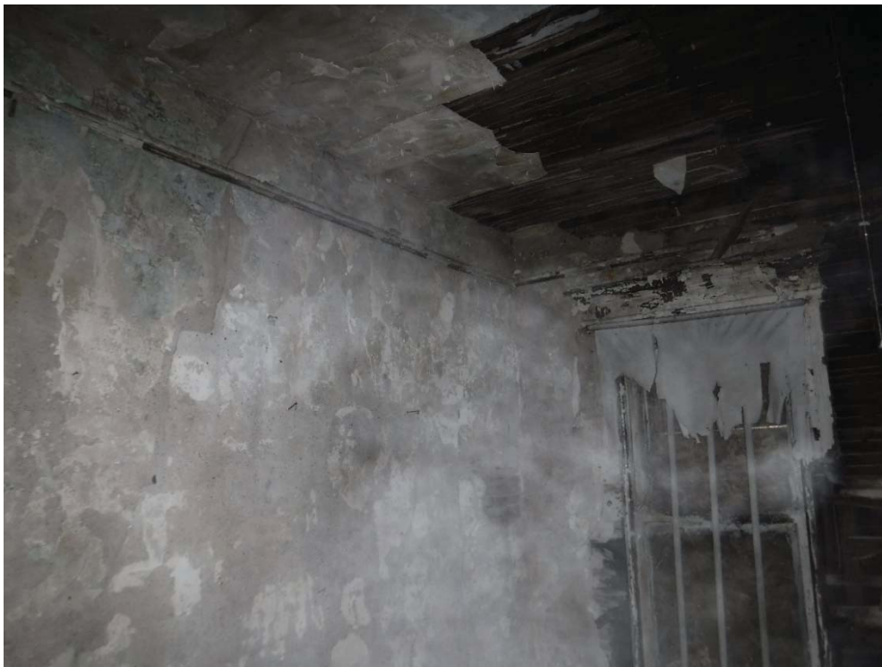
Photo 22: Interior room at 1 st floor
