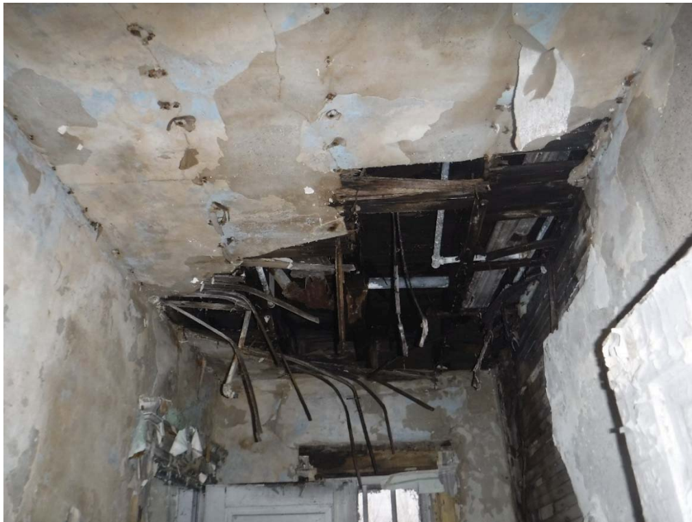
Photo 18: Interior room with pipes exposed at ceiling
