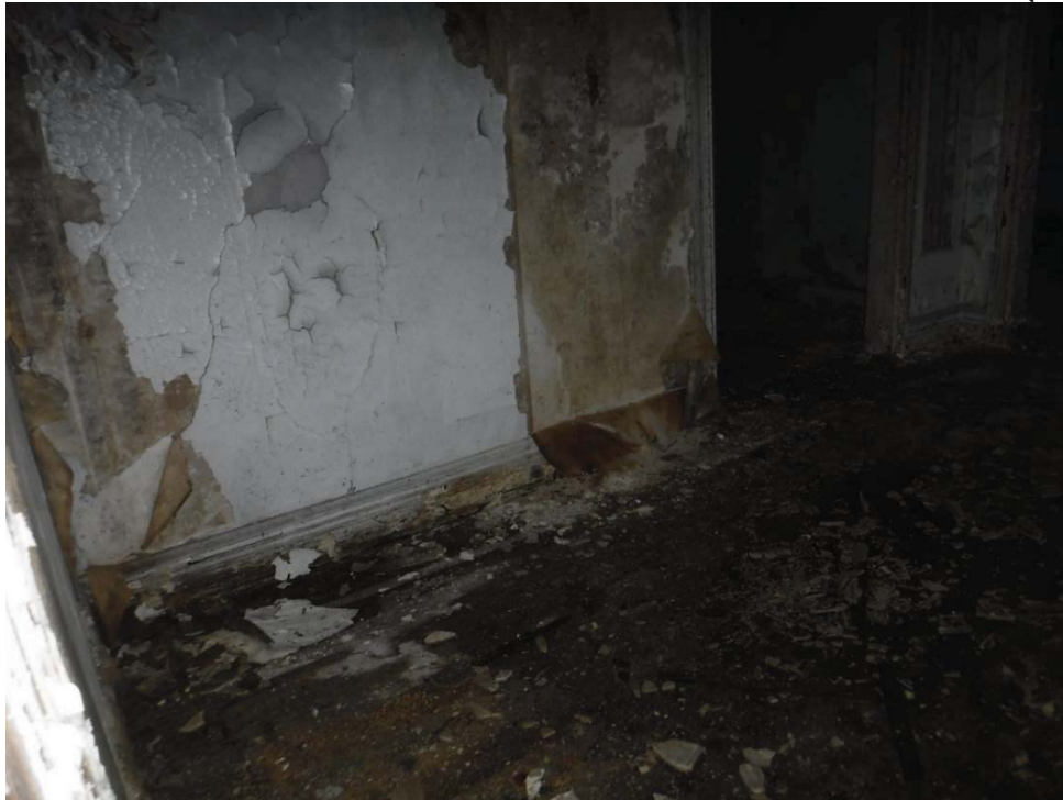
Photo 23: Interior room at 1 st floor
