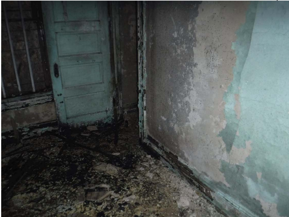
Photo 25: Interior room at 1 st floor
