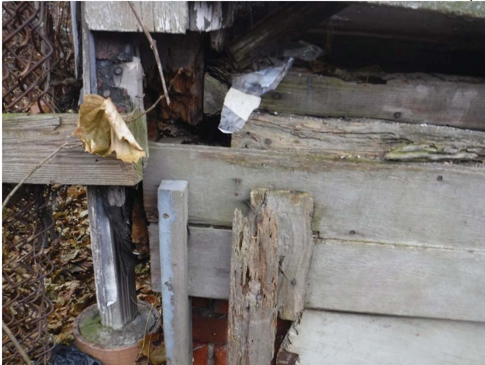
Photo 35: North-east corner of crawl space
