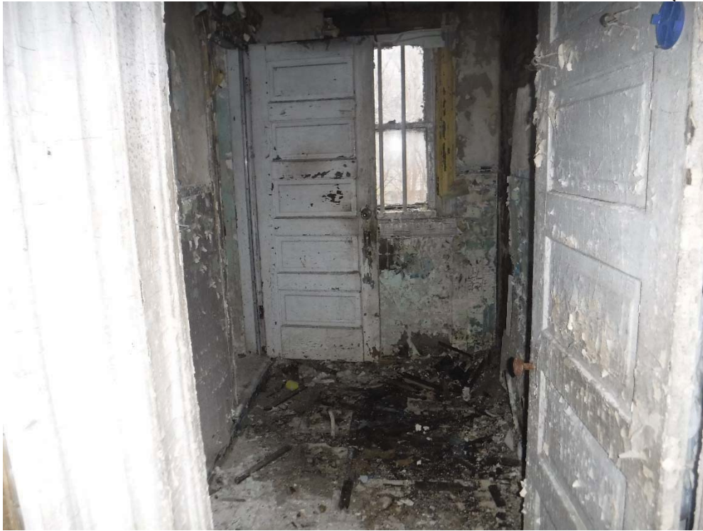
Photo 17: Interior room at 1 st floor
