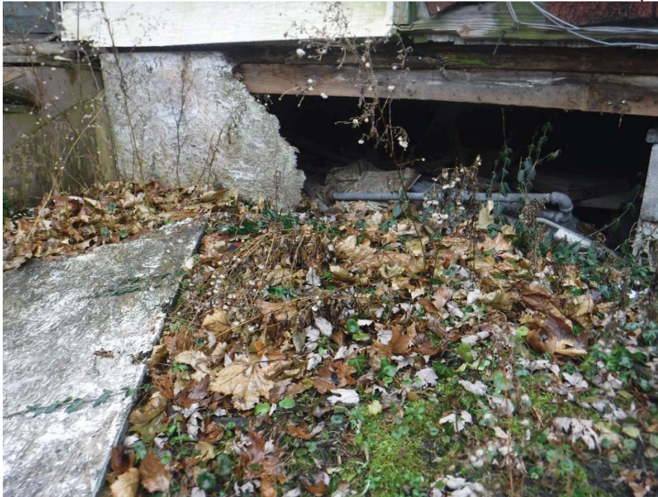
Photo 11: Rear opening at crawl space
