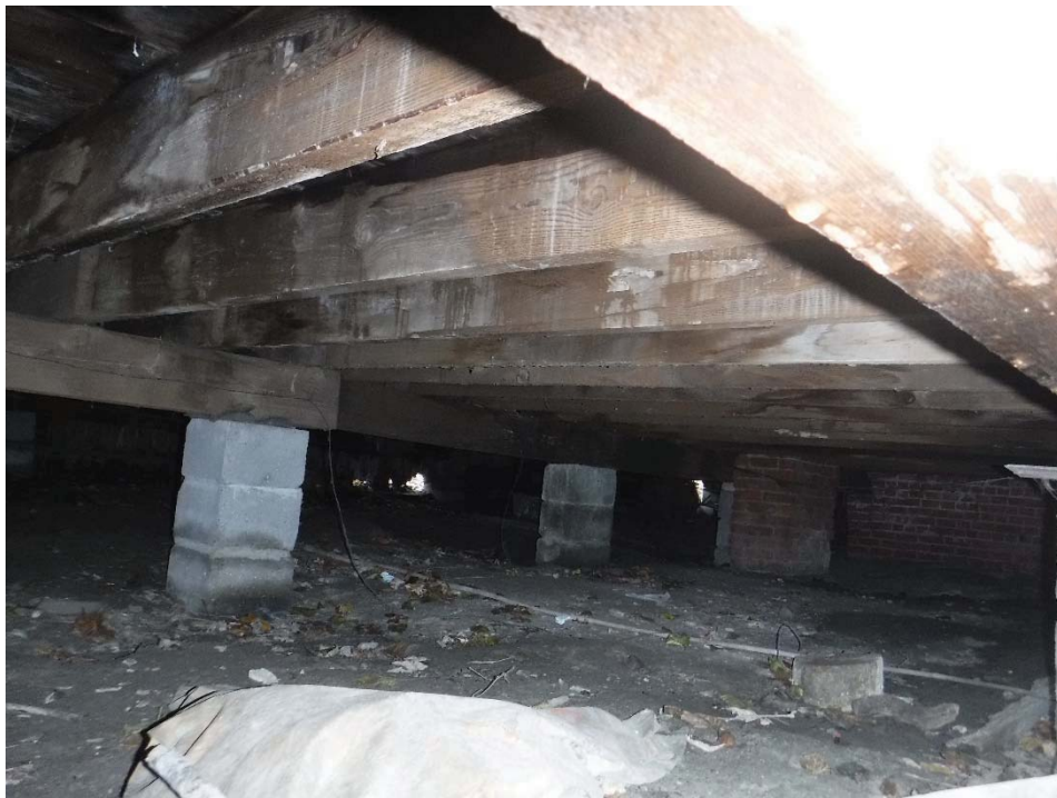
Photo 6: Crawl space framing
