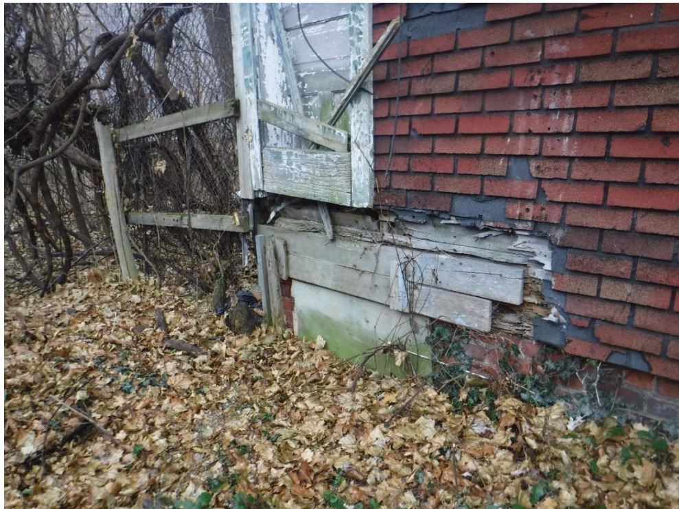
Photo 34: Rear north-east corner
