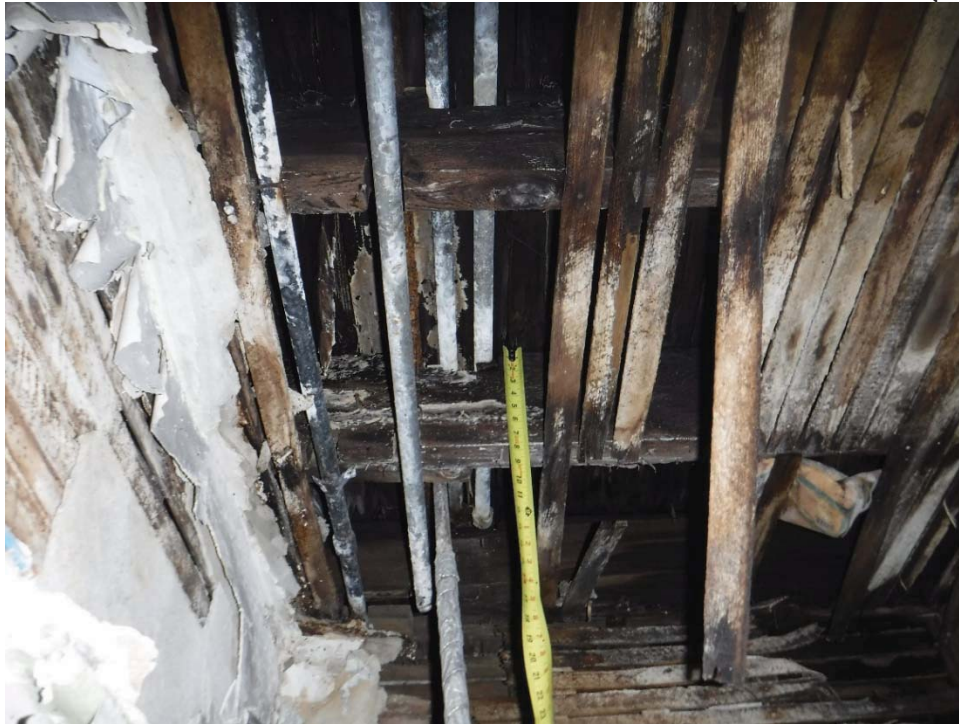
Photo 21: Interior room with ceiling joists and plumbing pipes exposed
