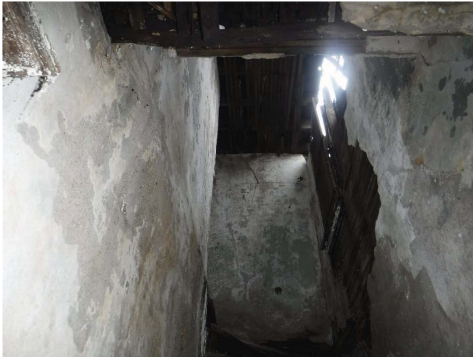
Photo 30: Stair landing with exterior wall opening
