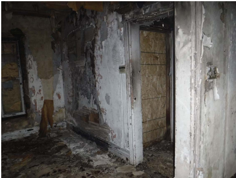
Photo 26: Interior room at 1 st floor
