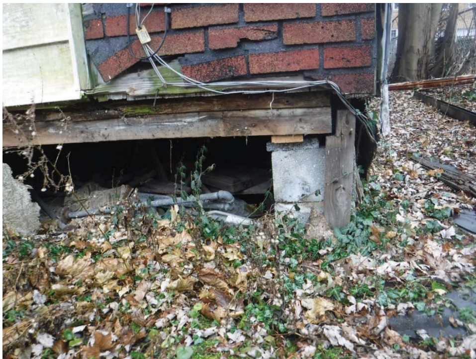
Photo 12: North-west corner at crawl space
