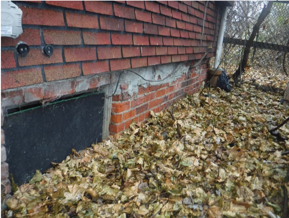
Photo 7: Crawl space opening at east side
