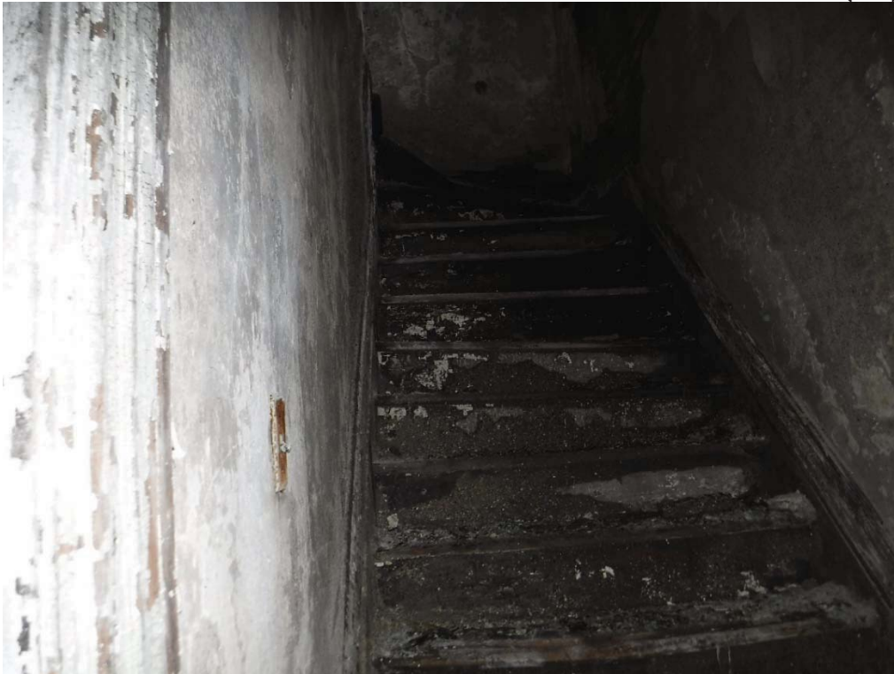
Photo 29: Stairs up to 2 nd floor
