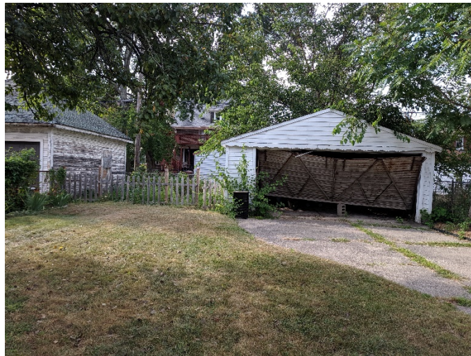
FIGURE 1 – EXTERIOR OF EXISTING GARAGE
