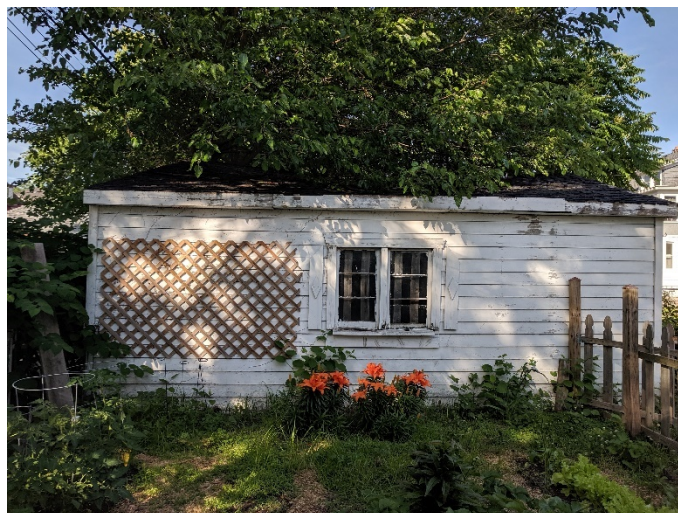
FIGURE 2 – EXTERIOR OF EXISTING GARAGE
