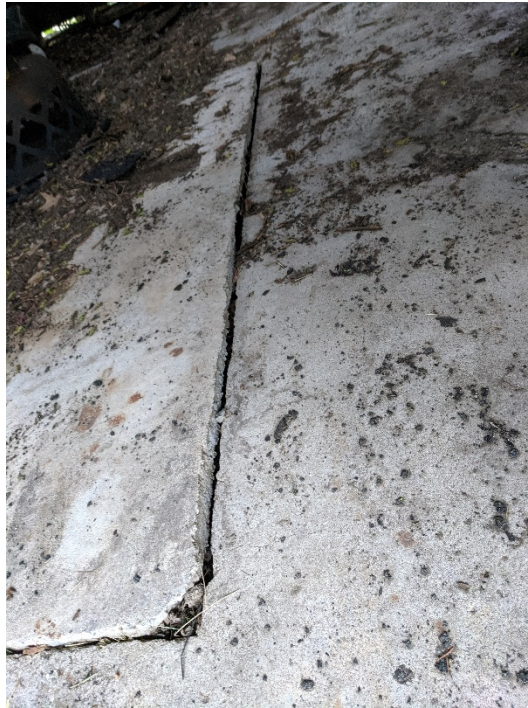
FIGURE 3 – SLAB LIFTING
