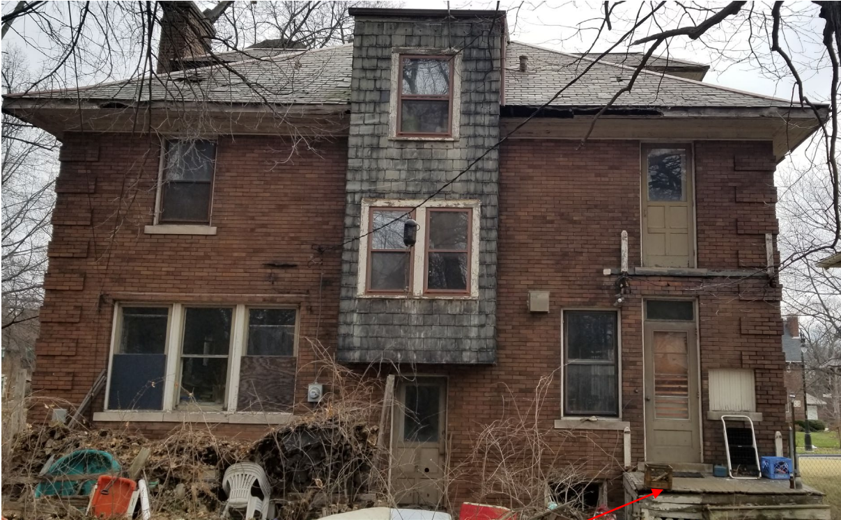
Rear elevation, current condition . Note, remaining wood deck and steps
