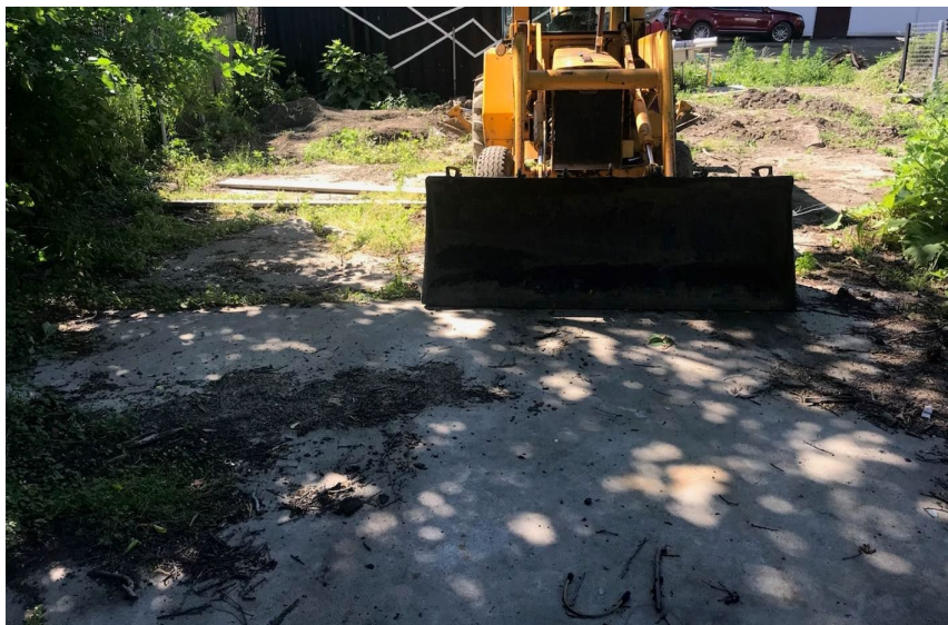
3466 Burns rear yard, current appearance. Existing concrete slab
