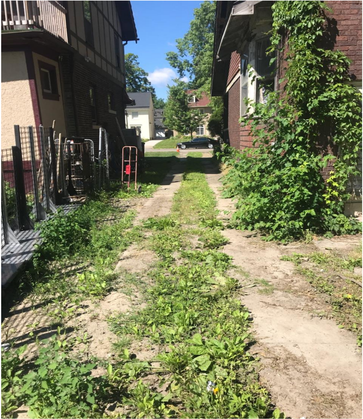
2 Lines of concrete up through the side of the house
