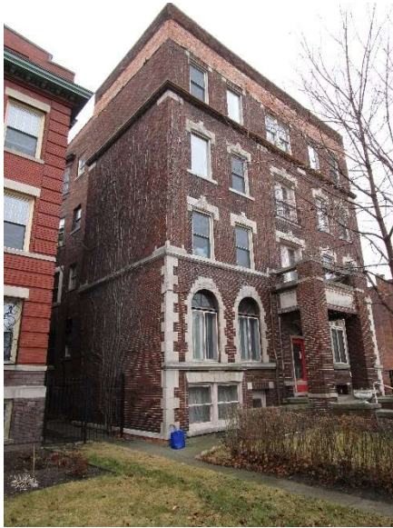
Photo 1: Covered front entrance
