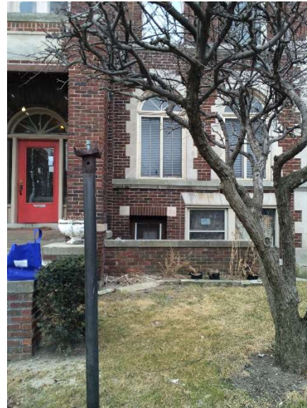
Photo 4: Stair each side to basement units
