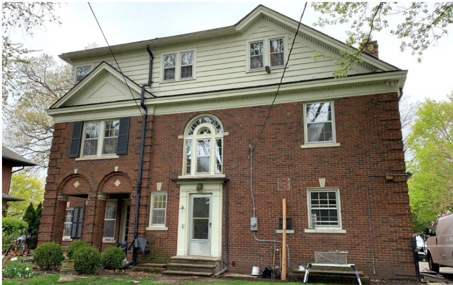
3000 Seminole. Front elevation (top photo) and rear elevation (bottom photo)
