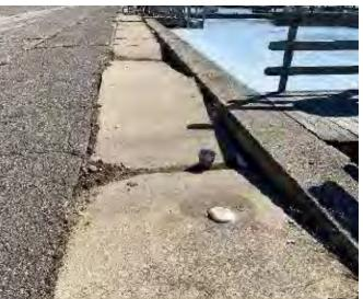
Significant settlement behind wall causing concrete walk to be uneven and potentially hazardous
