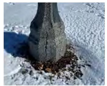
Precast concrete lighting fixtures with vertical cracking
