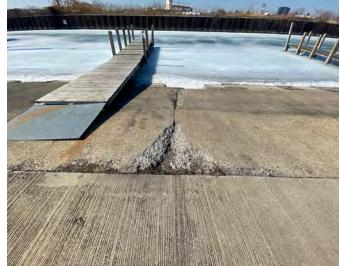
Concrete pad at the launch showing large potholes
