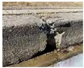
Concrete seawall shows deterioration to top of wall section requiring maintenance
