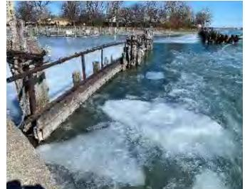
Timber pile and steel components noted to be in poor condition for breakwall at riverside entrance
