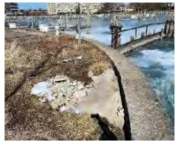
Concrete seawall in fair condition; separation in wall segments causing material loss from behind wall
