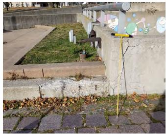
Fire and water damage to outside masonry wall in recessed area. Significant damage to painted surfaces
