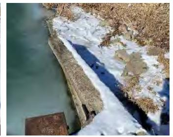
Noted deterioration of concrete seawall
