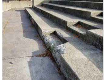
Concrete Step with numerous concrete deficiencies at walkway locations and concrete seating location
