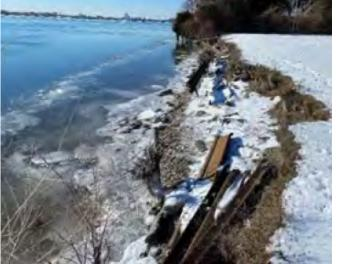
Guardrail section along shoreline is damaged and portions are missing, a potential hazard
