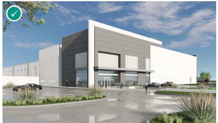
Building massing and materials articulate entrances and corners.
