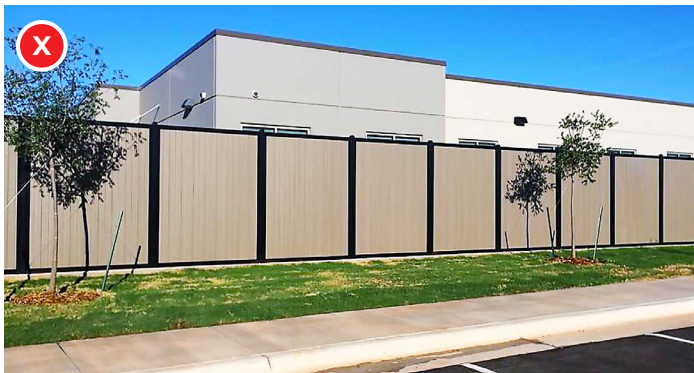
Tall, solid fencing along the ROW with sparse landscaping.
