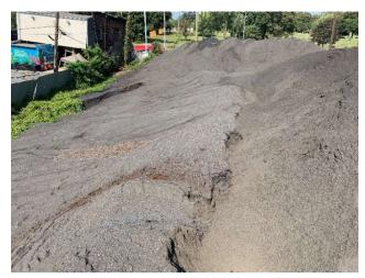
Exhibit 6 - Typical Slope Failure
