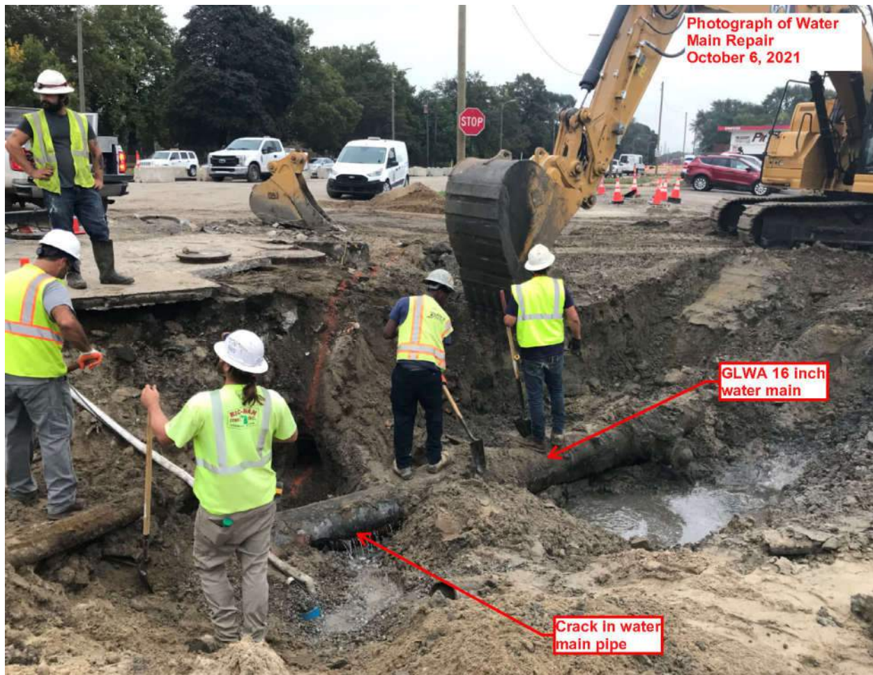
Exhibit 2 - Repair of Watermain
