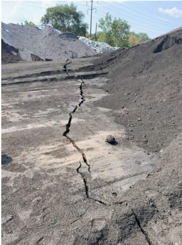
Exhibit 5 - Surface Cracking around Stockpile
