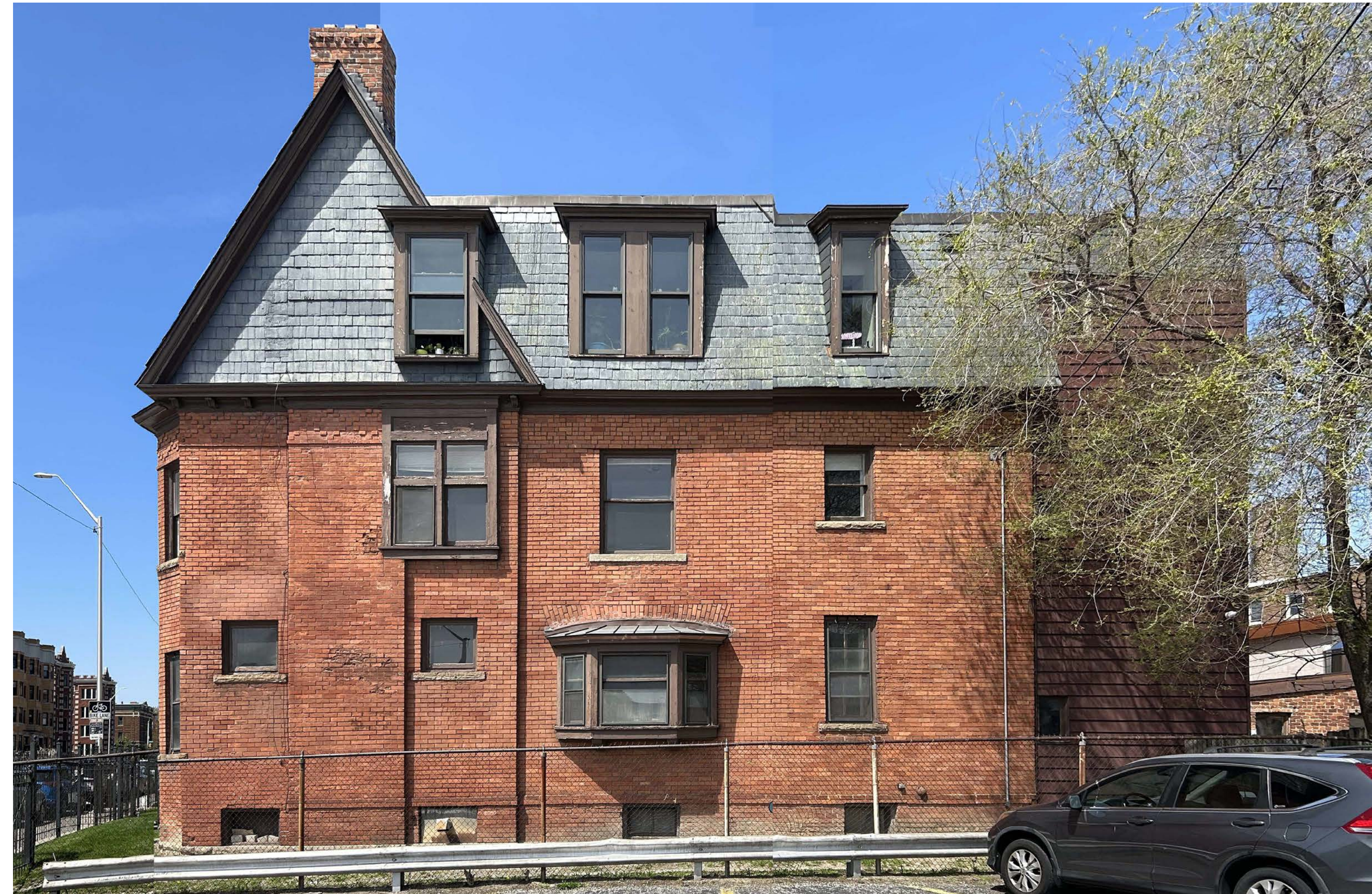
2 PHOTOGRAPH OF SOUTH FACADE EXISTING CONDITIONS
