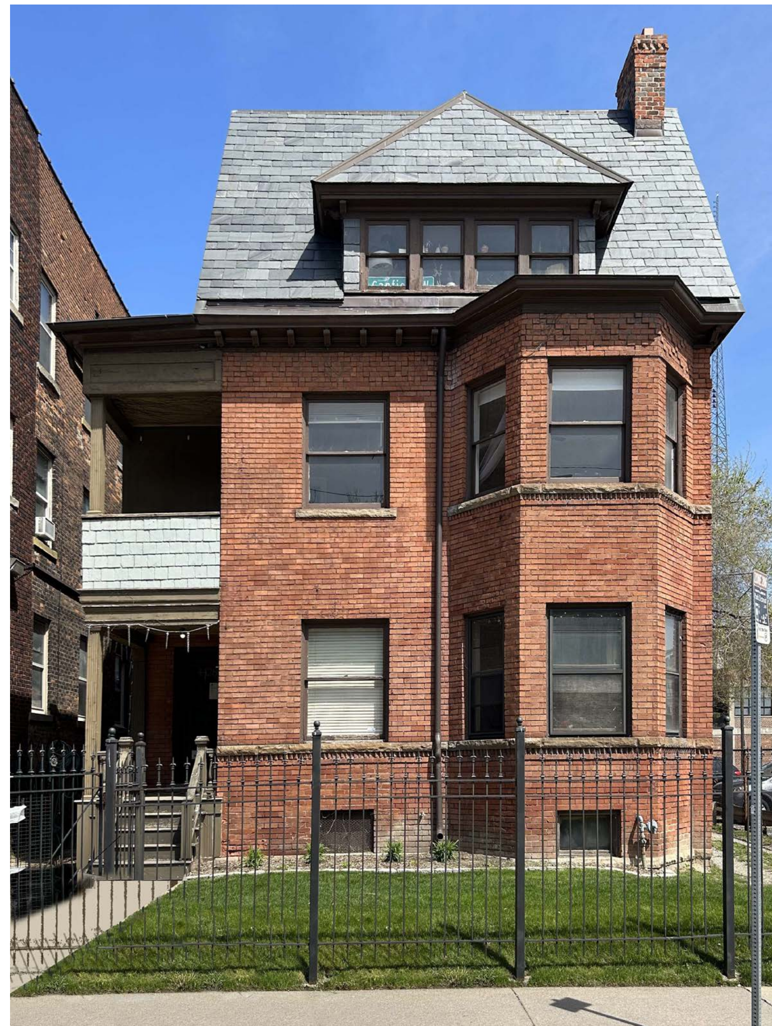
1 PHOTOGRAPH OF WEST FACADE EXISTING CONDITIONS
