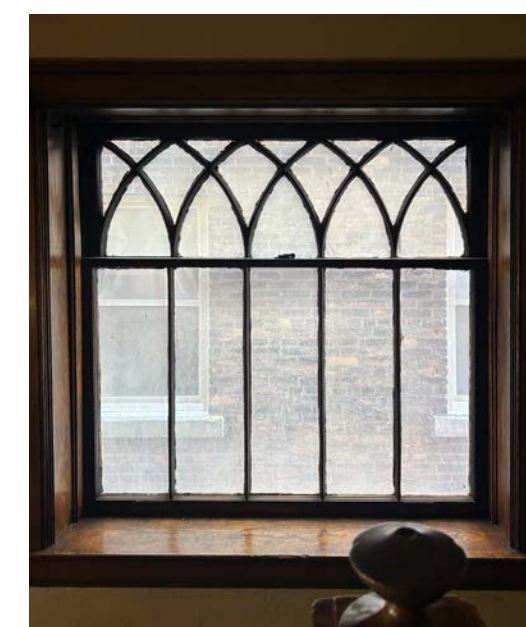
EXISTING WINDOW TO REMAIN
