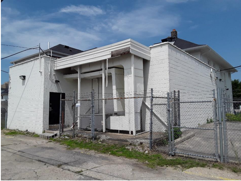
Rear face of 2648 West Grand Boulevard
