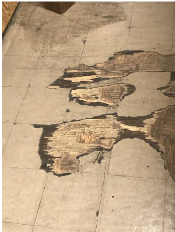
Photograph 1: Asbestos-containing 9” x 9” floor tile-light tan (HA3). Mastic is non-ACM.
