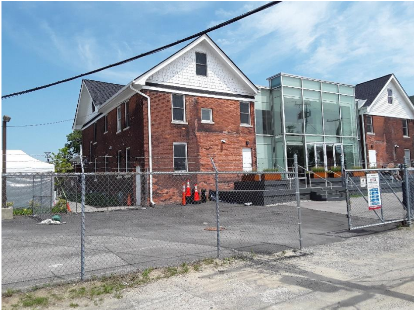
Rear face of 2650-2666 West Grand Boulevard
