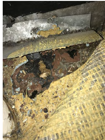
Photograph 2: Asbestos-containing 9” x 9” floor tile-dark red (HA8), with asbestos-containing 9” x 9” floor tile-teal (HA7) below. Mastics are non-ACM.
