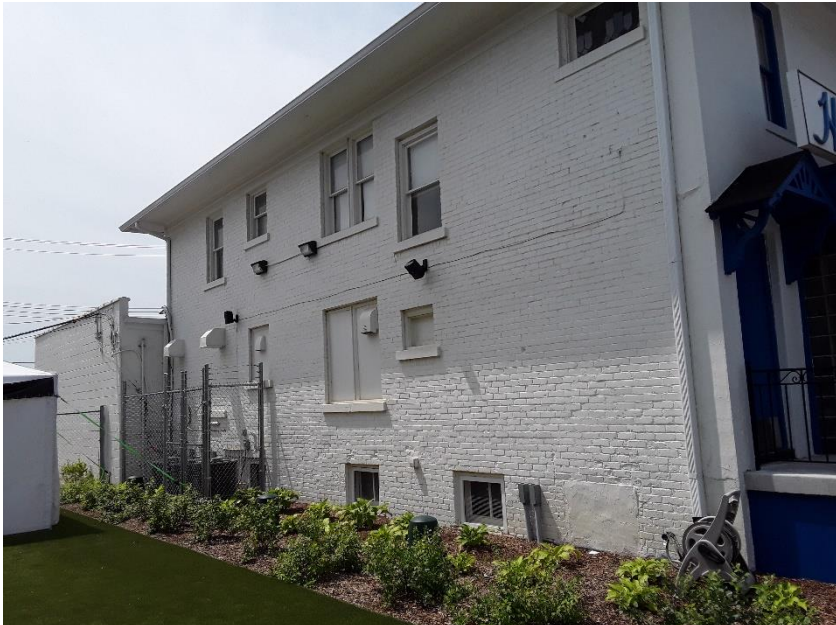
Western face of 2648 West Grand Boulevard
