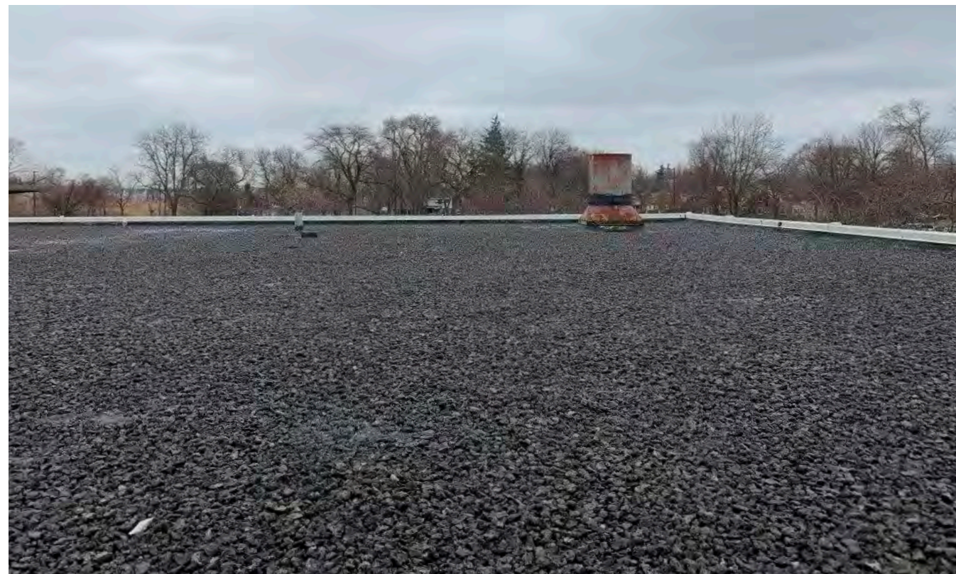
Photo R-07 / Overall view of High-Bay Roof looking North East
