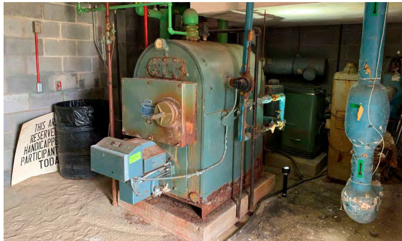
Photo M-01 / Overall view of Mechanical Room (112).
