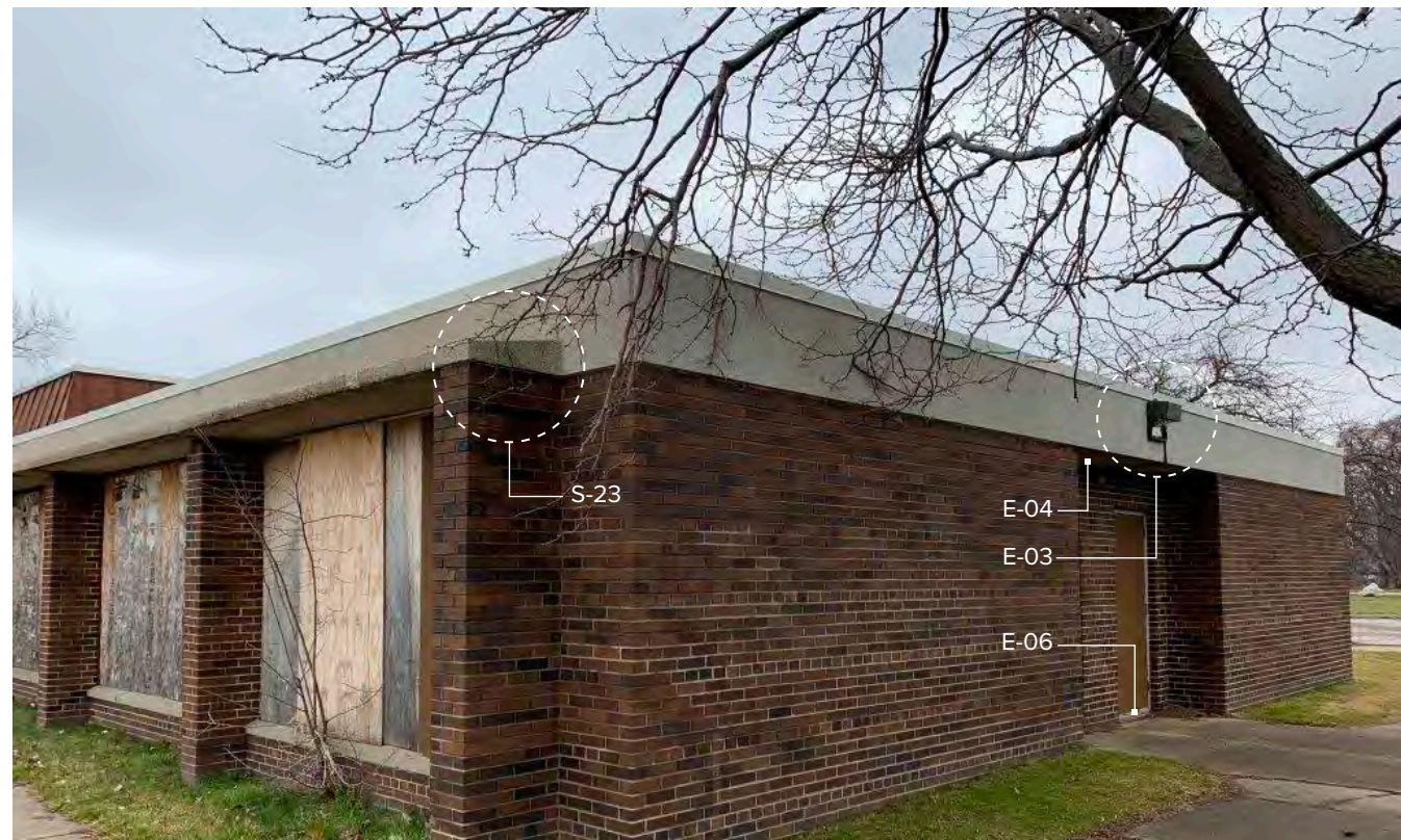
Photo E-01 / Overall view of East Elevation
