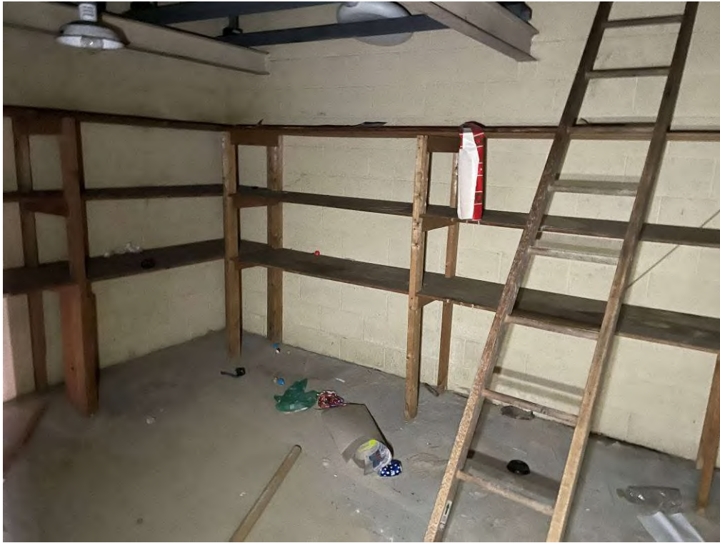
Photo 19: View of the eastern storage HVAC room.
