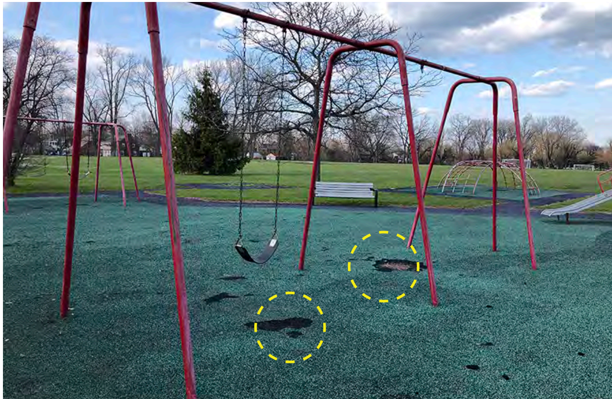
Photo ST-20 / View swing sets and worn safety surface at grade.
