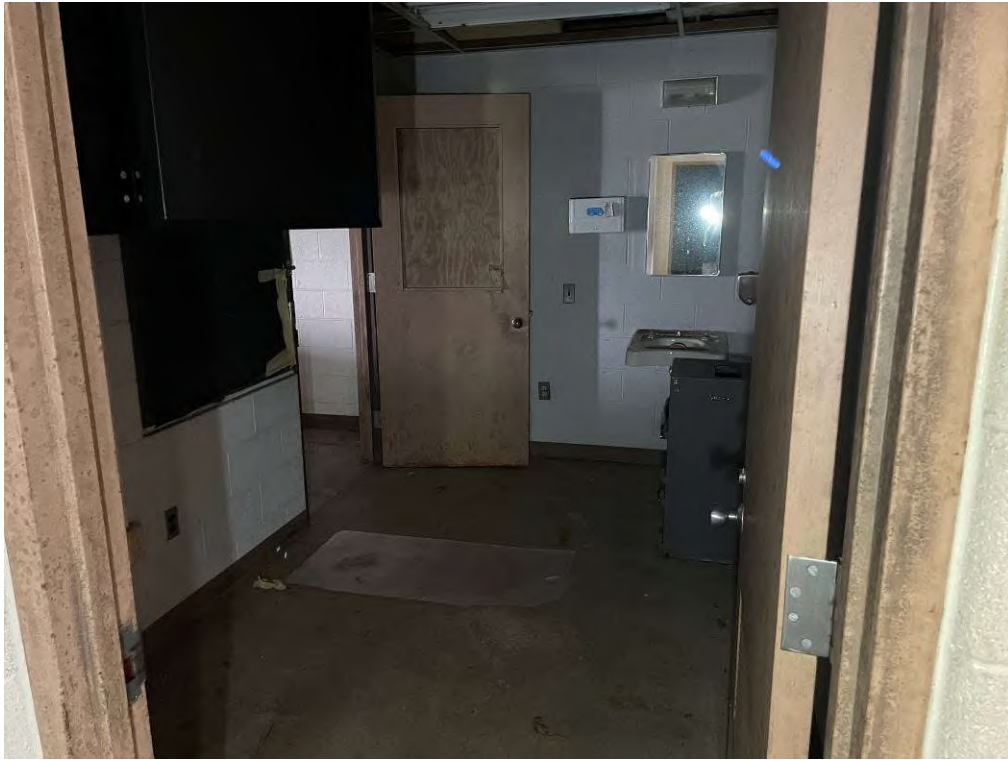
Photo 21: View of the first aid room.
