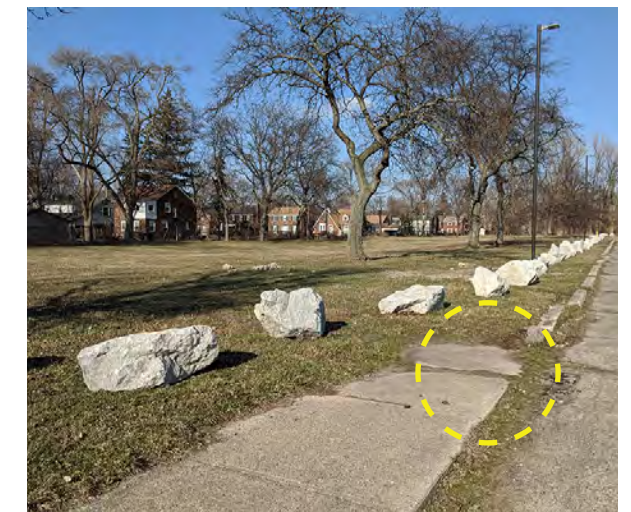
Photo ST-16 / Concrete walk adjacent to Main Parking Lot.
