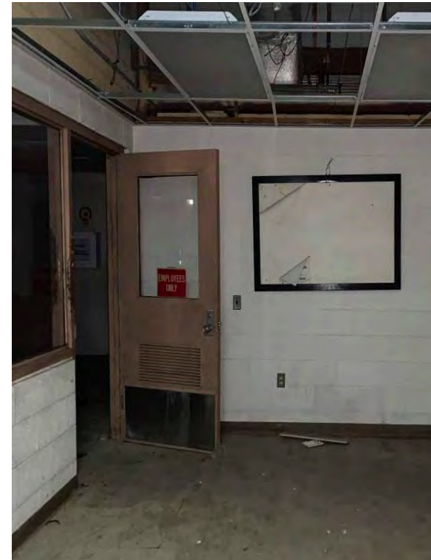
Photo I-26 / View looking west towards entry to Lounge (109) from Office (105)
