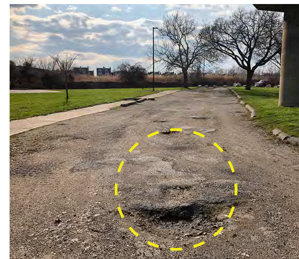
Photo ST-11 / View looking NW along Drop-Off Loop
