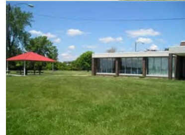
Picture above shows a picnic shelter on the south-west side of the building. The shelter is in fairly good condition.
