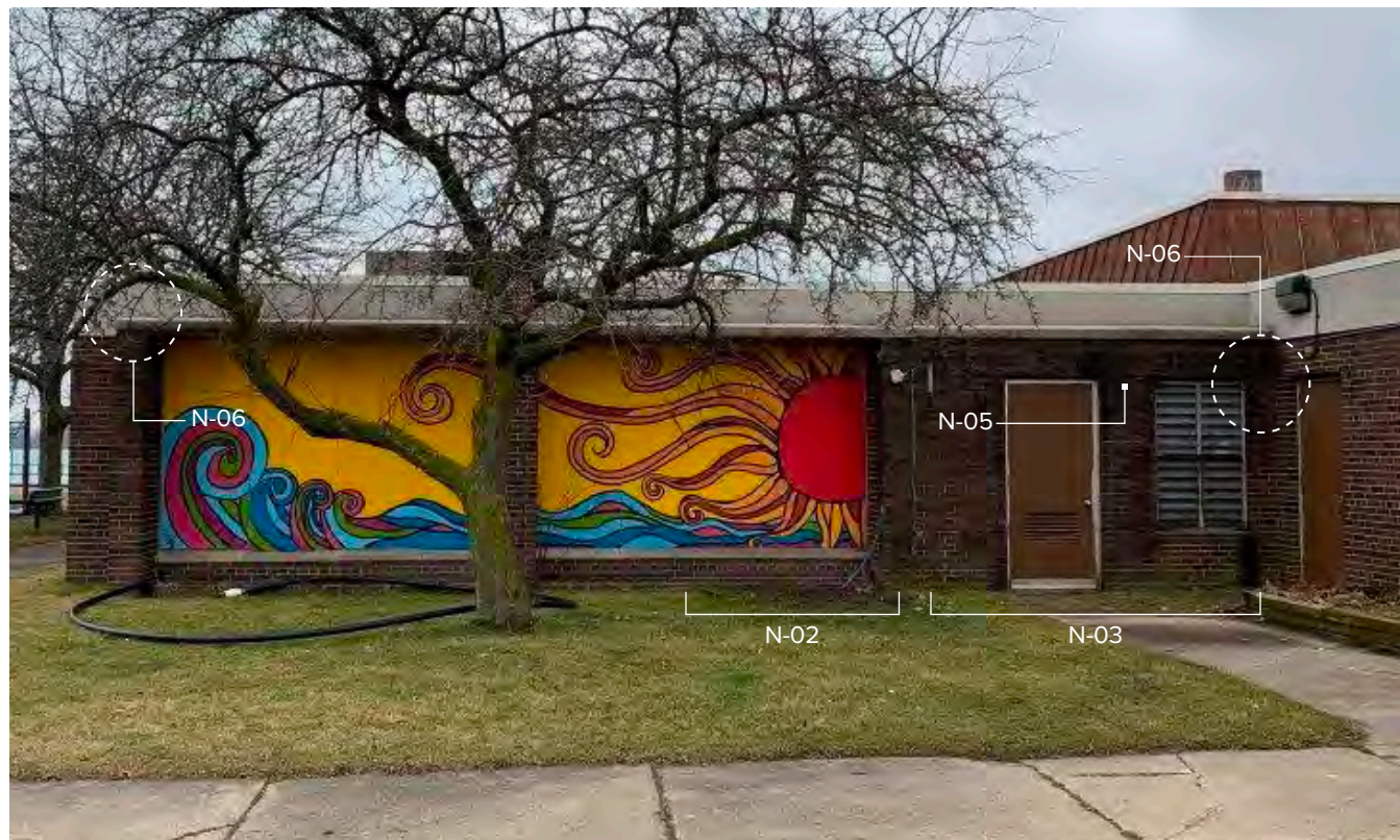
Photo N-01 / Overall view of North Elevation / East Wing
