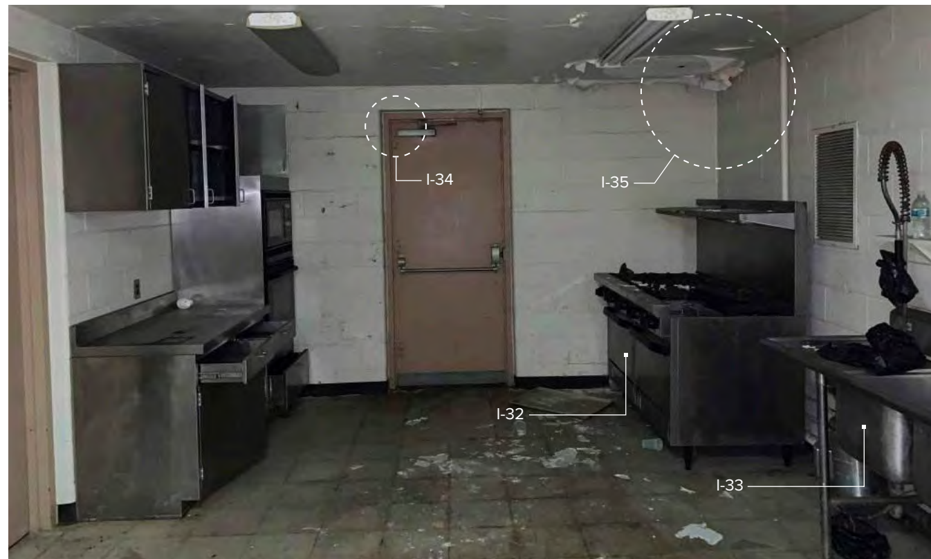
Photo I-31 / Overall view of Office (105) interior.
