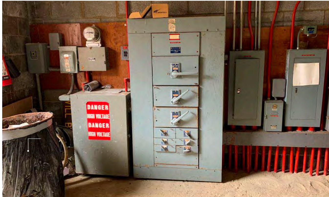
Photo E-01/ Partial view of South Elevation / East Wing
