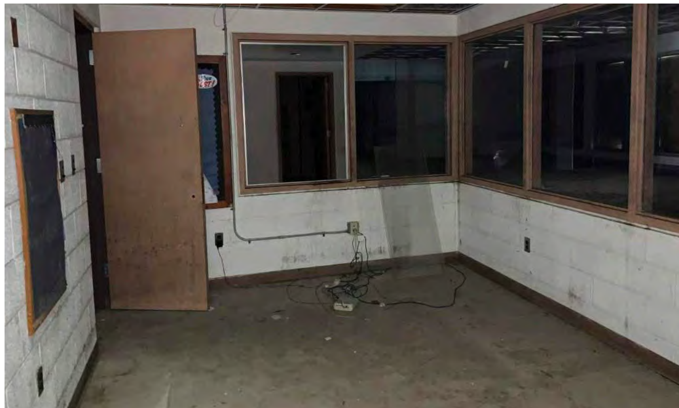
Photo I-25 / Overall view of Office (105) interior.
