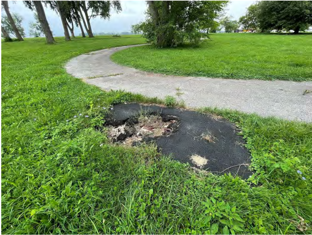
Photo 13: View of the walking path and former lighting structures pad located within the northeastern portion of the subject property.
