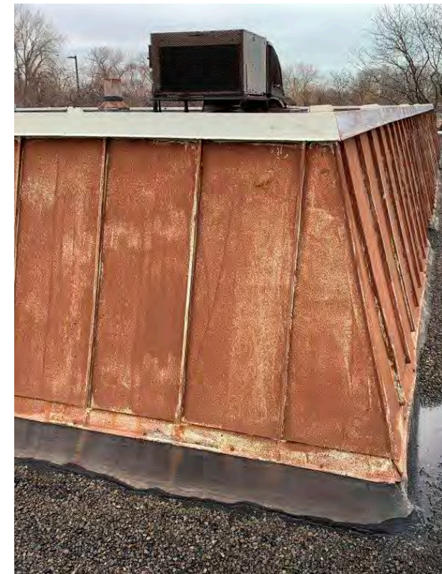
Photo R-08 / View of seamless terne standing-seam roofing at sloped wall of high-bay roof.
