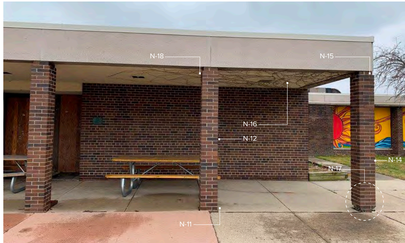
Photo N-13 / Partial view of North Elevation / Entry Wing (west)
