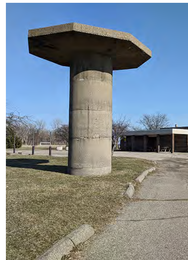
Photo ST-28 / Missile Tracking Radar (MTR) Tower
