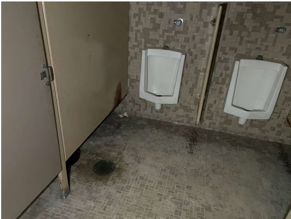
Photo 18: View of the eastern men's bathroom.
