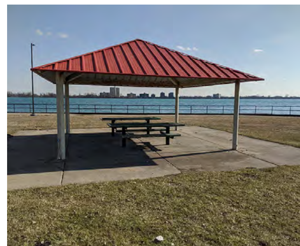
Photo ST-25 / Picnic Shelter
