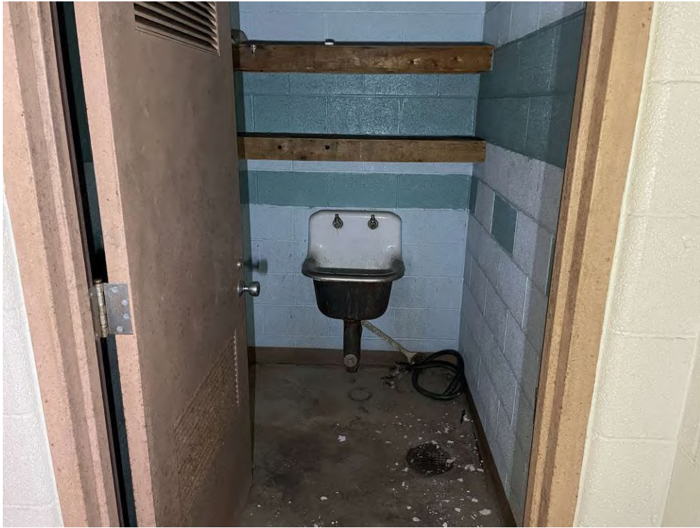
Photo 17: View of the eastern janitor's closet.
