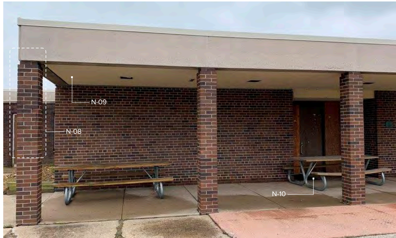
Photo N-07 / Partial view of North Elevation / Entry Wing (east)
