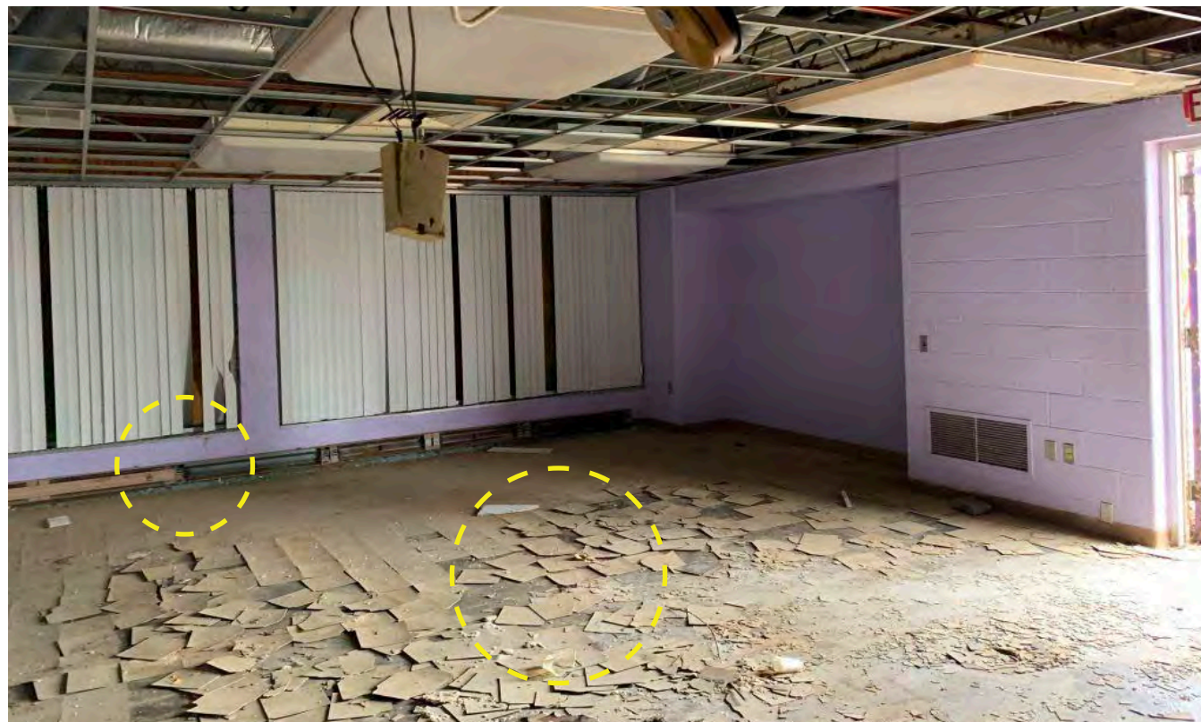
Photo I-62 / Overall view of Multi-Purpose (111) interior.
