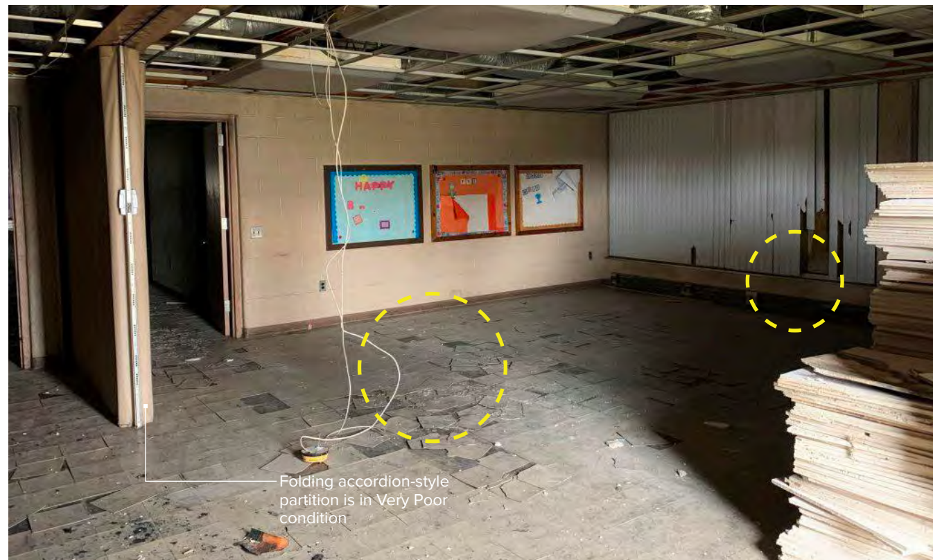
Photo I-37 / Overall view of Multi-Purpose (107) interior.
