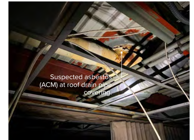
Photo 1-40 / View through ceiling grid of steel joist framing, metal roof deck and roof sump penetration.
