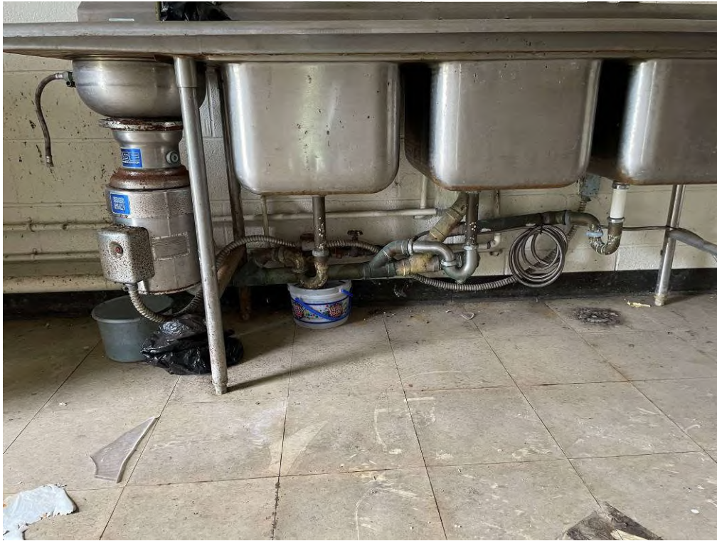
Photo 25: View of drains within the kitchen.
