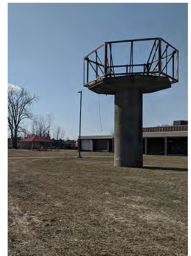
Photo ST-29 / Target Tracking Radar (TTR) Tower
