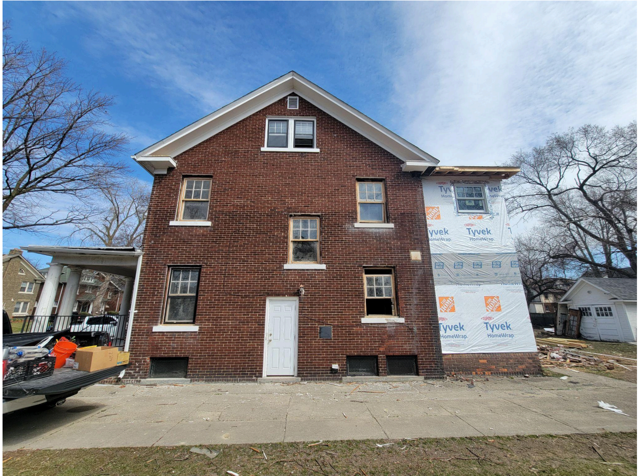
Side (west) facade
