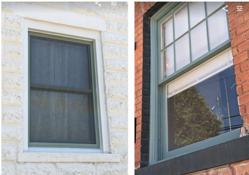
Left: Example of aluminum wrap covering brickmould, an unappropriated installation. Right: example of historically appropriate brickmould. Photos by staff. The type of installation proposed is not clear from application materials.
