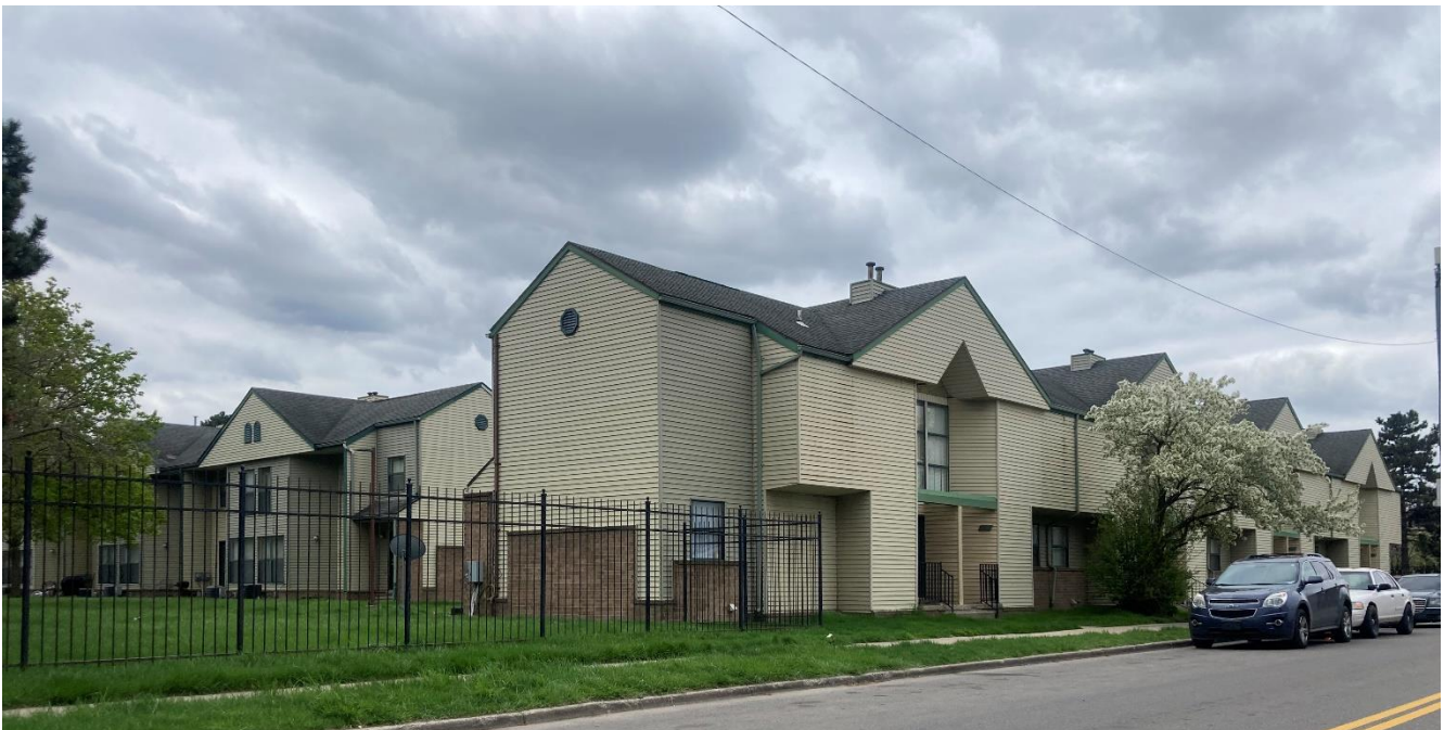
1601 Bagley, facing northwest. Staff photo taken on 4/22/2024
