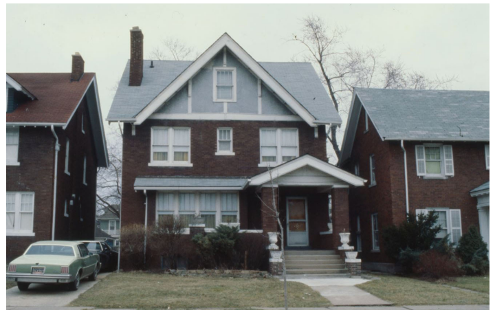
Image, 1980: (South) front elevation showing original windows and porch condition.
