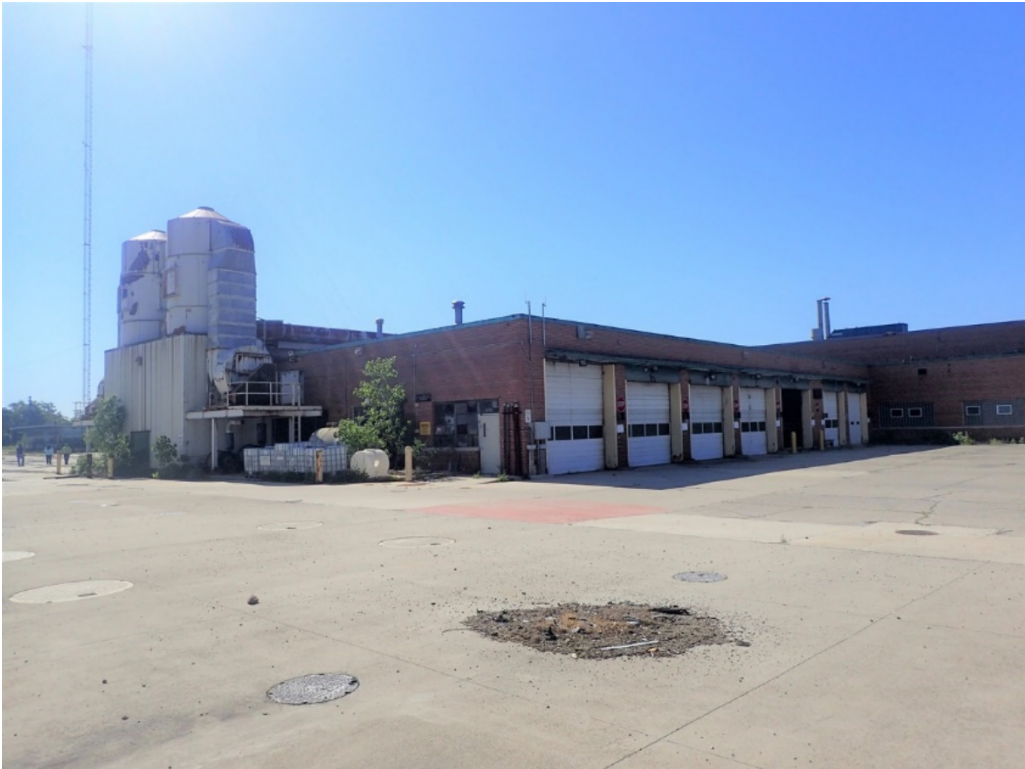
Figure 37. 14044 Schaefer Highway, Coolidge Terminal Building
