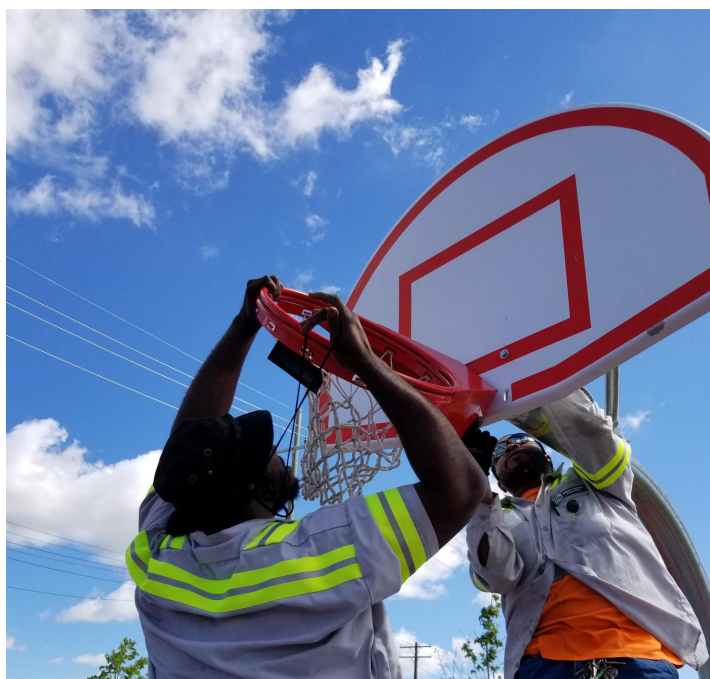
Park Development assembling a basketball hoop.
